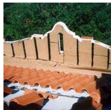
Projections on the underside of these replacement Spanish clay tiles help them adhere to the cement mortar on the roof sheathing. Photo: NPS files.
