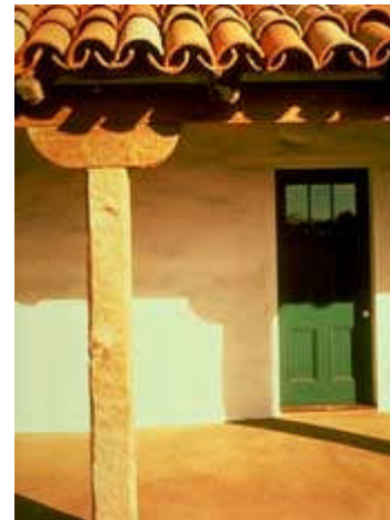
Tapered barrel clay roof tiles were custom made for the restoration of the 1820s Indian barracks at Mission Santa Cruz in California. Photo: NPS files.
