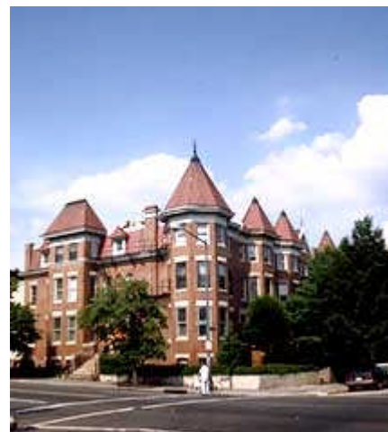
Clay tiles emphasize the prominence of the peaked roofs of these late 19th century rowhouses. Photo: NPS files.
