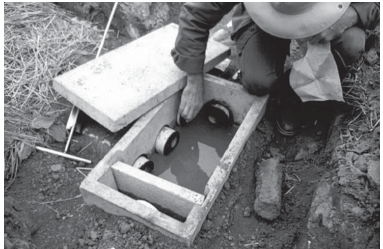
Figure 4-8. Distribution box with adjustable weir outlets
