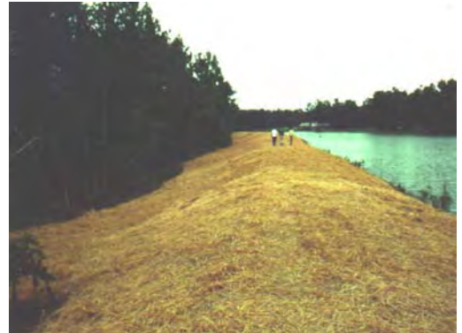
Figure 7. Completed remediation job after removing stumps, seeding, fertilizing & mulching.
