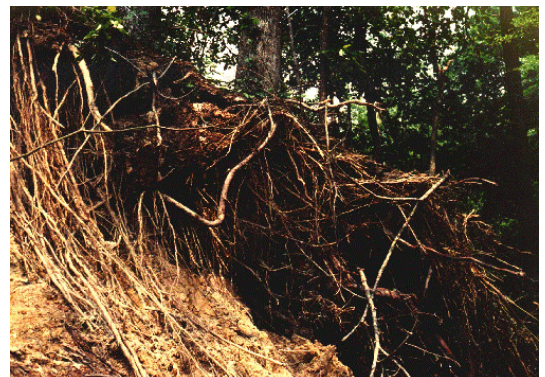
Figure 8. Exposed tree roots in overtopped dam.
