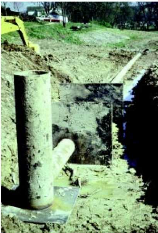
Figure 22 Drop-inlet pipe spillway with antiseep collar
