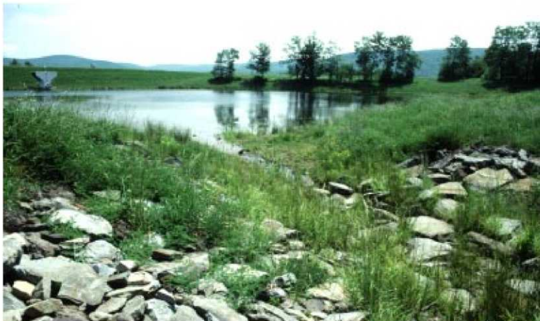
Figure 9 The shoreline of a well-designed pond is protected from erosion by the addition of stone. Such a pond, reflecting nearby trees, increases the value of the surrounding land
