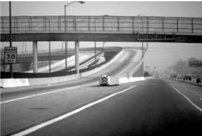
Figure 16. Grade separated HOV to highway flyover ramps
