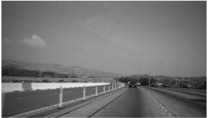
Figure 11. Tubular markers on SR 91
