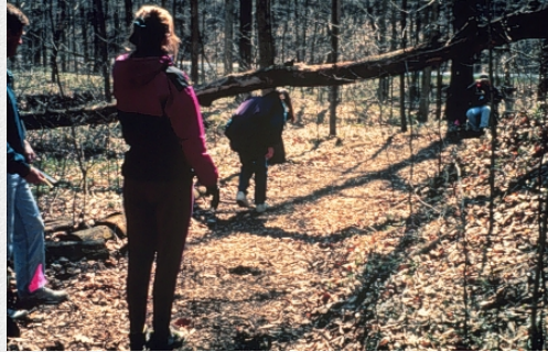
Figure 15-26. Objects, such as tree limbs, that protrude into the recreation trail tread more than 101 mm (4 in) should be removed.
