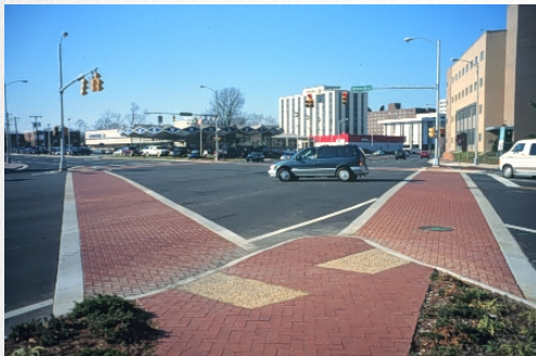
Figure 8-23. Skewed intersections create longer crossing distances, which significantly compromise pedestrian access.
