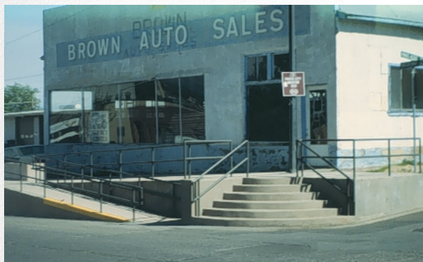
Figure 7-34. High curbs should be designed to provide access for both walking pedestrians and wheelchair users.
