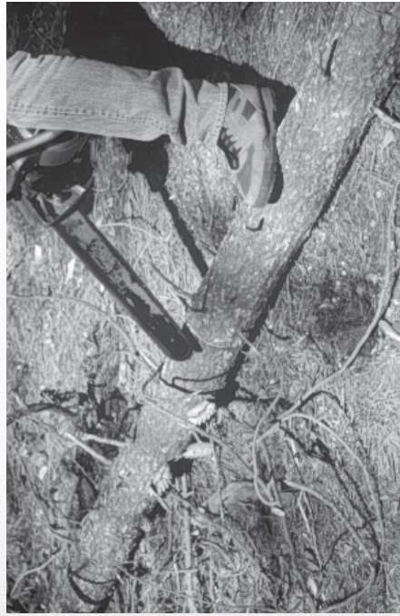
Figure 18-1. Obstacles, such as fallen trees, should be removed to maintain the tread in a condition that can be negotiated by all trail users.
