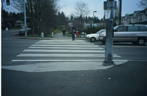
Figure 8-11. Continental crosswalks combined with alternative measures, such as pedestrian actuated traffic controls, enhance pedestrian crossing.
