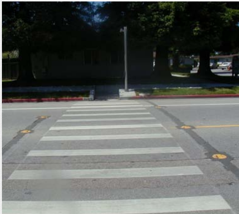
Figure 8-13. Imbedding lights in the asphalt at the edge of a crosswalk is an experimental method for making crosswalks more visible to motorists.
