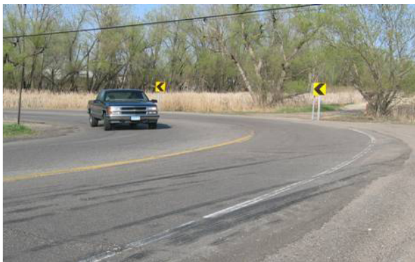
Widening on inside of curve.
