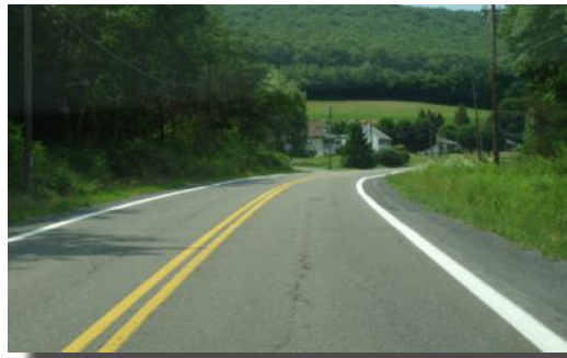
Roadway with 8-in edge line
