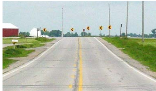
After installation of Chevrons.
