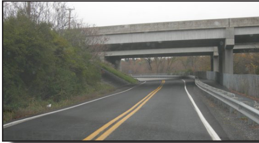
Centerline and edge line for two-lane road.
