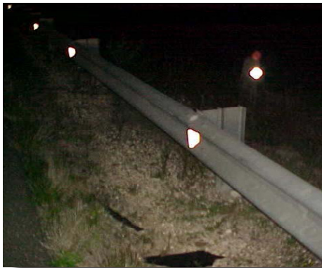
Installation of reflectors on W-beam guardrail.
