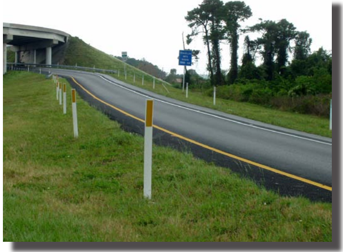
Post delineators installed on a ramp.
