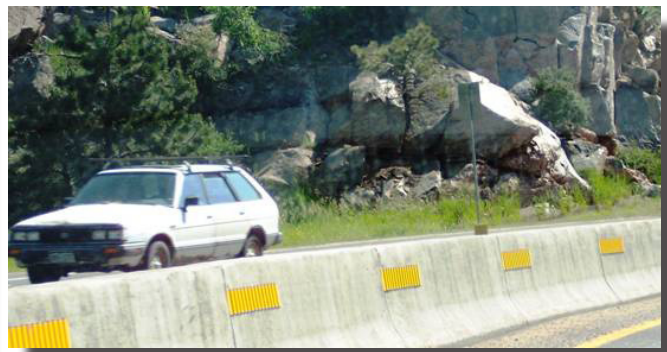
Reflective sheeting shaped to provide linear reflectorization.
