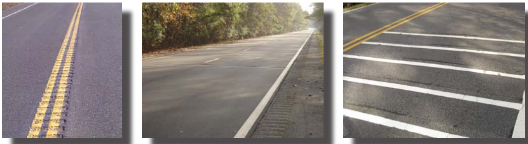
Illustrations of rumble strip for centerline (left), shoulder (middle), and across roadway (right).
