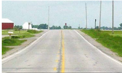
Before installation of Chevrons.
