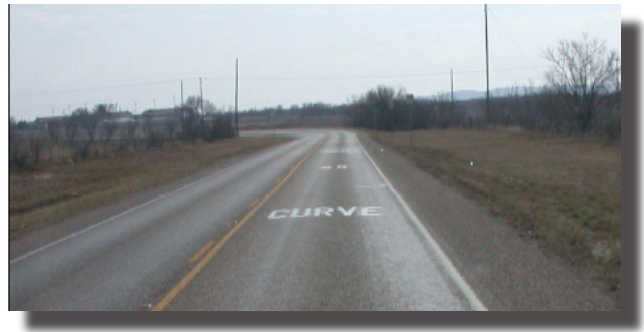
Speed-limit advisory pavement marking.
