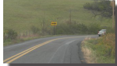
One direction Large Arrow Sign placed within curve.
