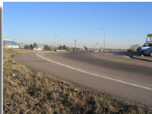
Widening on the outside of the curve.
