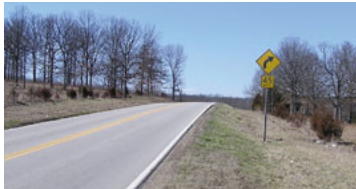
Photo source: Missouri DOT Curve Horizontal Alignment sign with an Advisory Speed Plaque warns the driver of an approaching curve over the crest of a hill.
