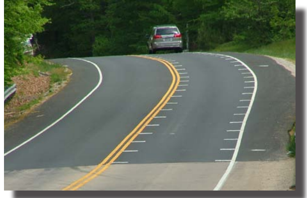
Photo: Courtesy of Virginia Department of Transportation Optical Speed Bars used to reduce vehicle speed.
