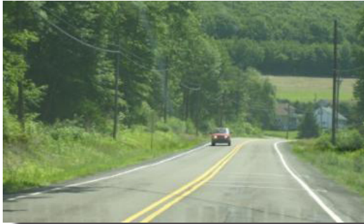
Roadway with 4-in edge line
