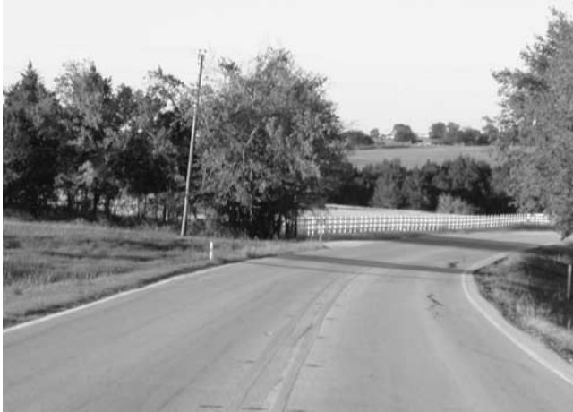
Figure D-1. Case Study A roadway.
