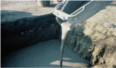
Figure 5-1. Flowable fill used in a utility trench application
