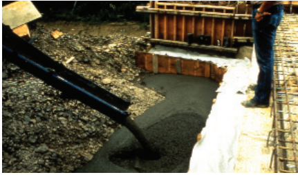
Figure 5-4. Bridge abutment backfill with flowable fill.
