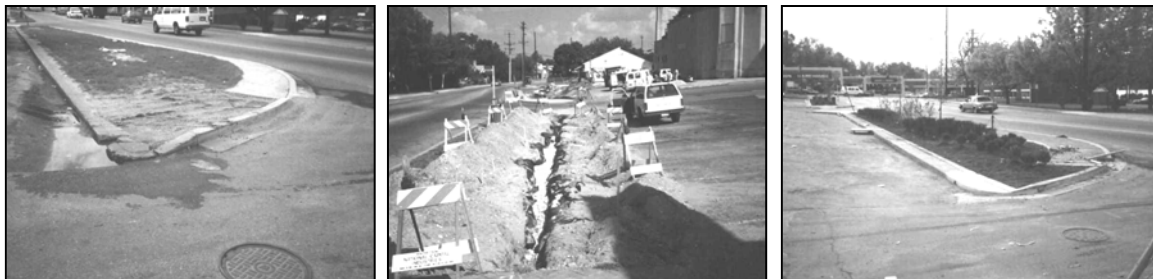
Fig 4.7: Same island- before, during and after construction
