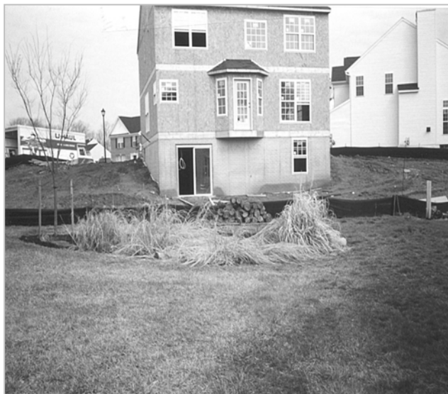
Fig. 4.1: Silt fence around bioretention
