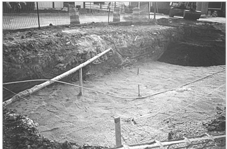
Fig. 4.6: Natural compaction and settlement is recommended
