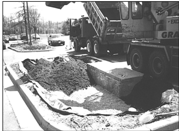
Fig. 4.5: Installation of filter fabric and soil medium
