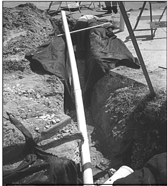
Fig. 4.2: Installation of underdrain
