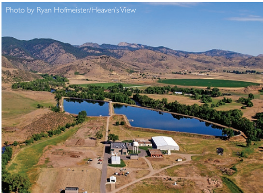
Effective utility management is applicable to all utilities, regardless of size or circumstance
