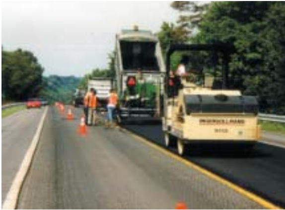
Figure 17. Construction of HMA pavement
