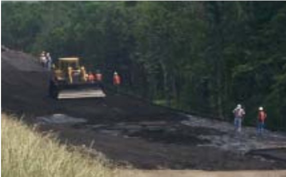
Figure 10. Spreading foundry sand (Ohio turnpike, sand supplied by Kurtz Bros. Inc.)
