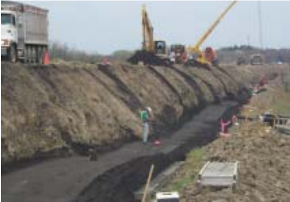
Figure 7. Embankment with foundry sand subbase (Ohio Turnpike, sand from Ford Motor Company supplied by Kurtz Bros. Inc.)
