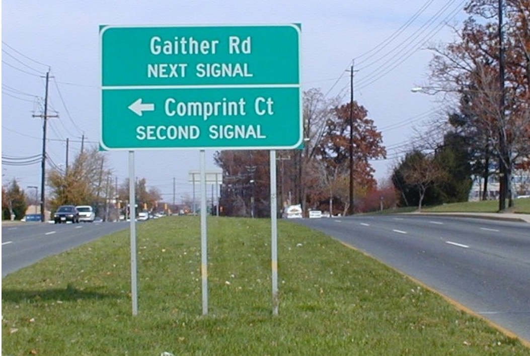
Figure 39. Example of advance street name sign for two closely spaced intersections.
