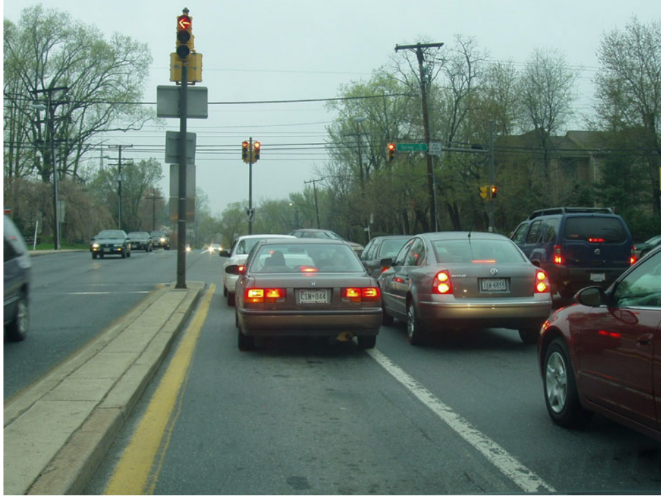
Figure 117. Narrow (2.4-m (8-ft)) left-turn lanes may be used effectively in retrofit situations.
