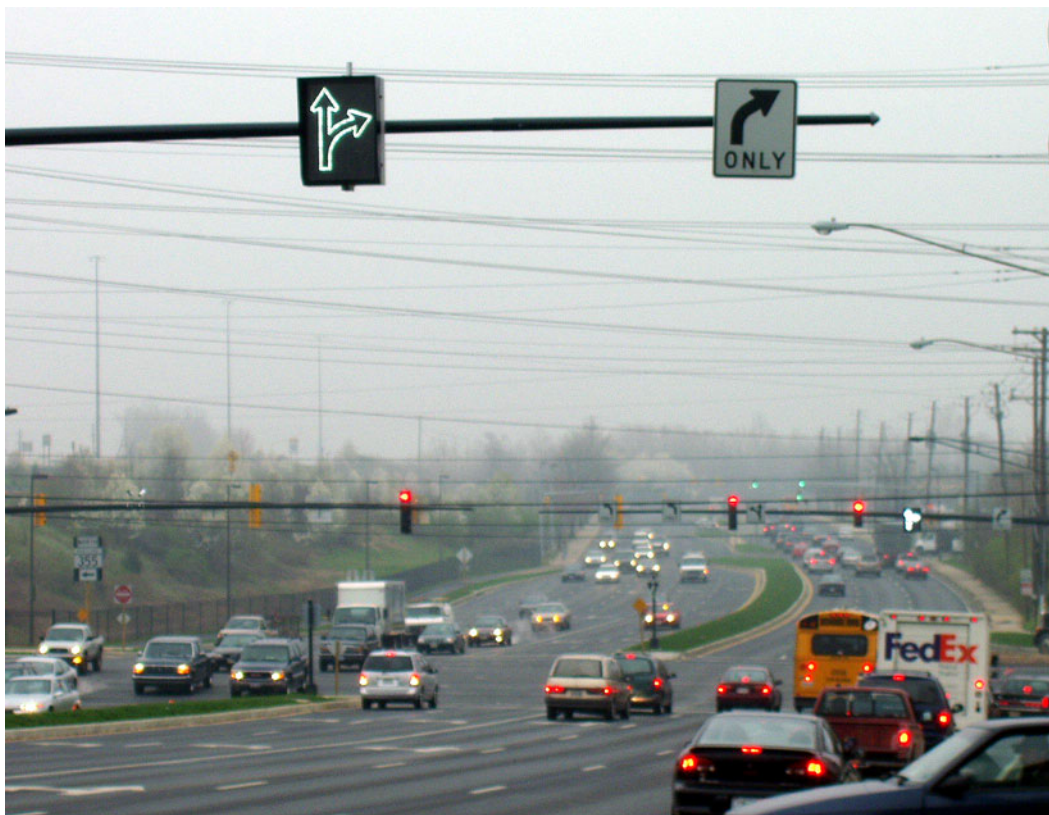
Figure 126. Example use of variable lane use sign to add a second right-turn lane along a corridor during certain times of day.
