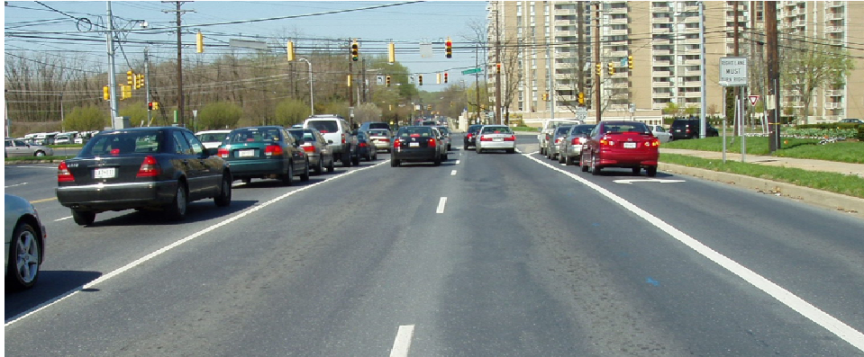
Figure 123. Narrow (2.4-m (8-ft)) right-turn lanes may be used effectively in retrofit situations.
