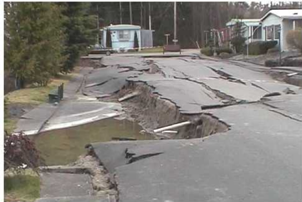
h) Collapsing soils, karst conditions, or liquefaction
