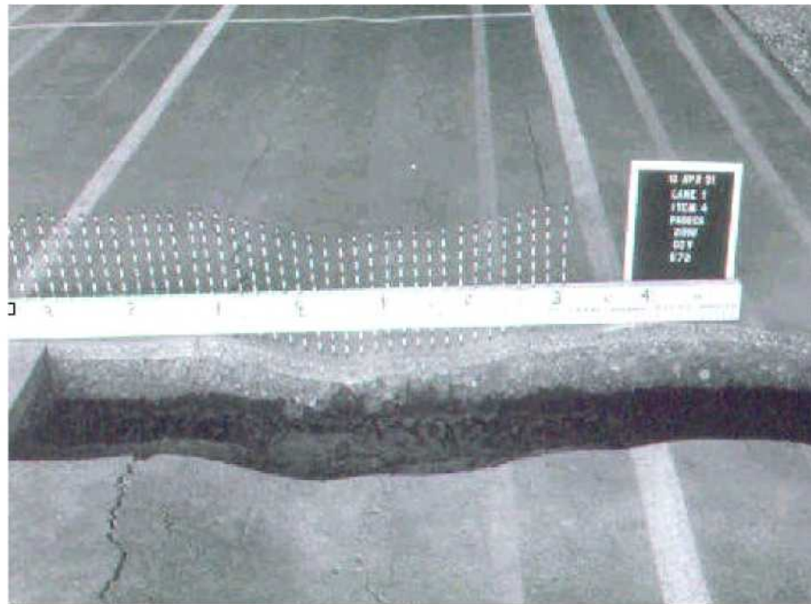
Figure 1-6. Normal rutting.
