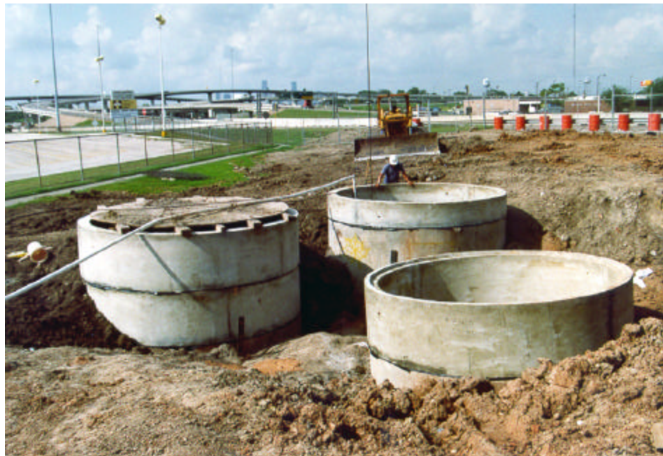
Figure 3-14. Circular caisson wet wells under construction.
