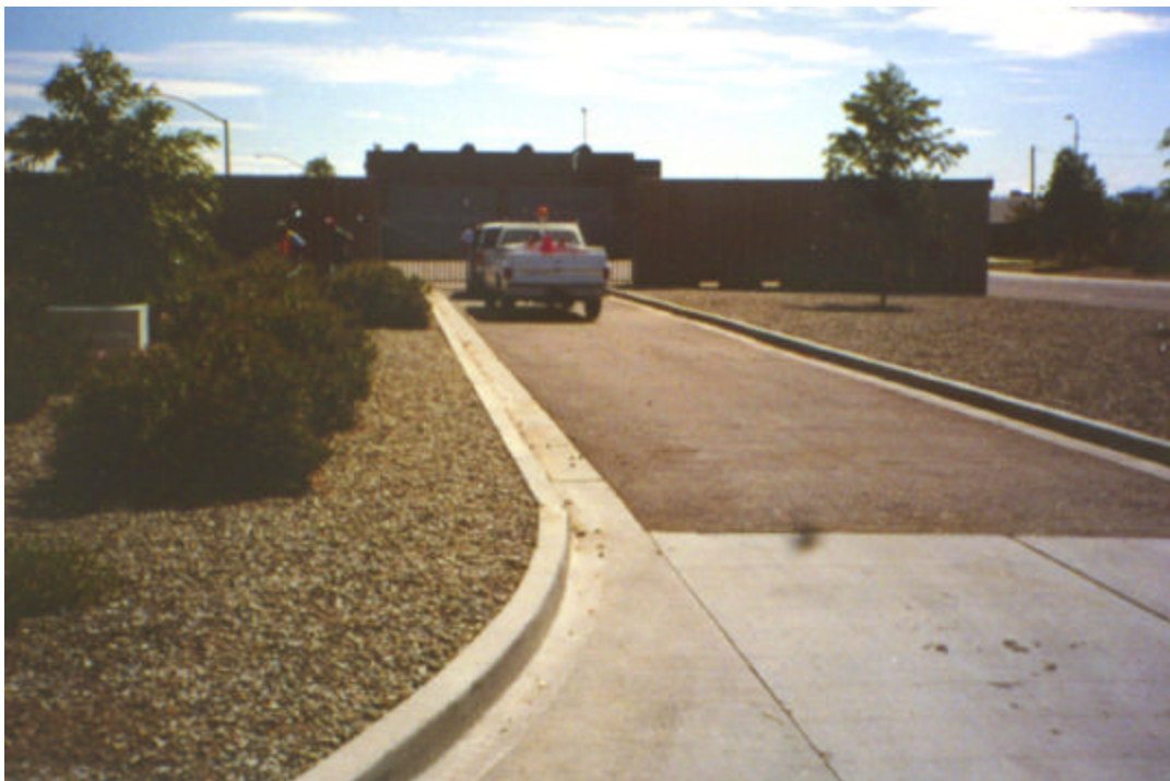
Figure 5-4. Driveway access to pump station in Arizona
