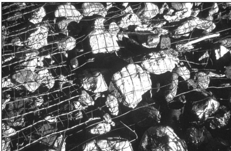
Figure 1.5. Wire-Enclosed Riprap
