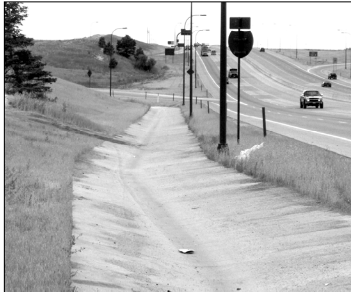
Figure 1.1. Rigid Concrete Channel Lining
