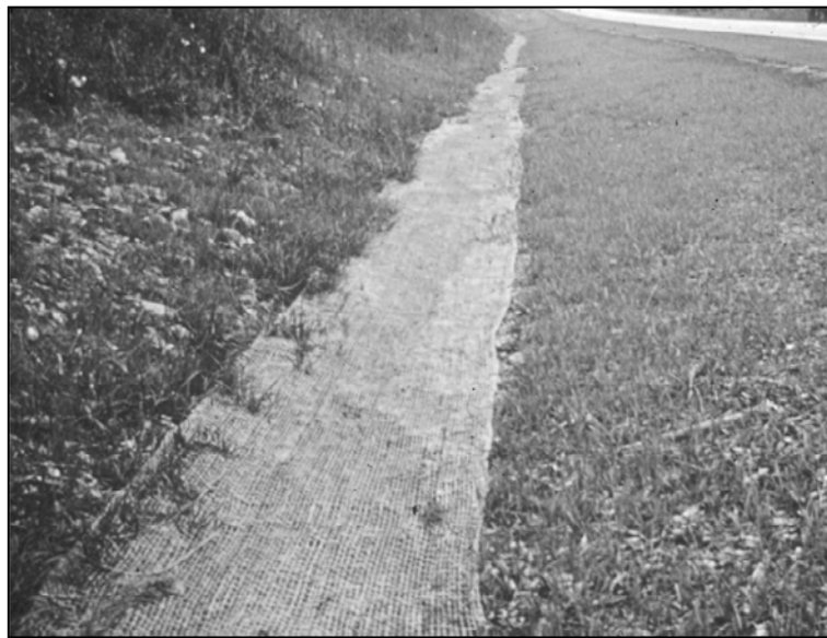
Figure 1.10. Installed Open Weave Textile Channel Lining
