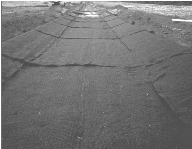
Figure 1.8. Installed TRM Lining Before Vegetation (Source: ECTC)
