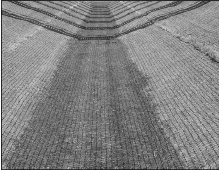
Figure 1.11. Erosion Control Blanket (ECB) Lining (Source: ECTC)
