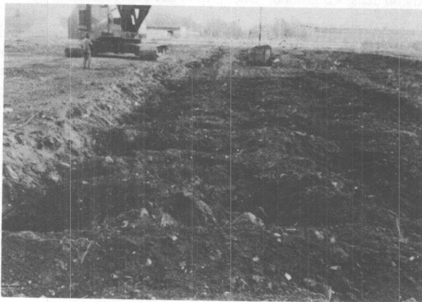
Figure 2. Typical dynamic compaction grid pattern with 13.6 Mg tamper in background.
