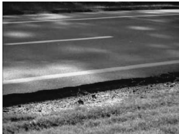
EXHIBIT V-9 Example of Edge Dropoff (ROR guide)
