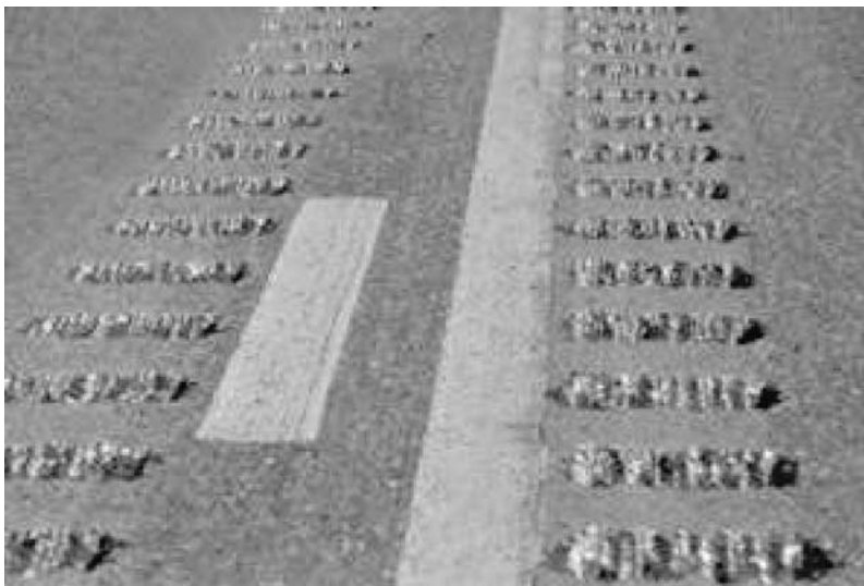
EXHIBIT V-7 Centerline Rumble Strips (Photo Provided by MnDOT)
