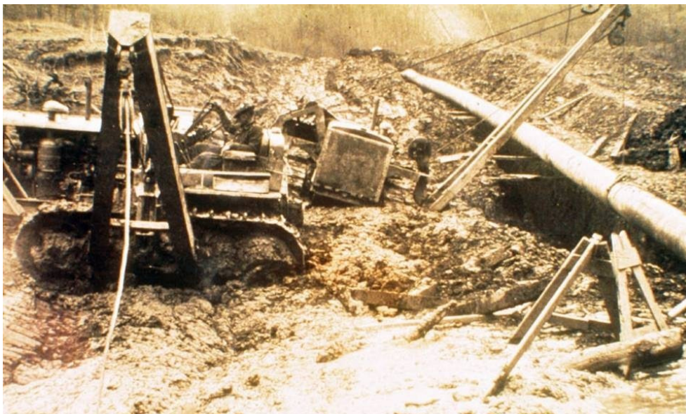
Figure 1: Pipeline Construction Near a Waterbody in the Mid-1900's
