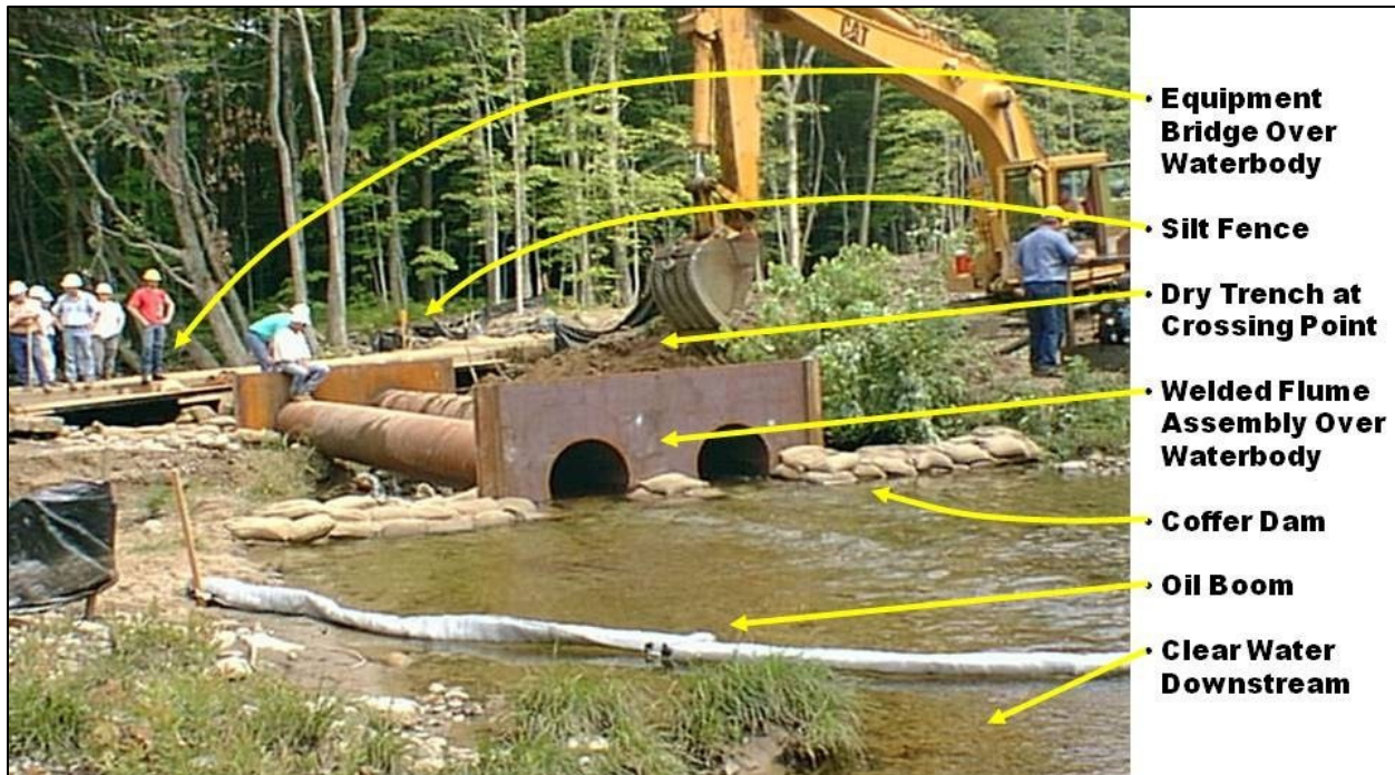
Figure 2: “Dry” Waterbody Pipeline Construction in Maine, 1999
