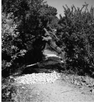
Constructing an underdrain from large rocks, with geotextile serving as a separator between surface material and large rocks.
