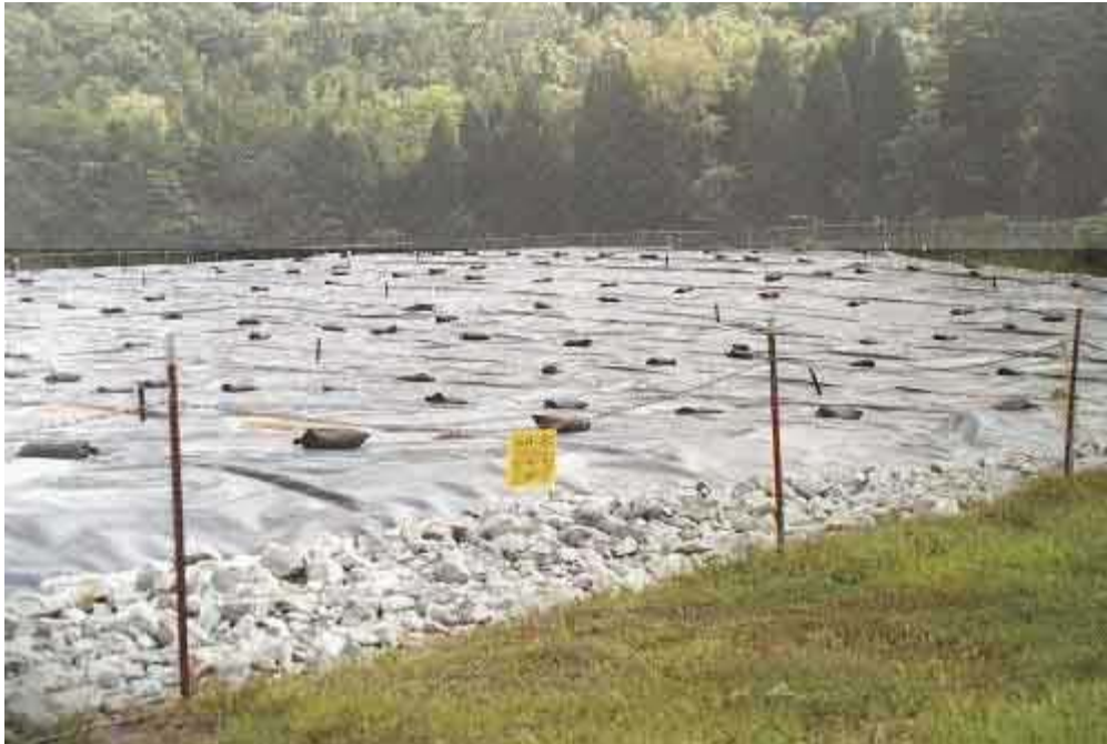
Figure 14: Example of a synthetic membrane used as a single barrier cap, Oak Ridge, Tennessee
