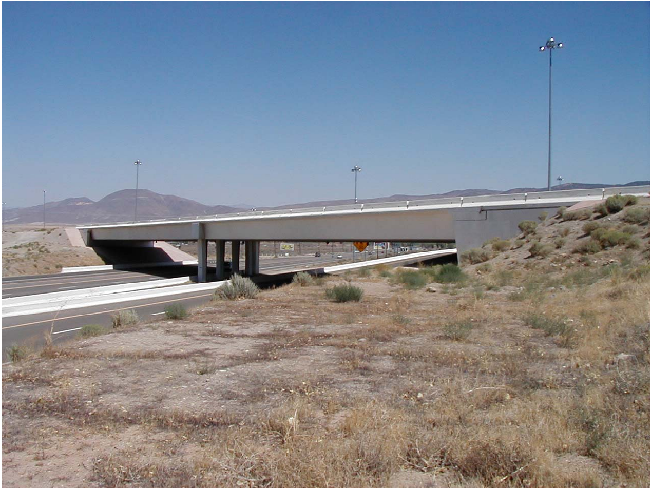
Figure 2-12: Mt. Rose Interchange: I-580 Overcrossing at Mt. Rose Highway, Nevada
