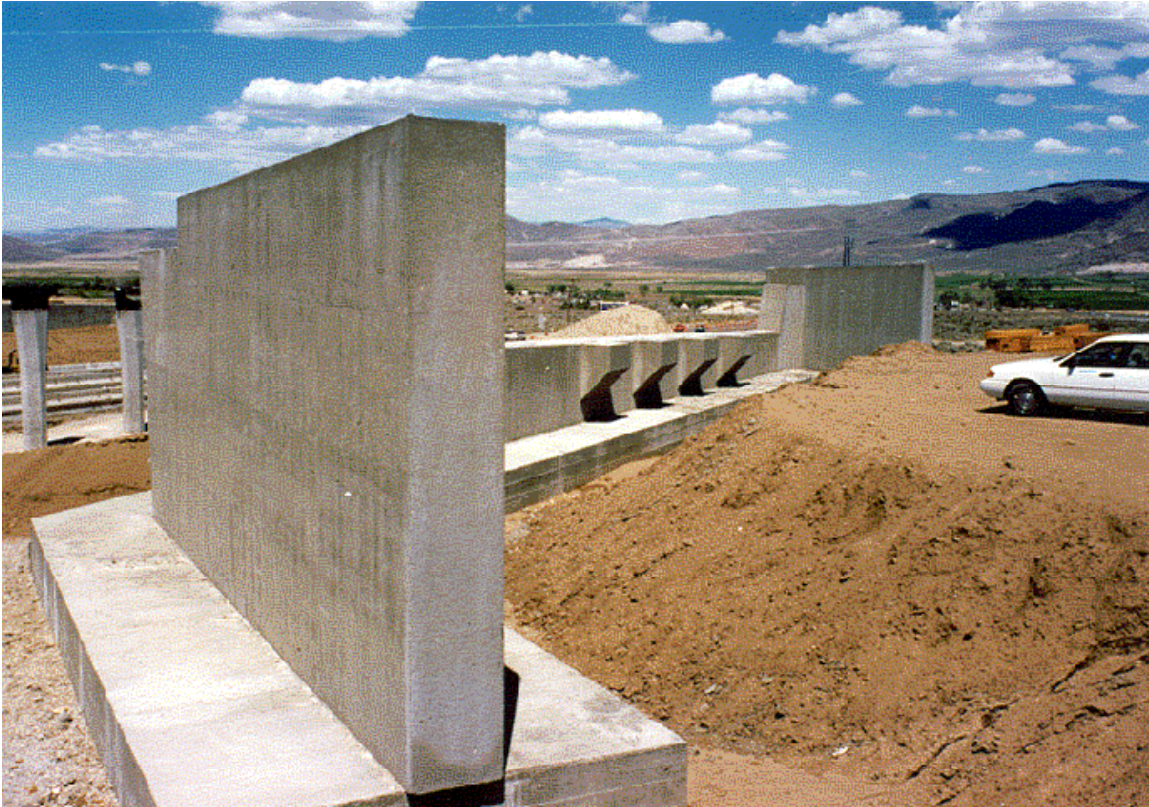
Figure 2-14: Footing at South Abutment, I-580, Nevada
