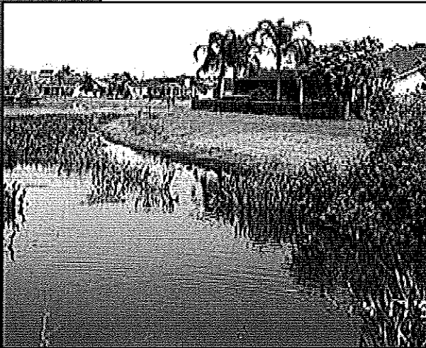
▲ Planted littoral zone in residential stormwater pond.
