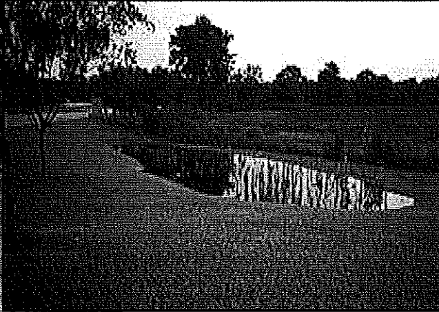
Pretreatment Sediment Basin ▲
