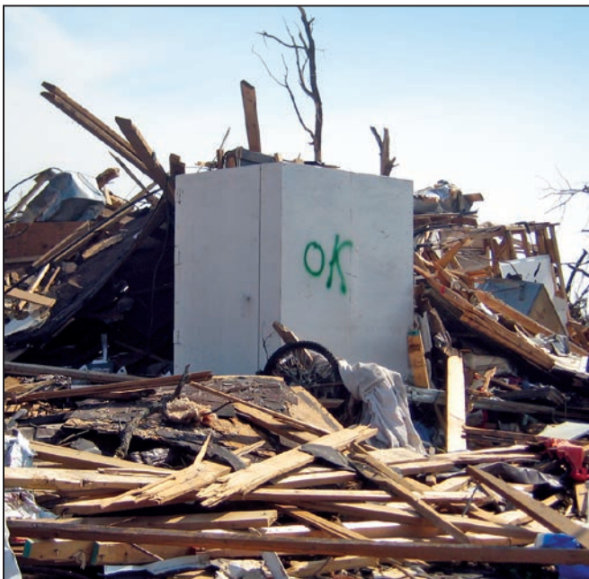
Figure 3-5: Above-ground residential safe room that was in the garage of a home hit by an EF5 tornado in Joplin, MO (2011)
