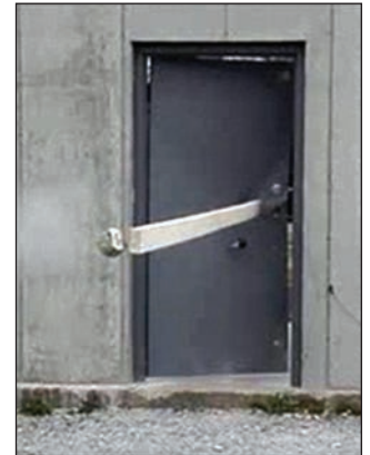
Tornado safe room impact test results: Door assembly failed at latch/lock
