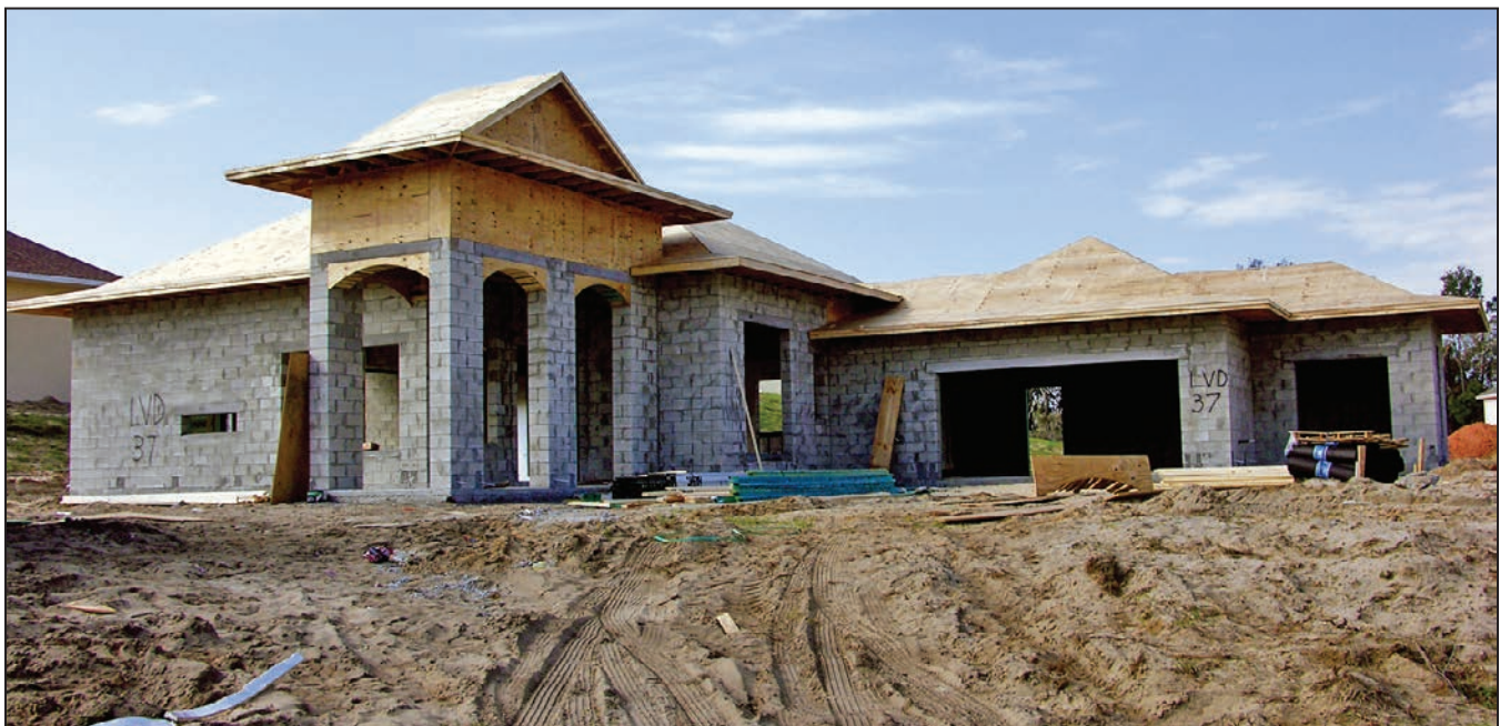
Figure 3-1: Exterior walls constructed of CMUs (New Smyrna Beach, FL, 2007)
