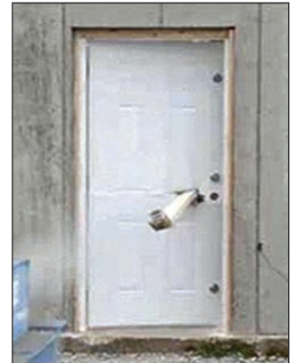
Tornado safe room impact test results: Door assembly failed when perforated
