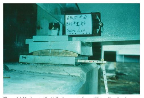
Figure 9.1.28 Longitudinal Misalignment in Bronze Sliding Plate Bearing
