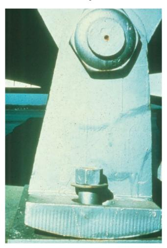
Figure 9.1.12 Pinned Rocker Bearing
