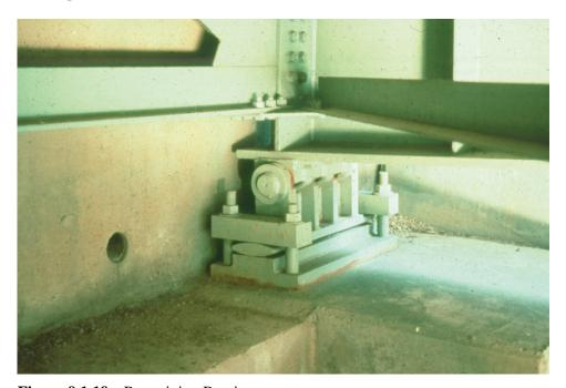
Figure 9.1.19 Restraining Bearing
