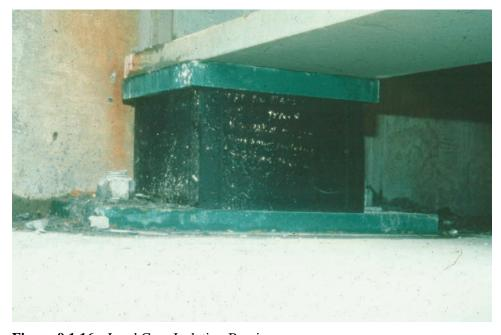
Figure 9.1.16 Lead Core Isolation Bearing
