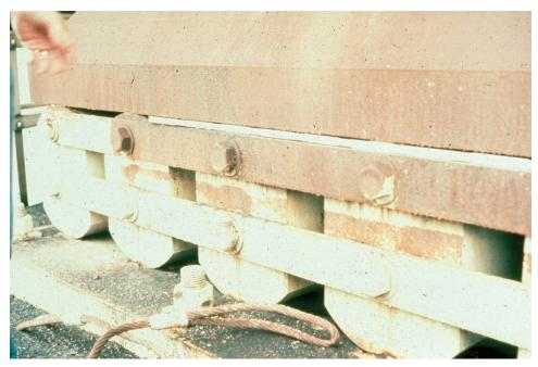
Figure 9.1.11 Segmental Rocker Nest Bearing
