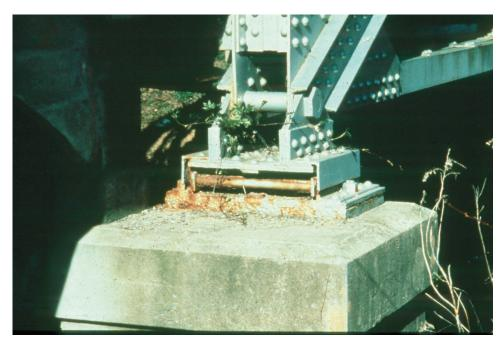
Figure 9.1.8 Roller Nest Bearing
