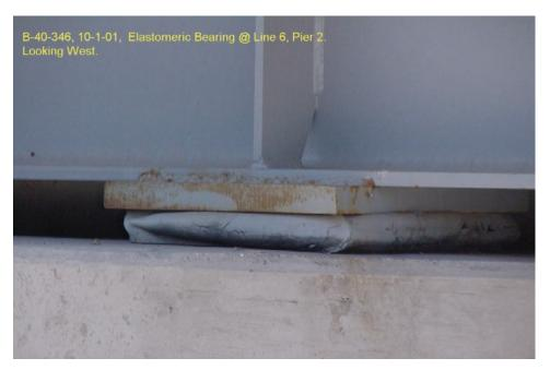
Figure 9.1.35 Neoprene Bearing Pad Excessive Bulging
