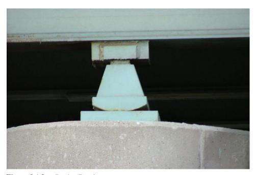
Figure 9.1.9 Rocker Bearing
