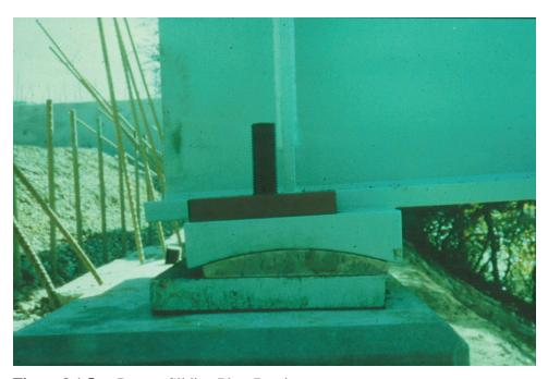
**Figure 9.1.5** Bronze Sliding Plate Bearing
