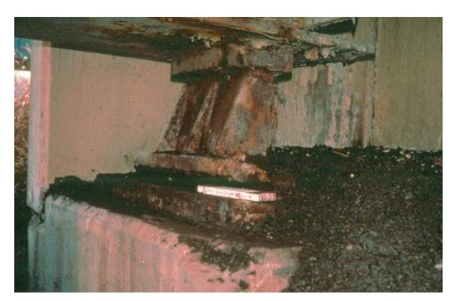
**Figure 9.1.22** Heavy Corrosion and Excessive Movement on Steel Rocker Bearing
