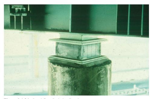
Figure 9.1.36 Lead Core Isolation Bearing
