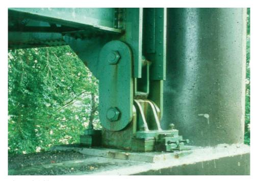
Figure 9.1.20 Pin and Link Bearing
