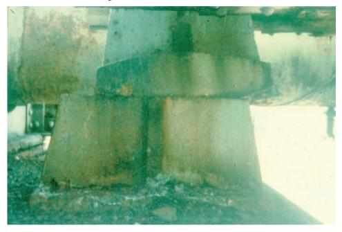
Figure 9.1.23 Rocker Bearing with Excessive Horizontal Movement
