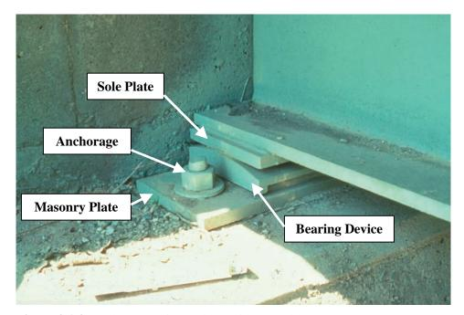
Figure 9.1.3 Elements of a Typical Bridge Bearing
