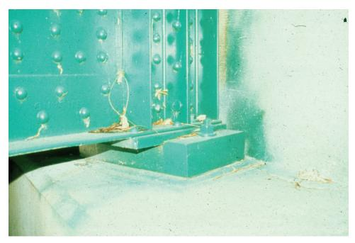
Figure 9.1.4 Lubricated Steel Plate Bearing
