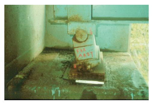
Figure 9.1.38 Broken Pintle on a Bearing
