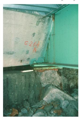
Figure 9.1.24 Spalling of Concrete Bridge Seat Due to High Edge Stress
