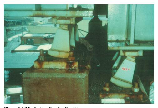
Figure 9.1.37 Serious Bearing Condition
