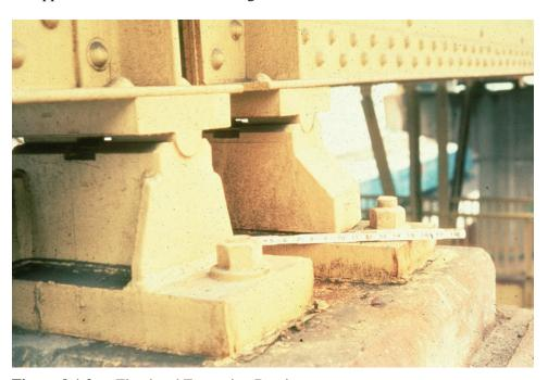
Figure 9.1.2 Fixed and Expansion Bearings
