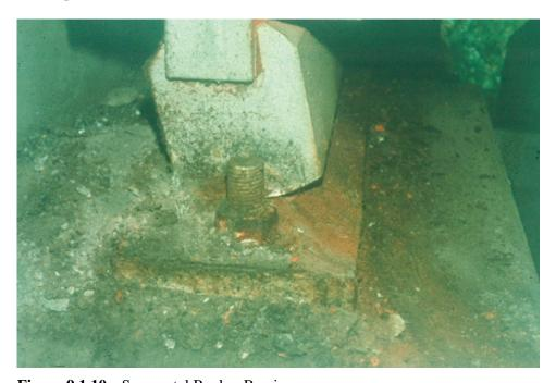
Figure 9.1.10 Segmental Rocker Bearing
