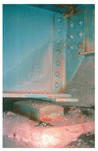
Figure 9.1.26 Uplift at Bridge Bearing
