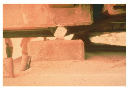
Figure 9.1.31 Excessive Tilt in a Segmental Rocker
