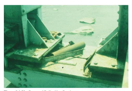
Figure 9.1.29 Damaged Roller Nest Bearing
