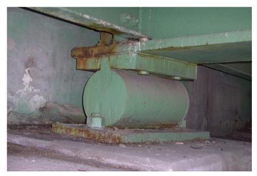
Figure 9.1.7 Single Roller Bearing
