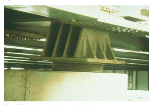
Figure 9.1.14 Laminated Neoprene Bearing Pad
