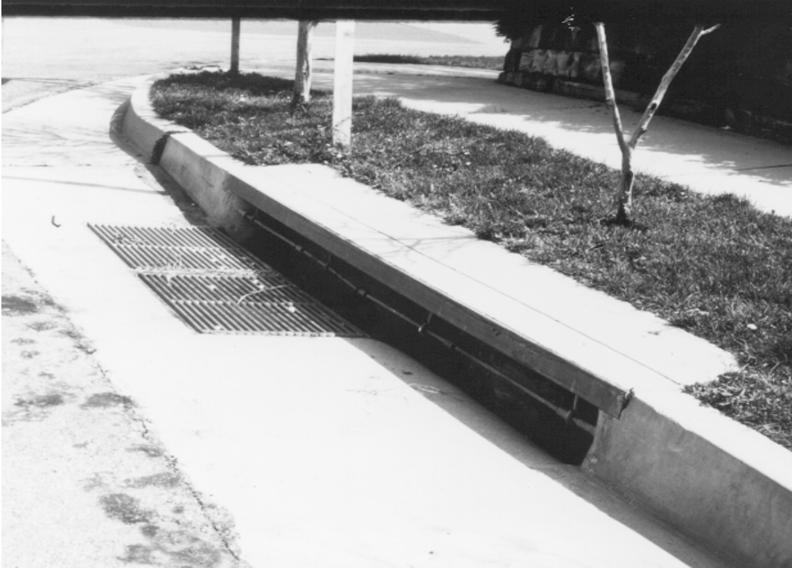
Figure 4-16. Sweeper combination inlet.
