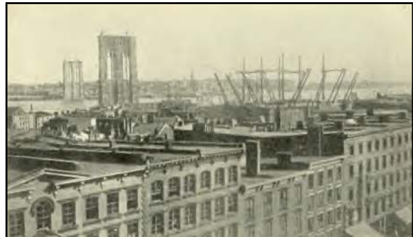
NY Tower and Anchorage (looking towards Brooklyn)
