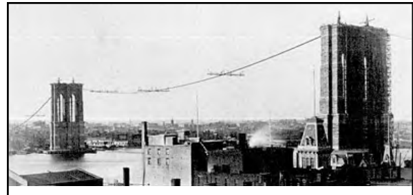
Main/River-span footbridge and access cradles (cradles at quarter points)
