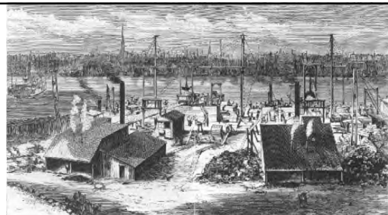
Atop the Brooklyn Caisson
