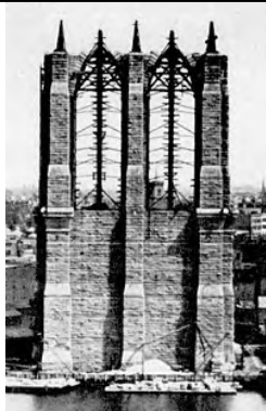
Wooden "falsework" in-place (for forming the Gothic Arches, Brooklyn Tower)
