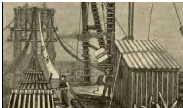
Eye-Bar Chain (connecting to cable strands)
