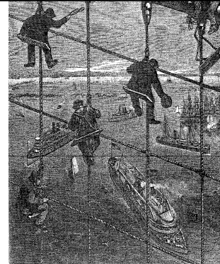
JAR's trademark cable stays (being tied to the suspenders cables)
