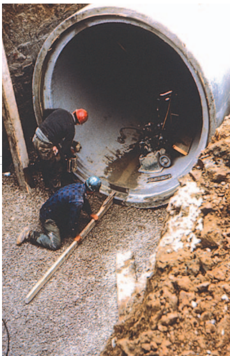
Workers install sewer line
