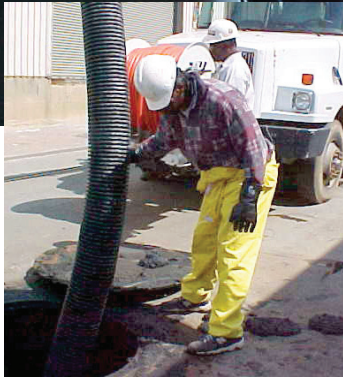
Sewer line maintenance
