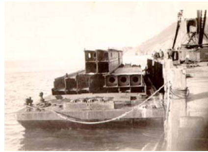
Barge with Steel Sections (adjoining pier)
