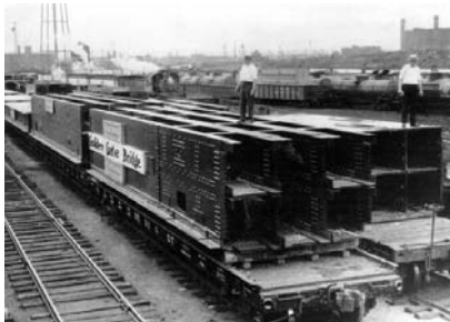
Tower Steel Sections (being transported by rail to Philadelphia)
