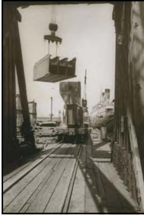
Off-Loading Tower Sections (San Francisco)
