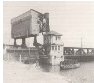
Fourth Street Bridge San Francisco, CA (1916)
