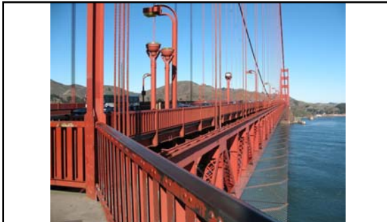
After years of debate and controversy (i.e. cost, aesthetics), in 2010 GGB officials approved construction of a Suicide Barrier . In the rendering above, a continuous net runs twenty-feet below the pedestrian walkway. 631
