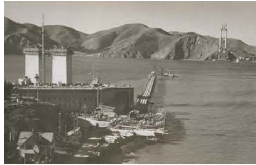
Access Trestle Complete
