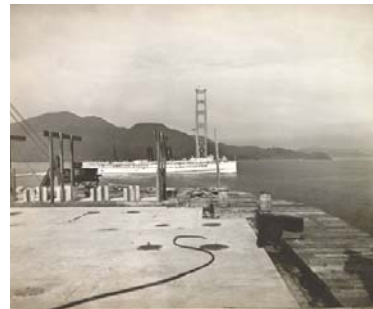
Atop the completed pier
