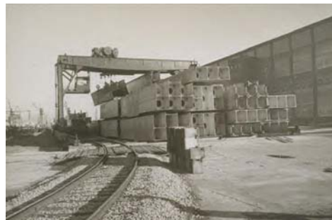
Loading Tower Sections (onto rail cars at foundry)
