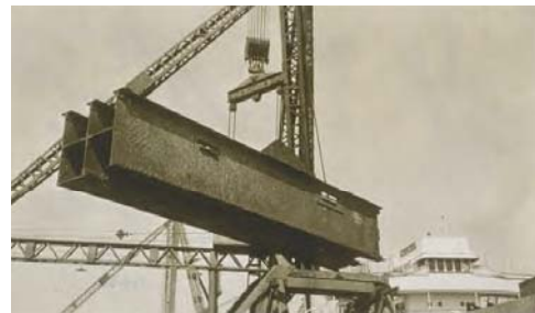
Tower Steel Sections (being loaded onto freighter)
