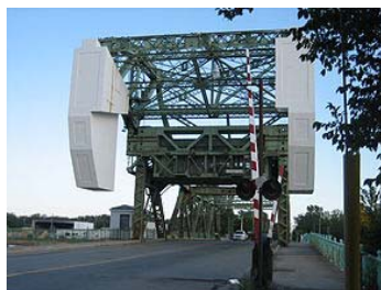
Cherry Street Strauss Trunnion Bascule Bridge Toronto, Ontario, Canada (1931)
