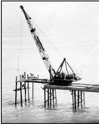
Rebuilding the access trestle after the storm (with timber piles)
