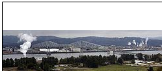
Lewis and Clark Bridge Over the Columbia River - between Longview, WA and Rainier, OR (1930)
