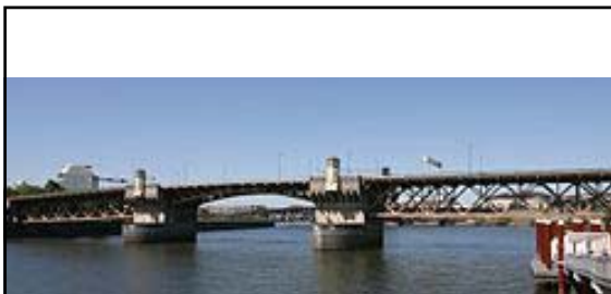
Burnside Bridge Portland, Oregon (1926)
