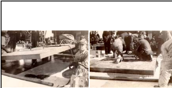
Installing Tower Base Plates
