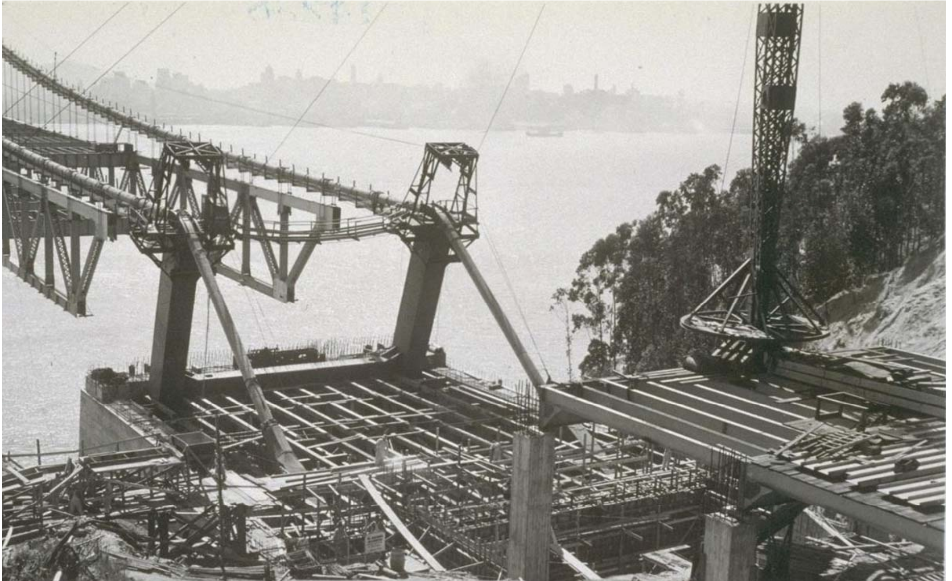
Yerba Buena Anchorage (Approach Viaduct at right) April 1936
