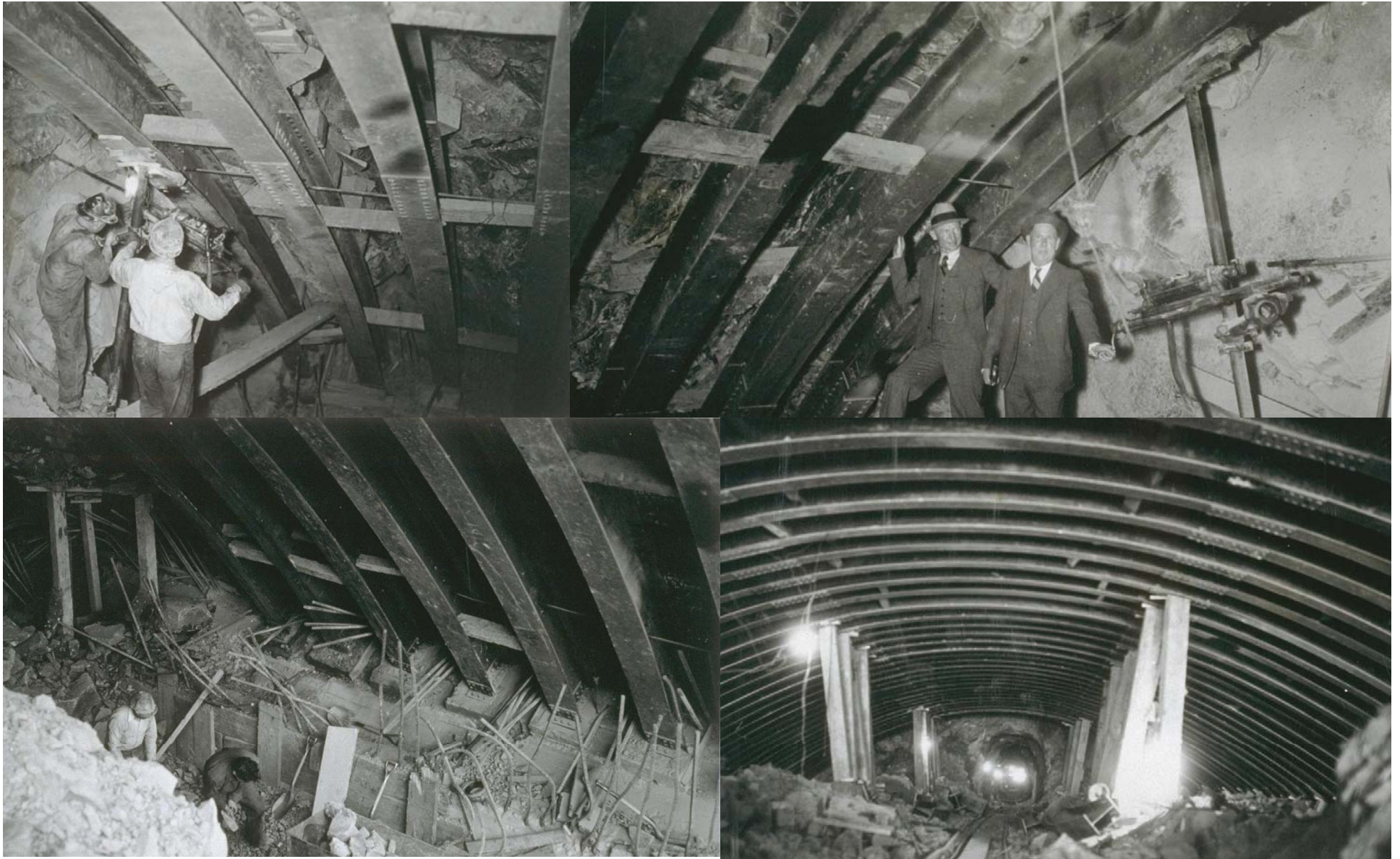
Steel Framing for Tunnel Vault April 1935 (top L&R) / June 1935 (bottom L&R)
