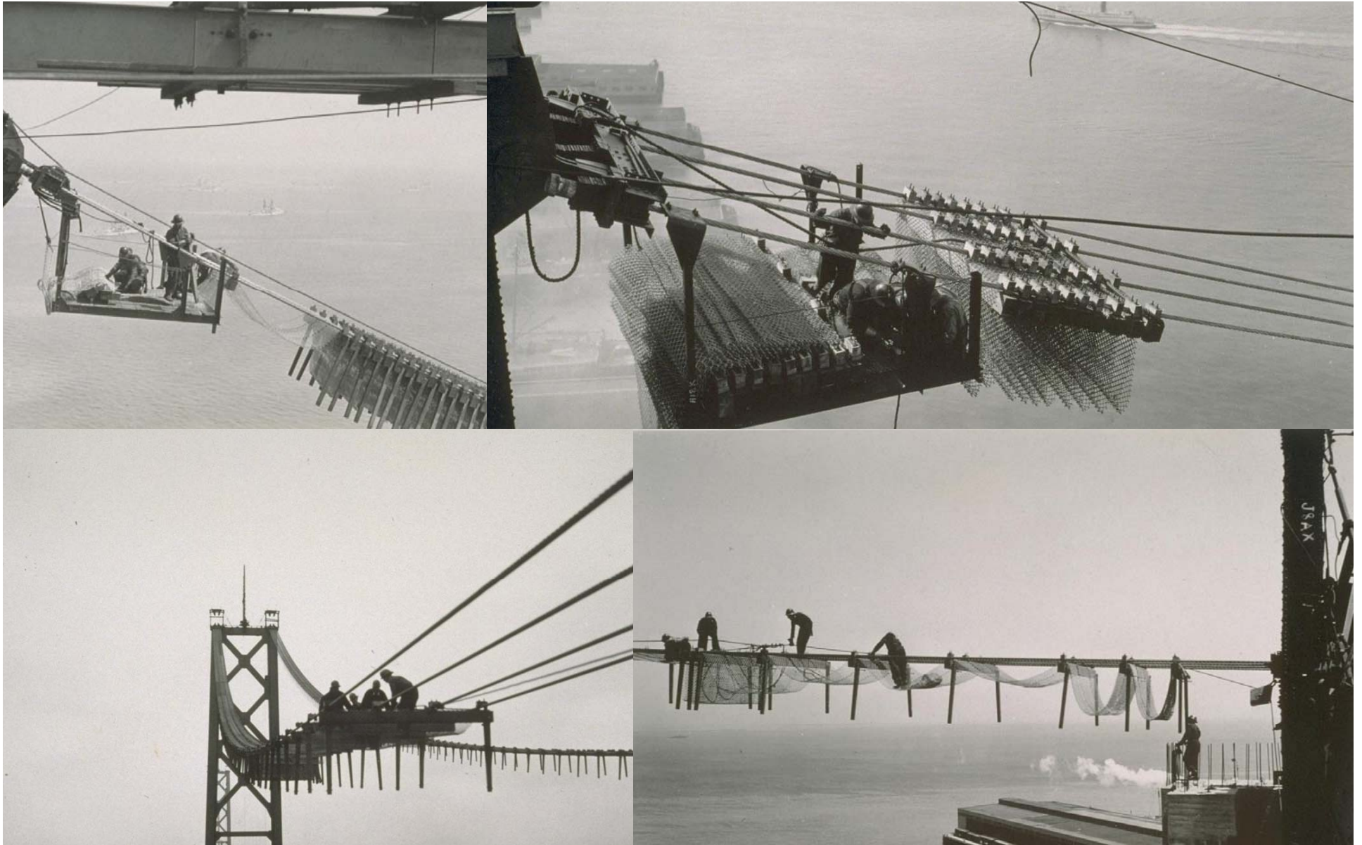
North Footbridge May 1935
