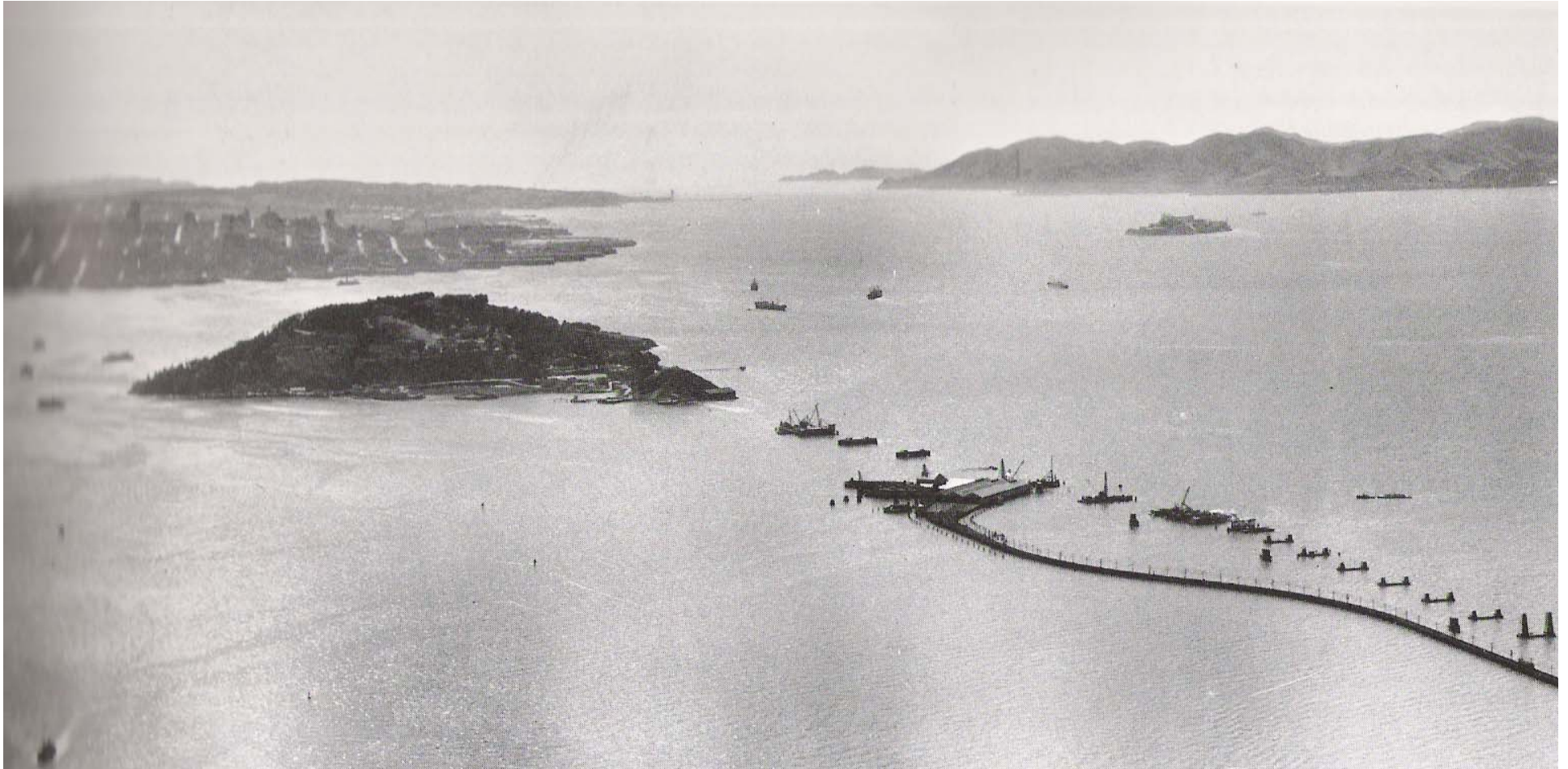
East Bay Piers (under construction)
