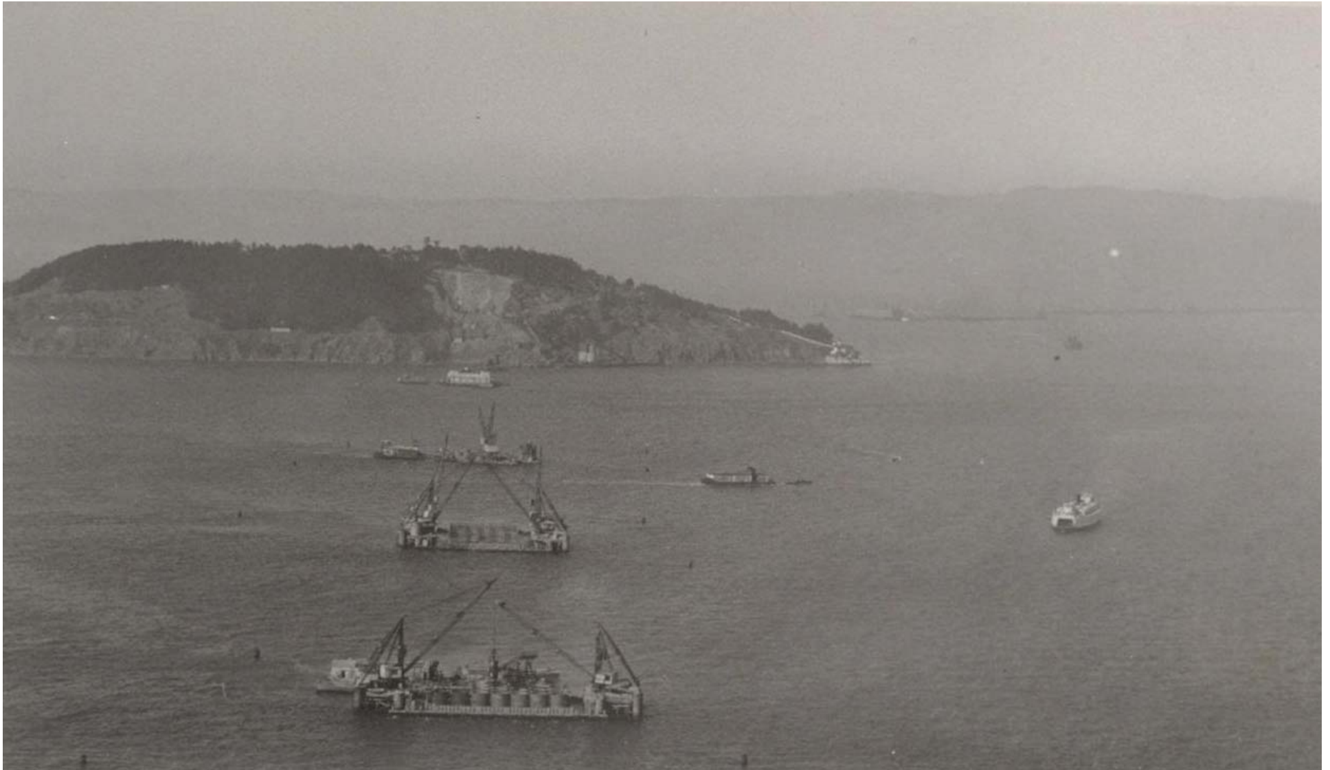
Piers W-3 thru W-6 (under construction - Yerba Buena beyond) May 1934
