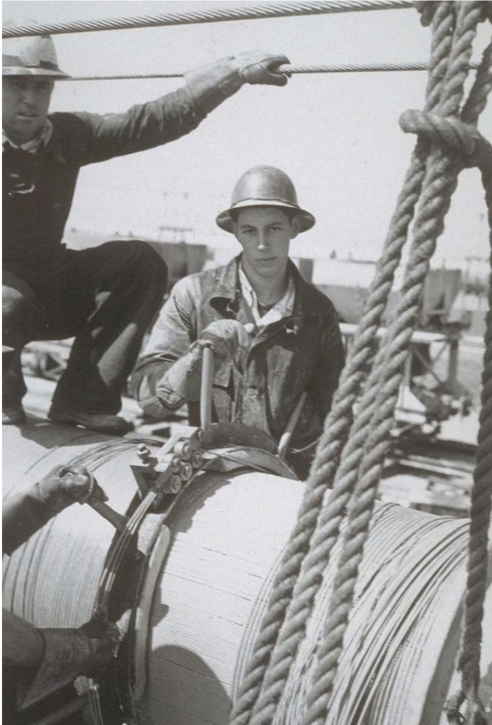
Wrapping the main cable/s with fine galvanized wire 1936
