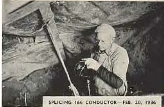
SPLICING 166 CONDUCTOR—FEB. 20, 1936
