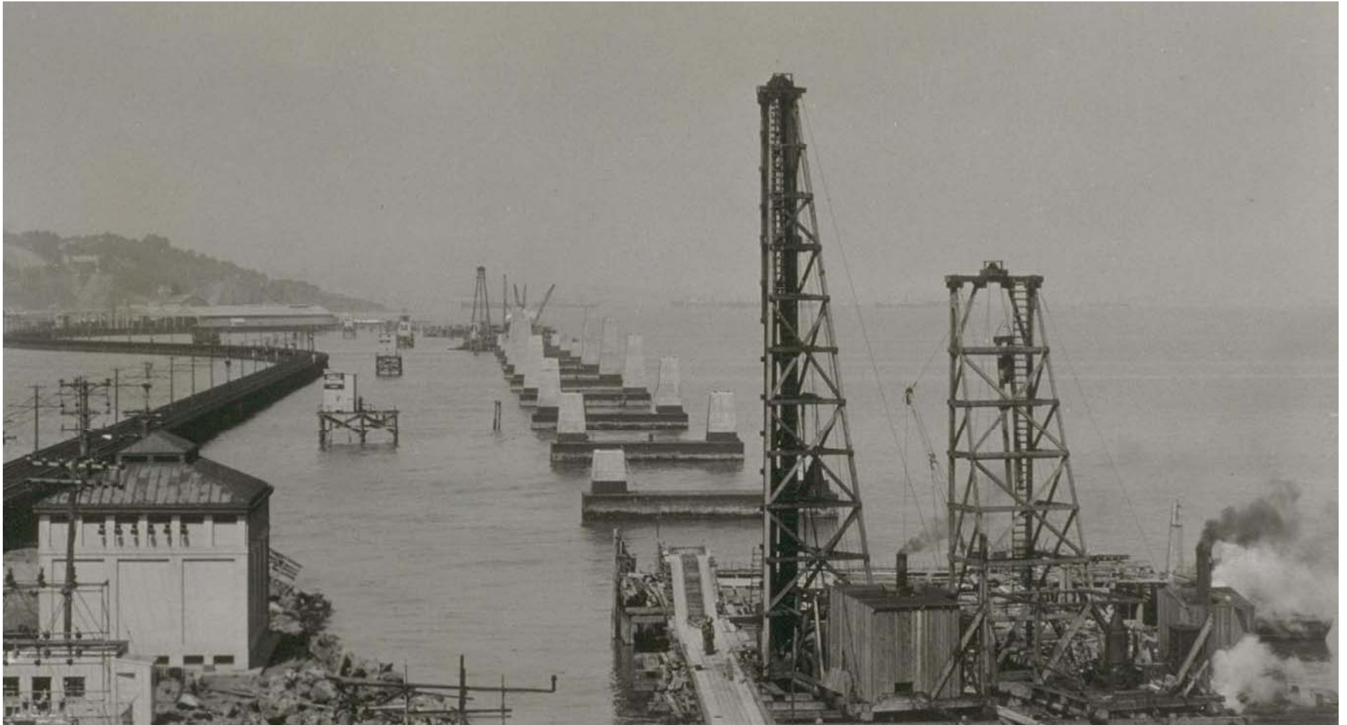
Piers E-22 thru E-14 (Oakland Approach) June 1934
