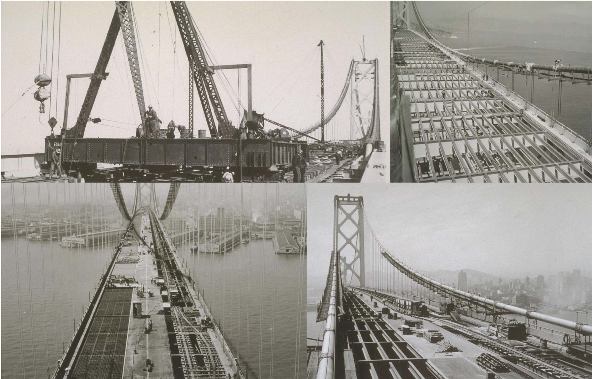
West Suspension-Span deck installation Summer 1936
