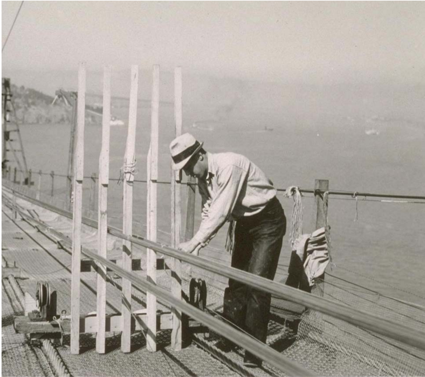
South Cable Strand Separator June 1935
