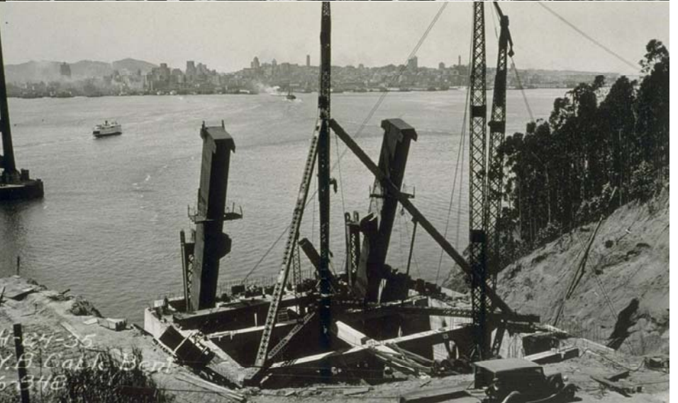
Yerba Buena Anchorage Cable Bents April 1935
