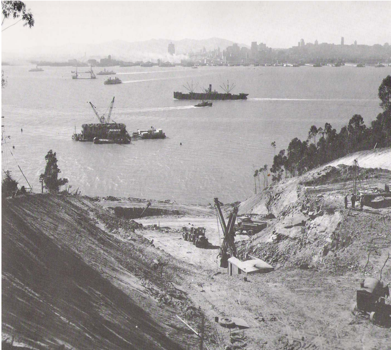
Yerba Buena Anchorage Excavation December 1933
