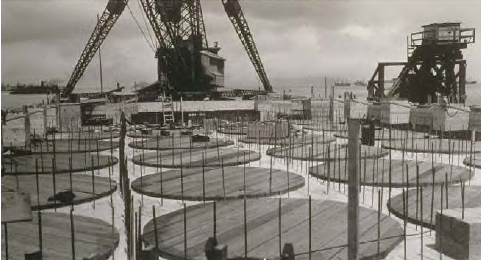
Pier W-3 June 1934
