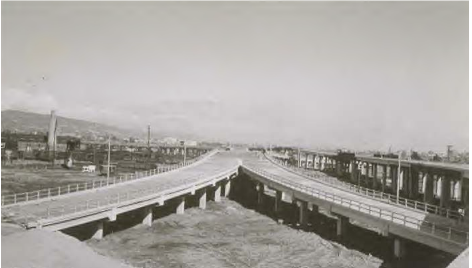
San Francisco Approach (NG and NM Lines – Contract No. 15) May 1936
