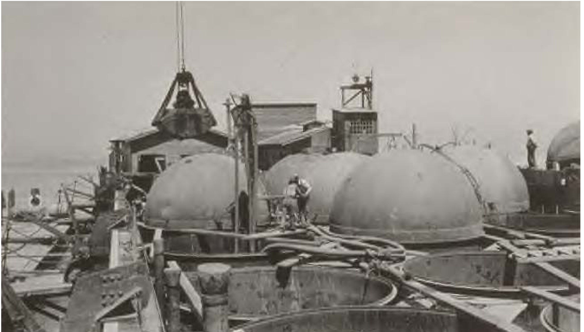
Pier W-5 (May 1934)
