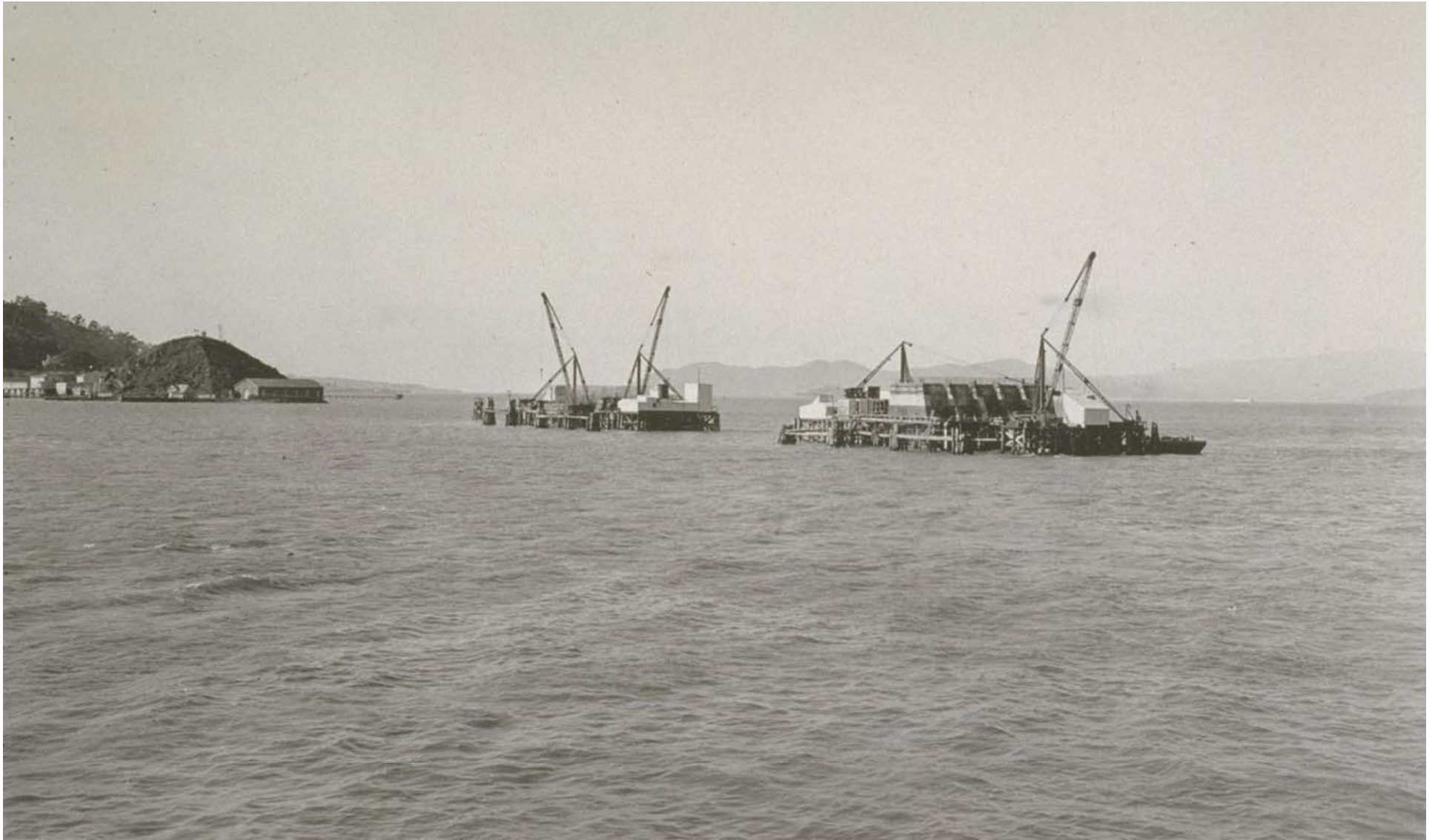
Piers E-4 and E-5 November 1933
