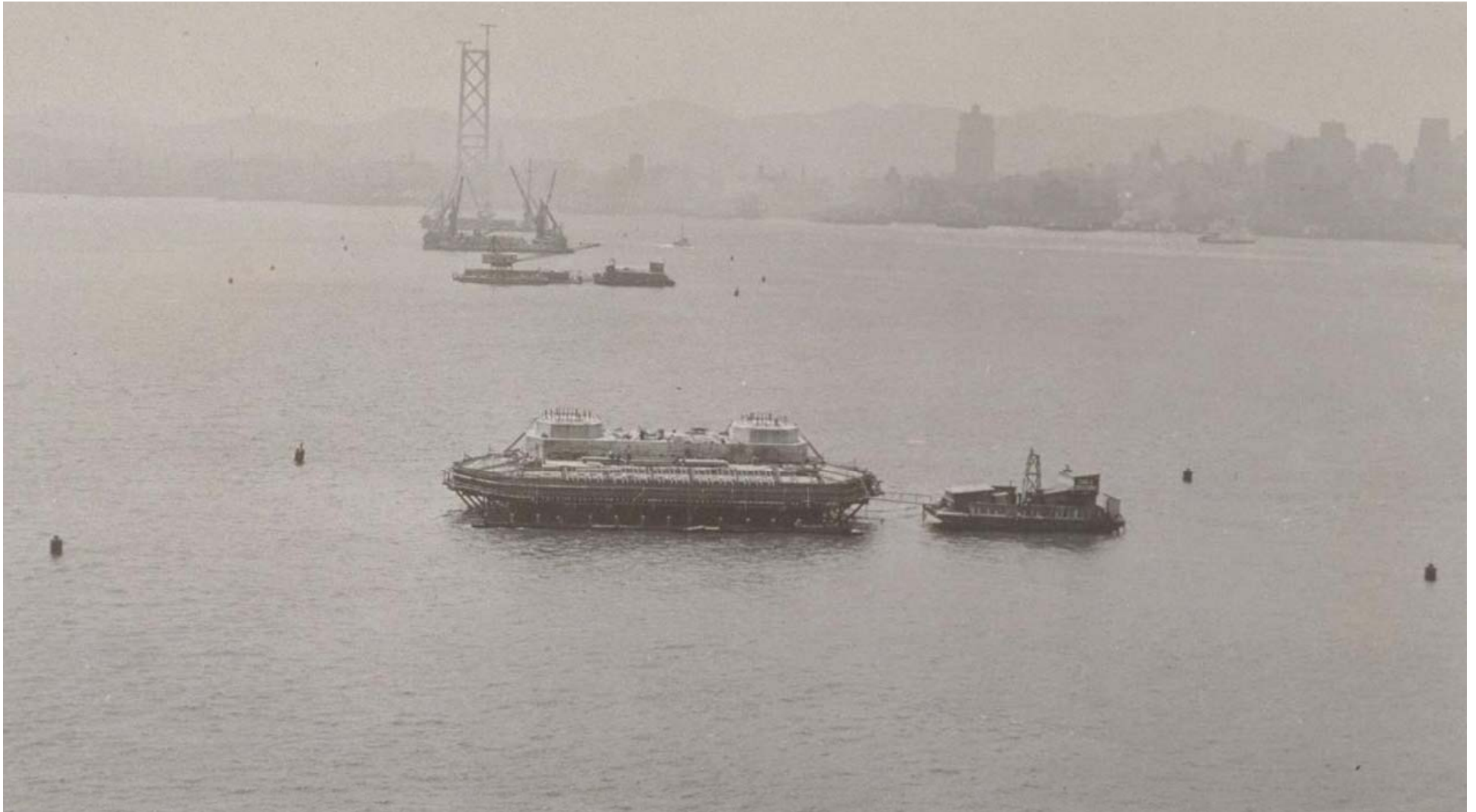
Pier W-6 thru W-3 (note the cantilevered concrete “fender” of Pier W-6 in foreground)
