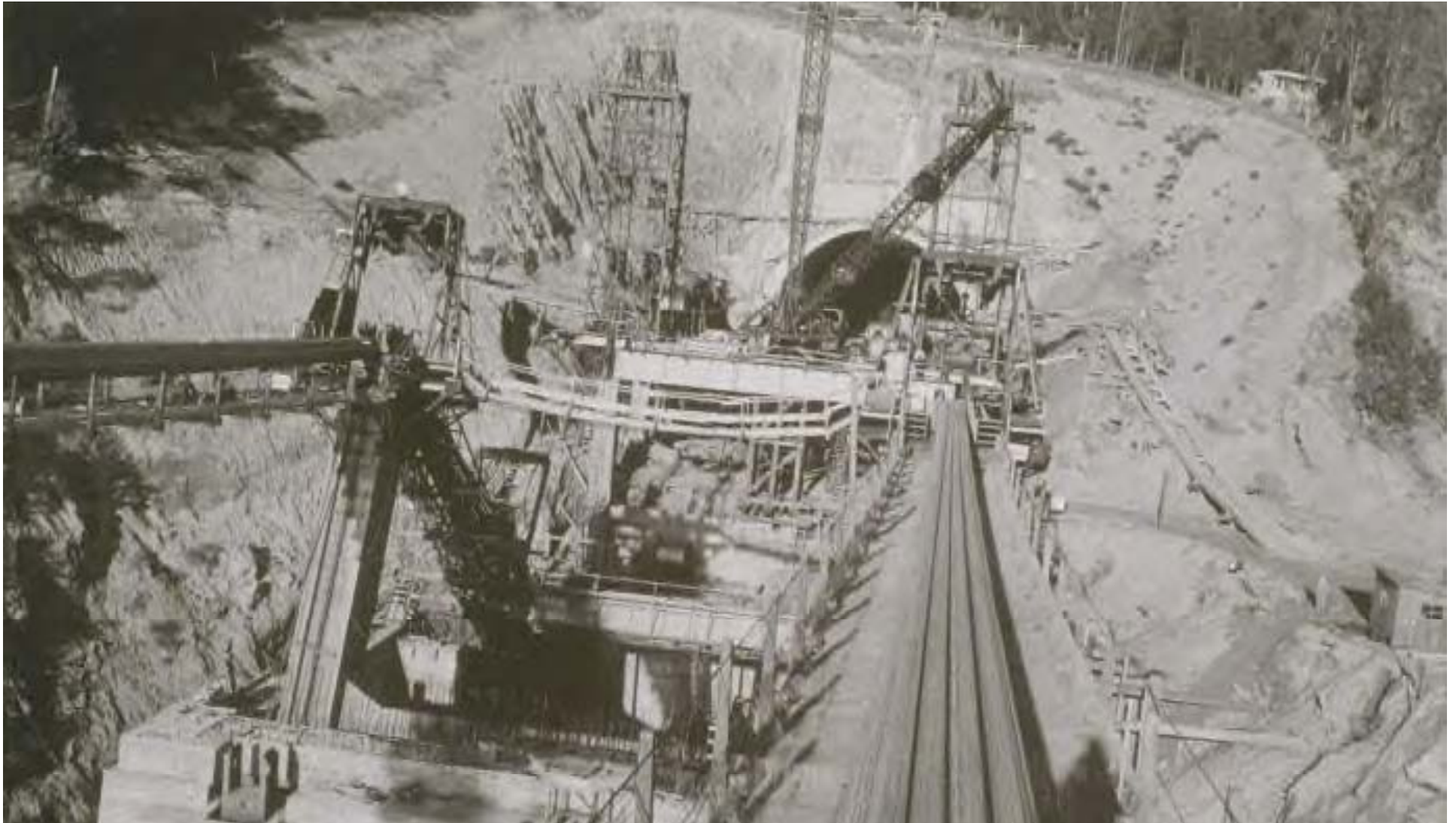
North and South Cables – Yerba Buena Anchorage January 1936
