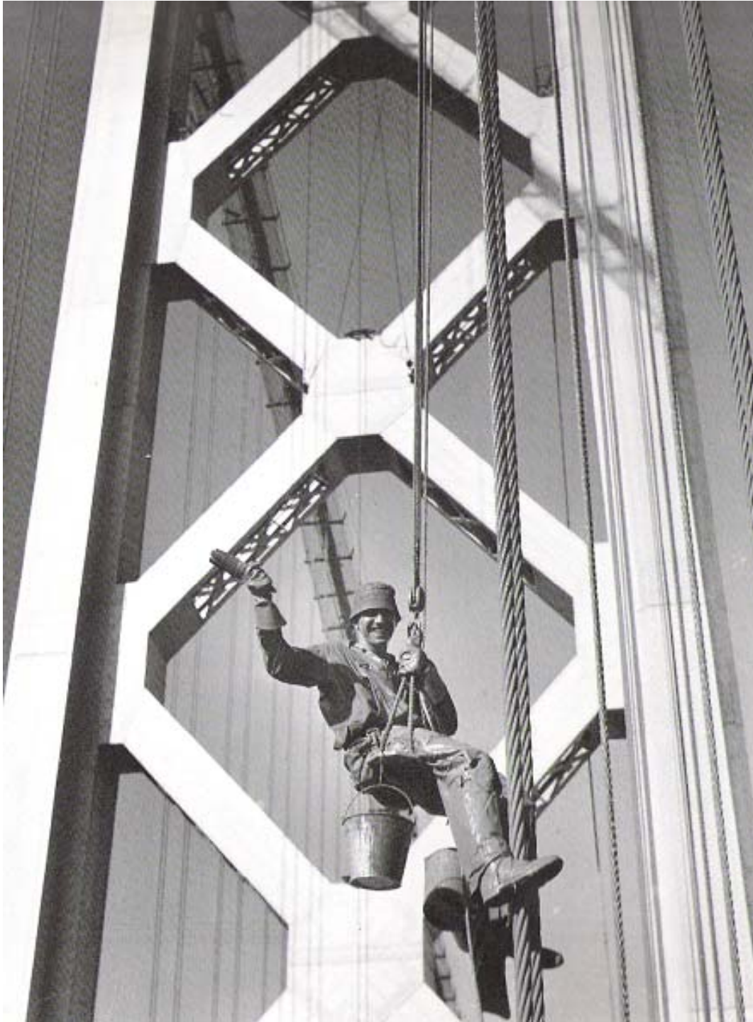
Painting Suspender Cables (between Tower Nos. 5 and 6) May 1936
