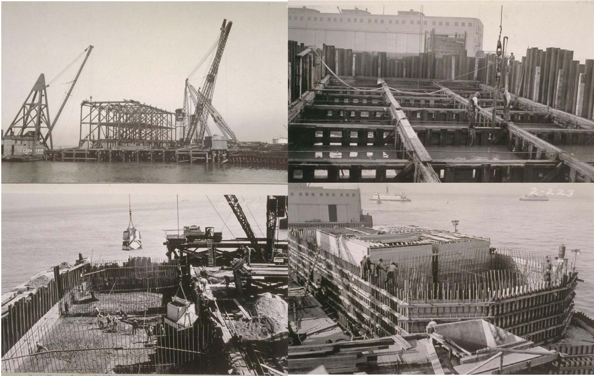
Pier W-2 (under construction, 1933)
