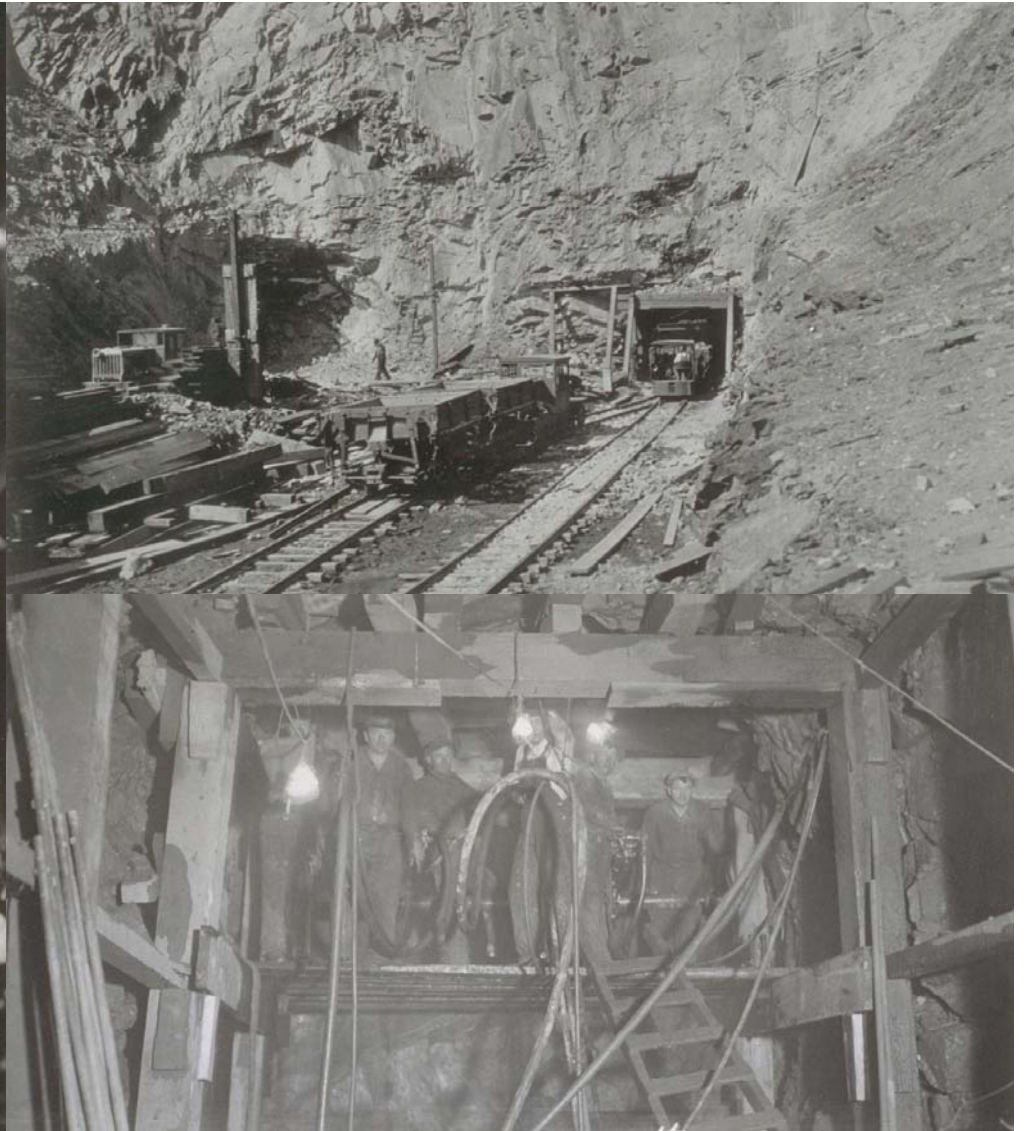
Left – Pilot Tunnel No. 5 (Sept. 1934) Above (top) – Pilot Tunnels Nos. 1 and 2 - Note RR tracks for muck (May 1934) Above – Tunnel No. 2 (July 1934) 467
