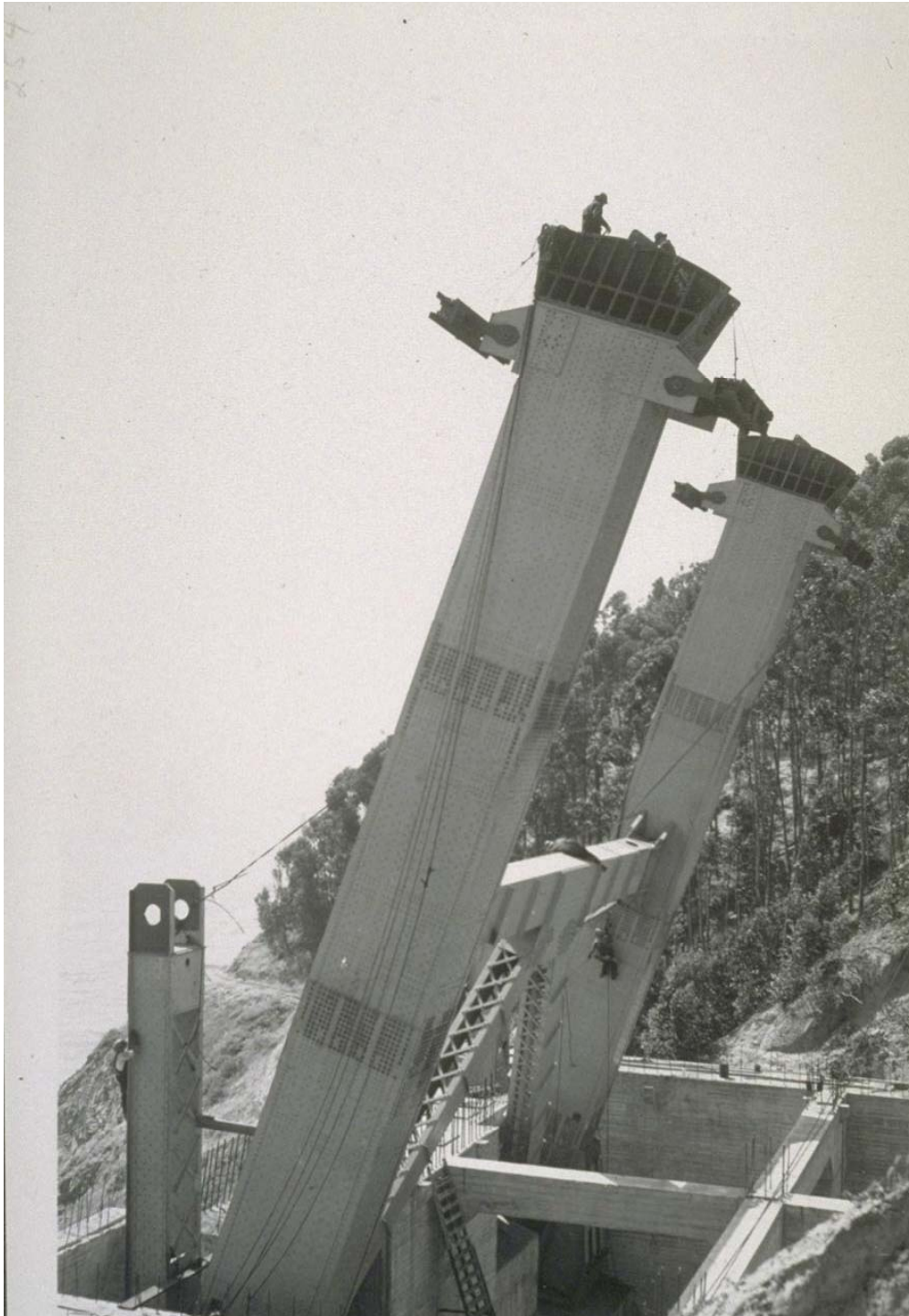
Yerba Buena Anchorage Cable Bents (w/cable saddles in-place) June 1935
