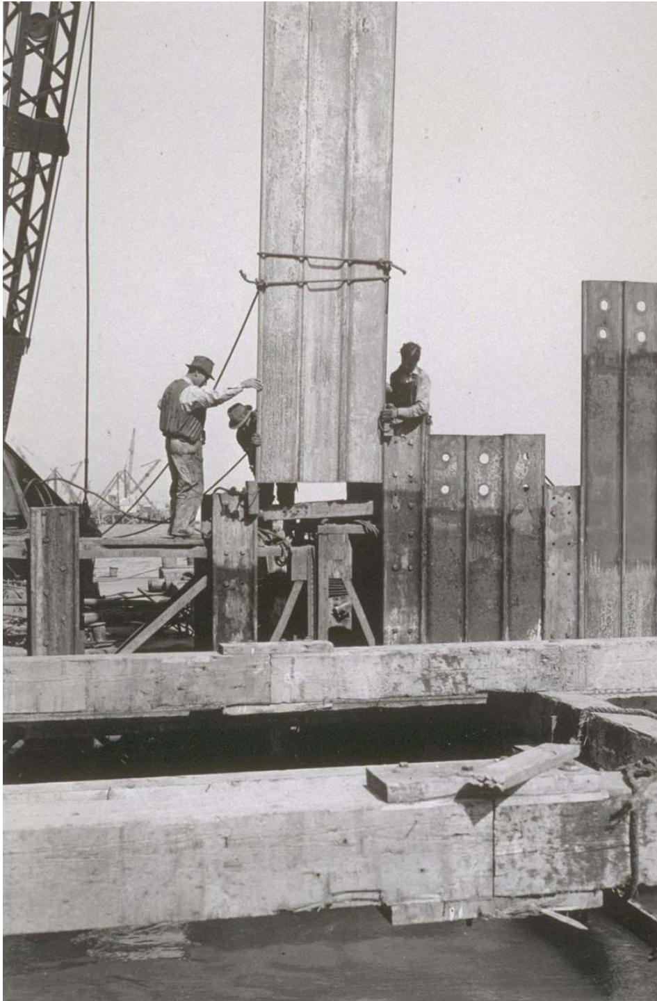
Pier E-2 under construction (September 1934). Built of solid concrete in an open cofferdam and founded on bedrock 45-feet below water level.
