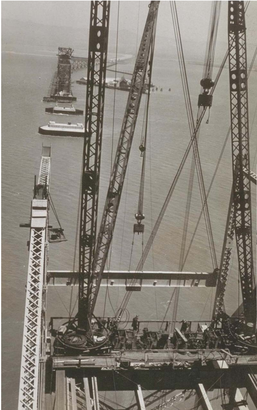
Left—traveler derrick (at work) Right— closing the suspension-span gap (March 1935)
