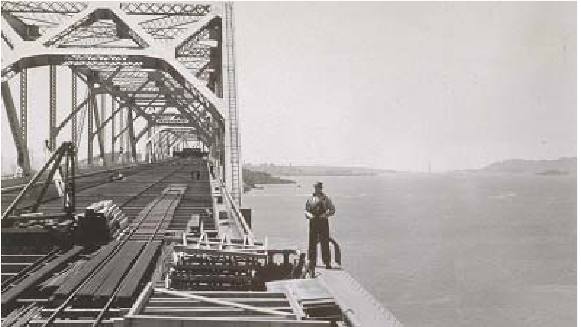
Through-Deck Truss Transition (atop Pier E-9) April 1935
