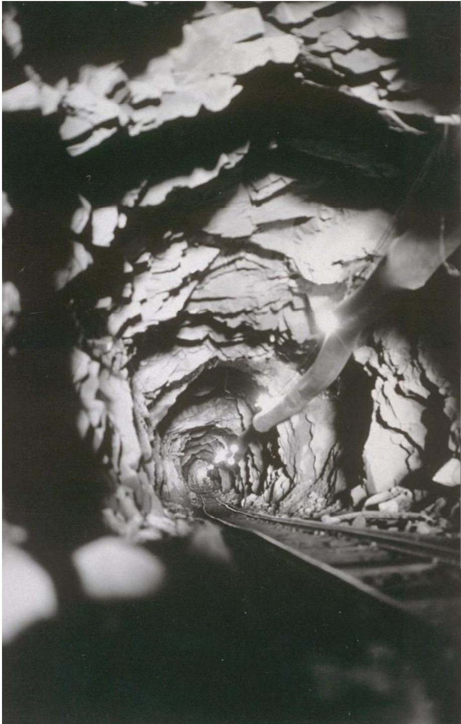
Left – Pilot Tunnel No. 5 (Sept. 1934) Above (top) – Pilot Tunnels Nos. 1 and 2 - Note RR tracks for muck (May 1934) Above – Tunnel No. 2 (July 1934) 467
