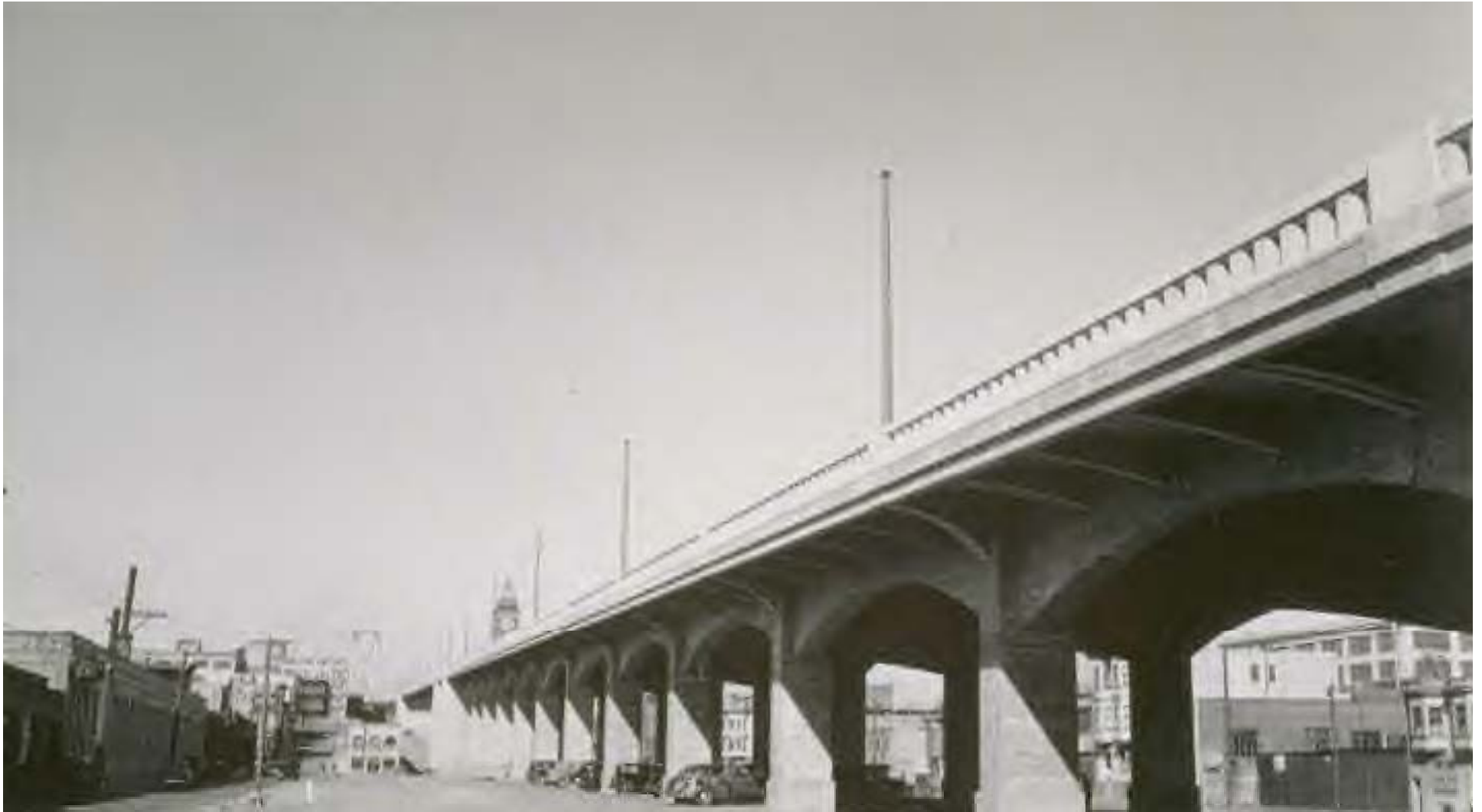
San Francisco Approach (Contract No. 15) September 1936
