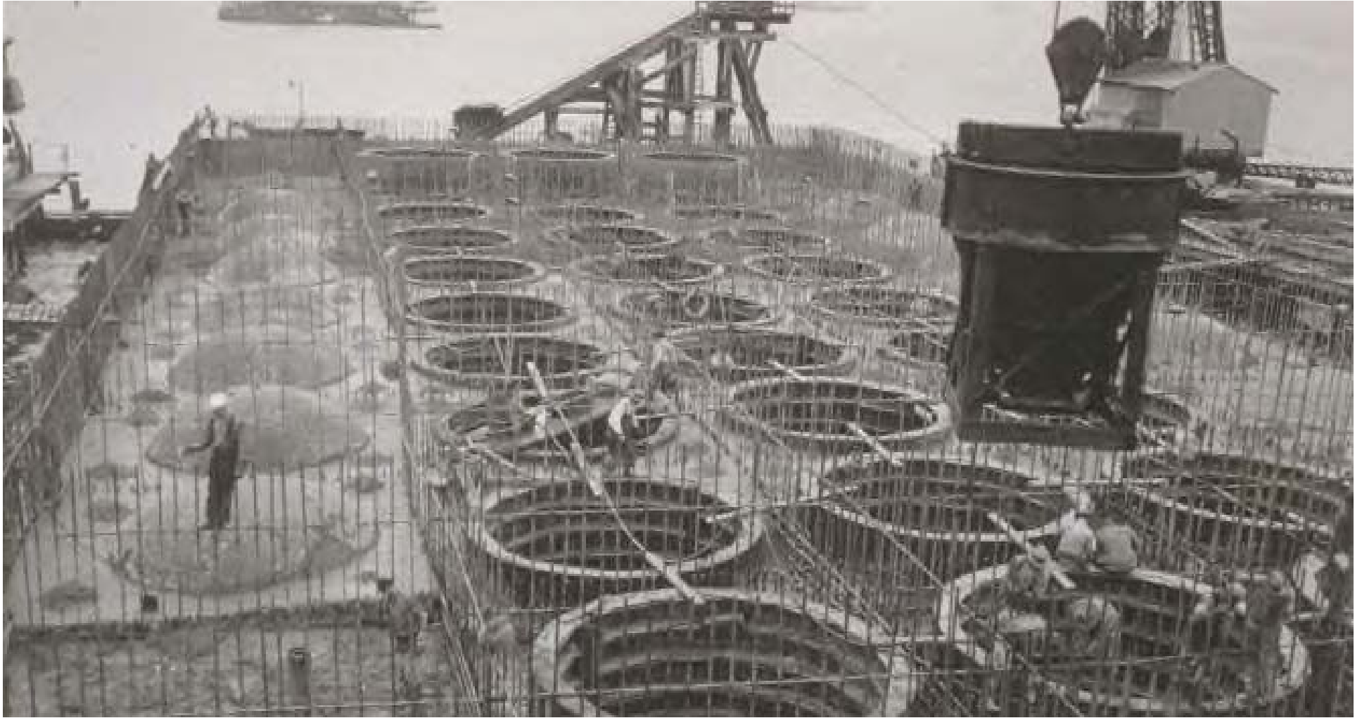
Pier W-4 August 1934
