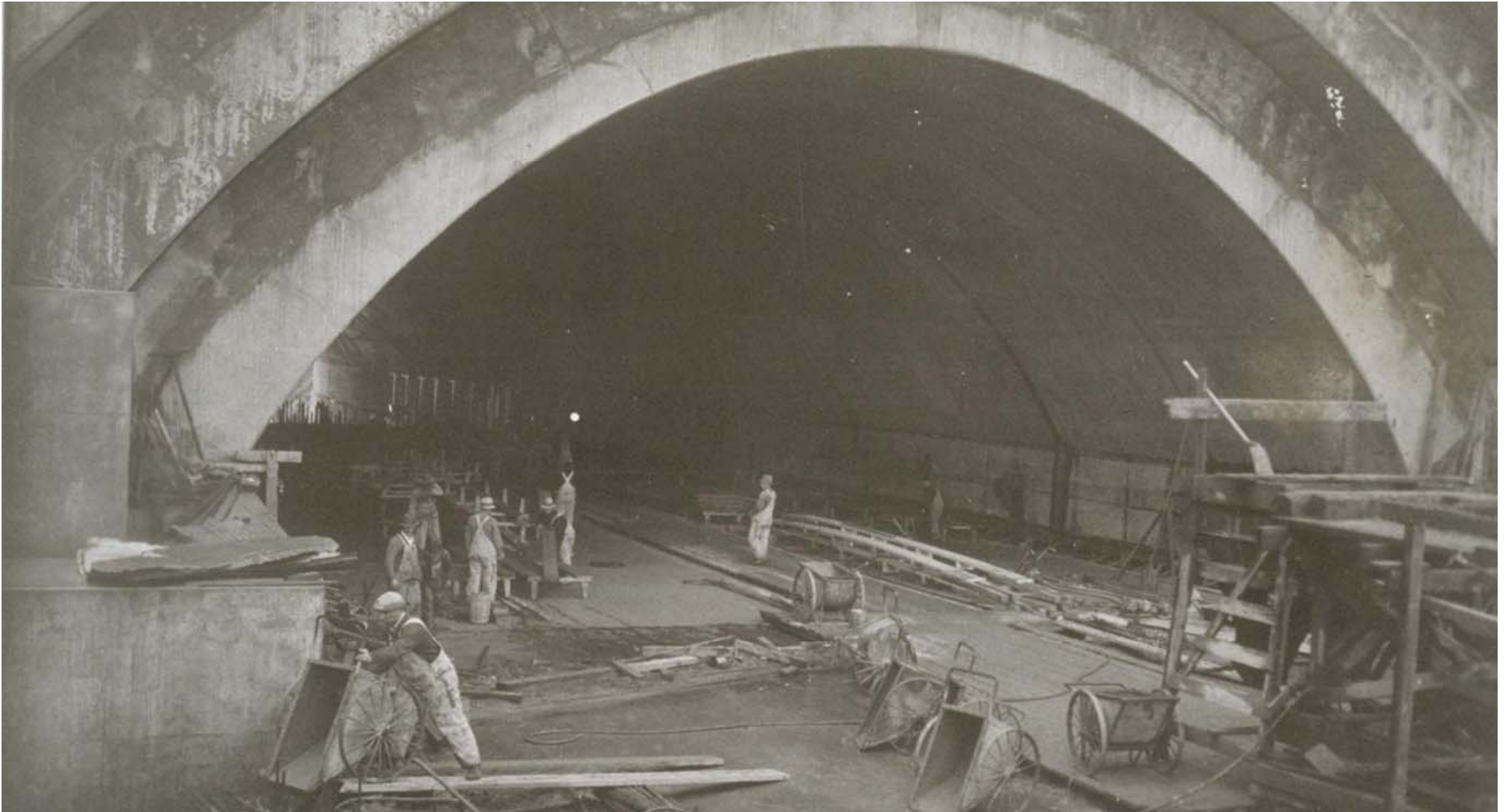
Tunnel Upper Deck (at West Portal) January 1936
