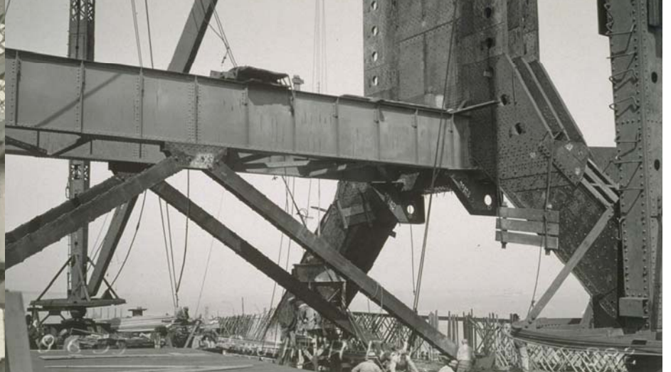
Central Anchorage A-Frame 1935
