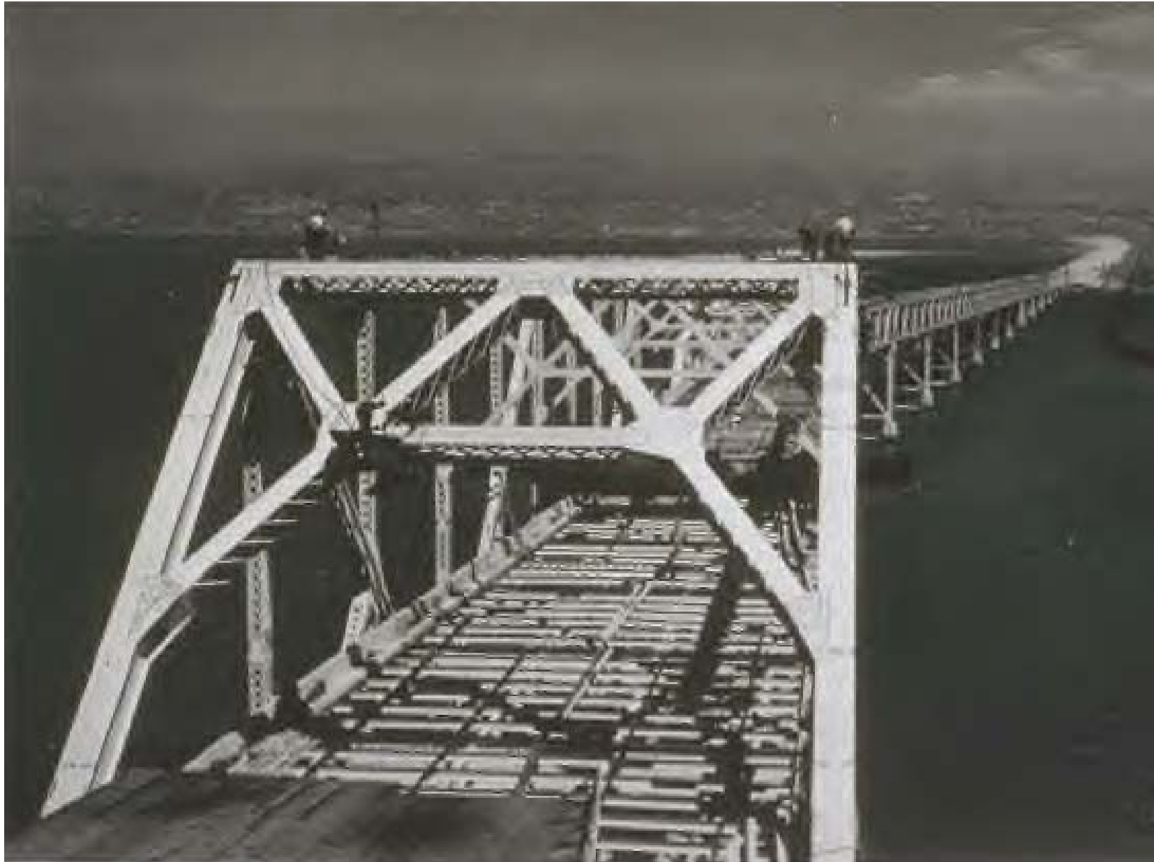
Span E-7 (Through Truss) – deck support in-place April 1935
