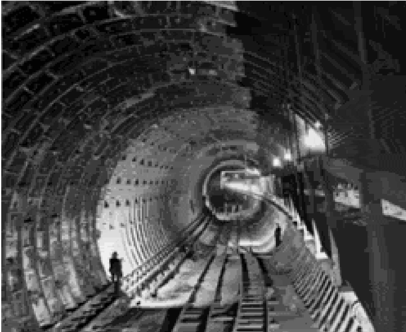
Brooklyn Battery Tunnel (under construction)
