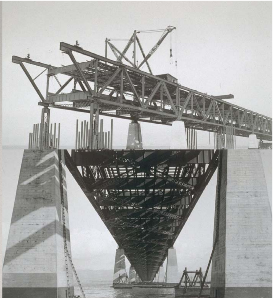
Left – traveler derrick Above – concrete (tower) pier supported deck truss spans – Oct./Nov. 1934
