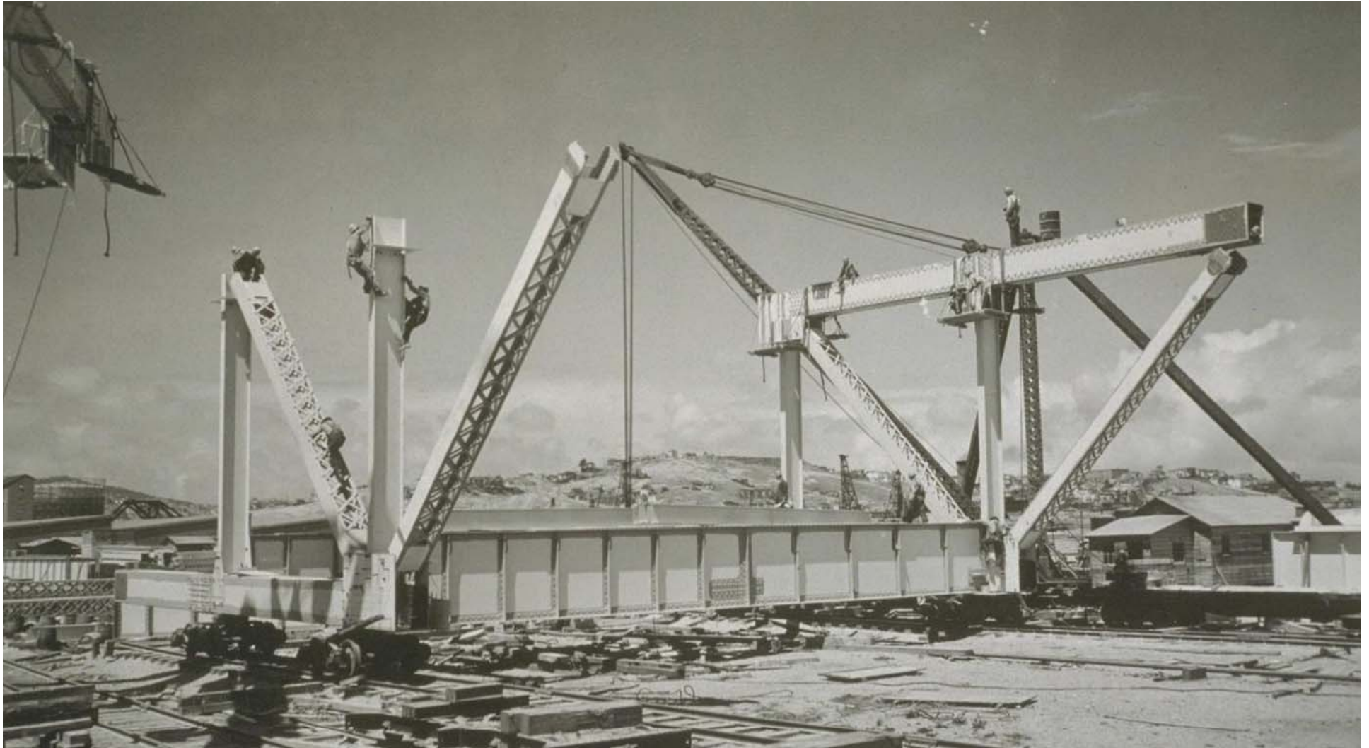
Unit No. 144 being assembled (at Islais Creek ) April 1936
