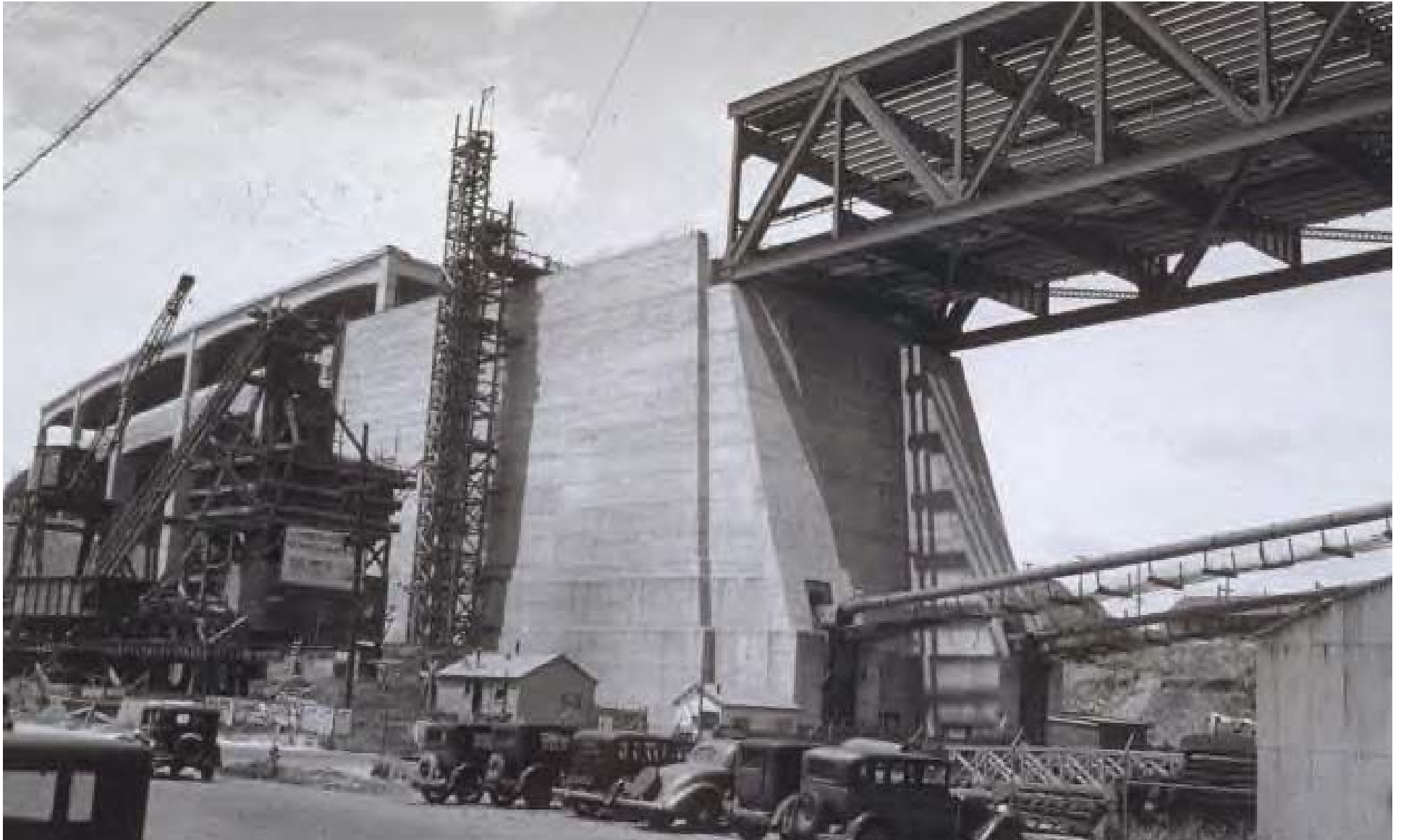
San Francisco Anchorage (Contract No. 3) May 1936
