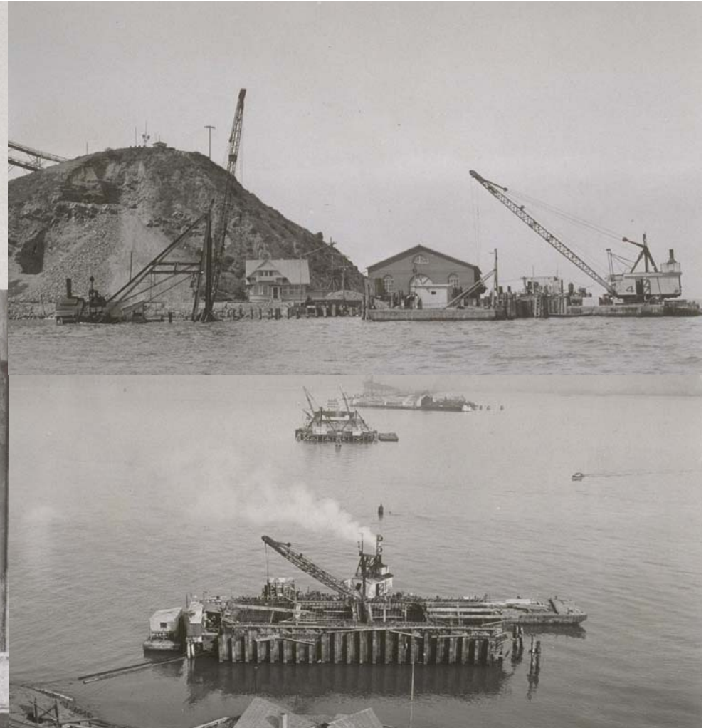
Pier E-2 under construction (September 1934). Built of solid concrete in an open cofferdam and founded on bedrock 45-feet below water level.
