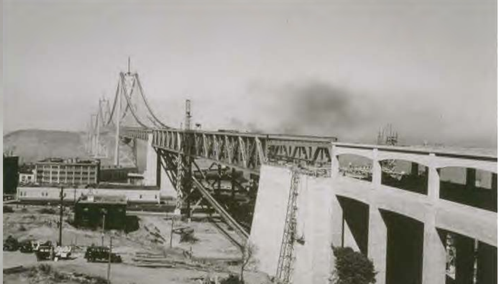
Left – Pier W-1 (April 1935) Above (top) – June 1935 (Pier W-1 at left) Above – August 1935 – Pier W-1 (left) supporting east-end of trusses
