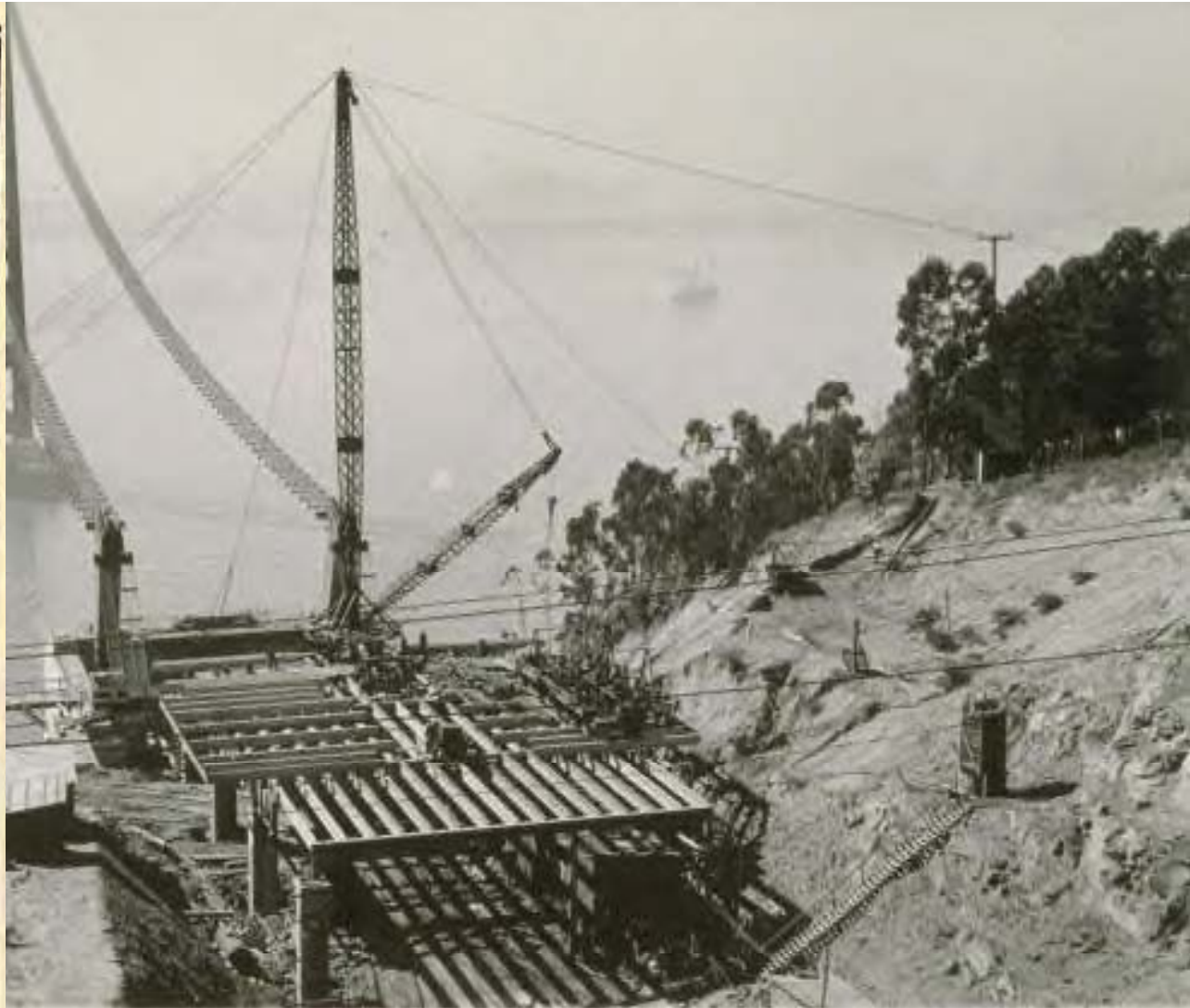
Yerba Buena Anchorage (under construction) (Contract No. 5) June 1935
