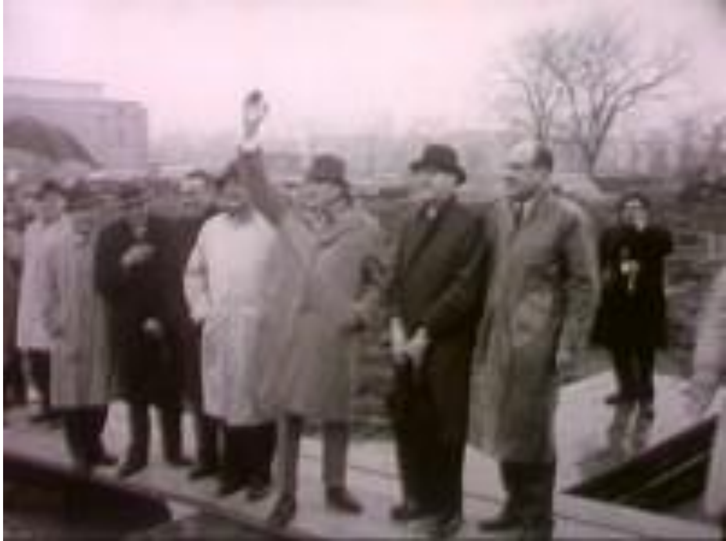
Rene Legrain Eiffel gives the signal to start construction of Unisphere – theme symbol of the 1964/65 NYWF at the “first steel” ceremonies for Unisphere, held on Wednesday, March 6 th 1963
