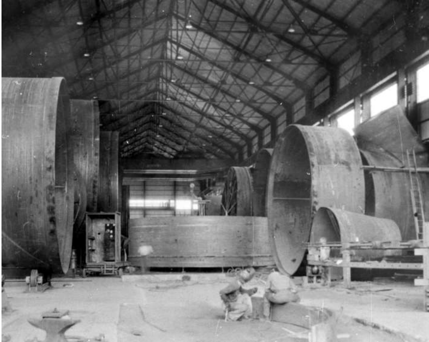
View looking (longitudinally) through the Babcock & Wilcox Co. plant showing the fabrication of thirty-foot diameter steel Penstock sections; August 1934)
