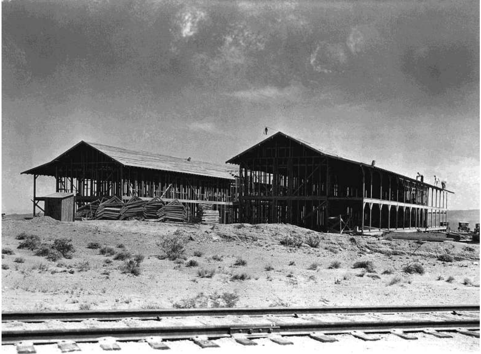
Six Companies Bunkhouses under construction at Boulder City
