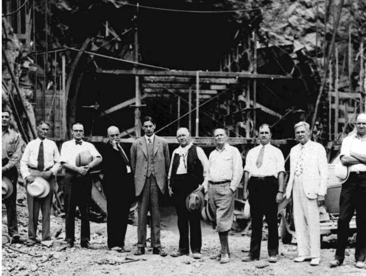
Inspection party in front of the outlet portal of a diversion tunnel. City Manager Sims Ely , Construction Engineer Walker Young , Six Companies Director H.J. Kaiser , Interior Secretary Ray Wilbur , Six Companies President W.A. Bechtel , MWD Engineering Chairman W.L. Honnald , Six Companies Director S.D. Bechtel , MWD President W.P. Whitsett , Six Co. Superintendent Frank Crowe (September 1932).
