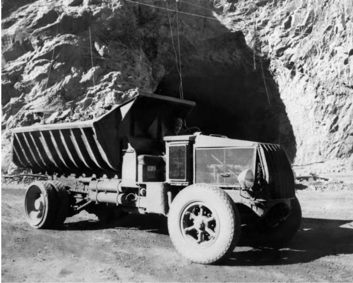
One of the Six Companies' Mack trucks (in front of the upper portal of Diversion Tunnel No. 2). This truck has nine cubic yards capacity (note the steel canopies over the drivers' heads on all the trucks; January 1932).
