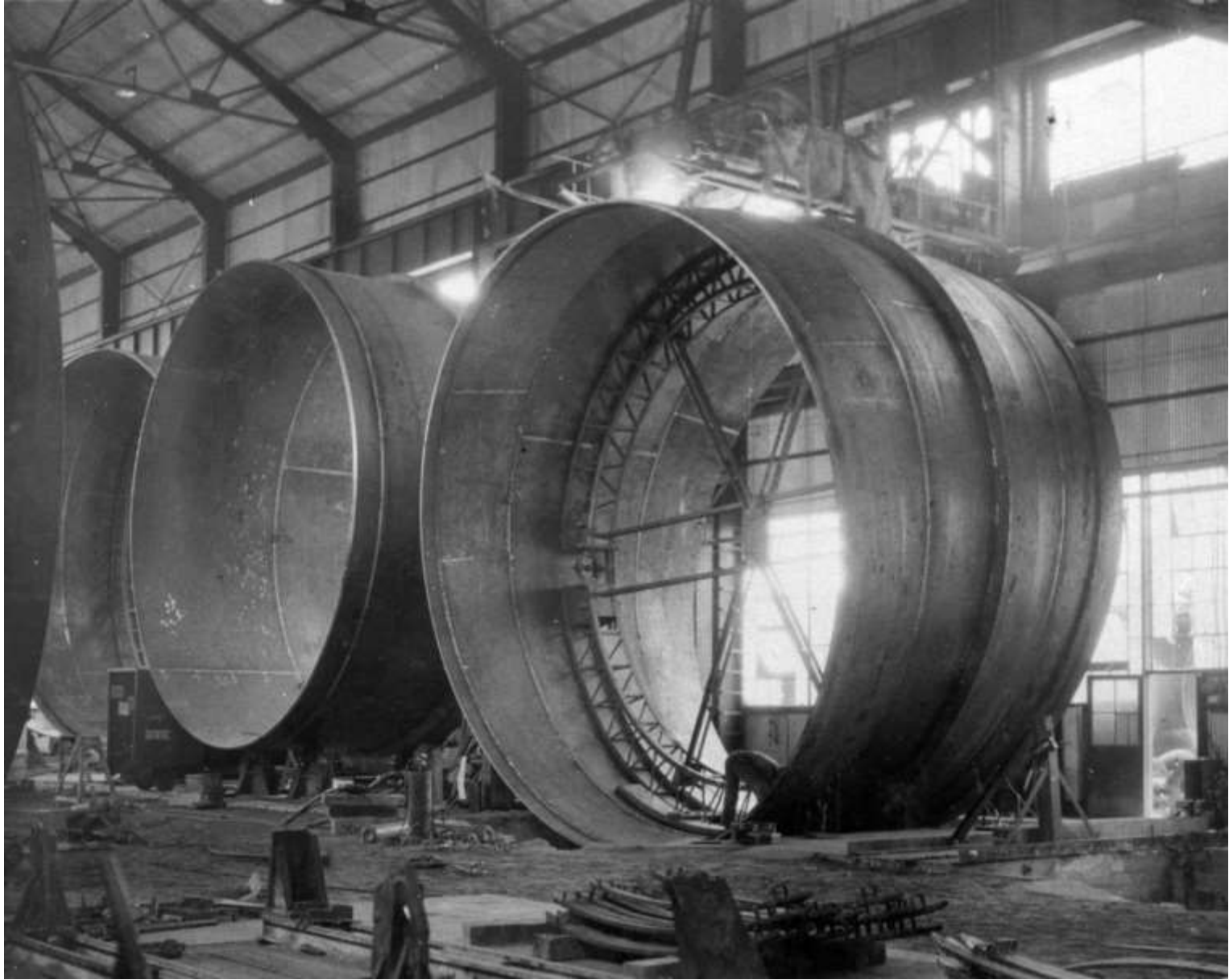
Interior view of the Babcock & Wilcox Co. plant showing the fabrication of thirty-foot diameter steel Penstock sections (August 1934)
