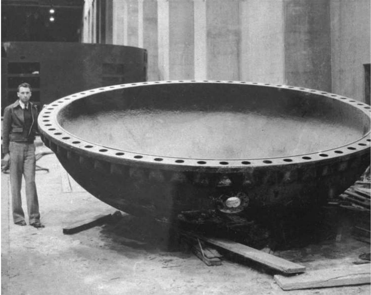
Testing bulkhead for scroll case of 115K-HP Turbine (power plant; November 1935)
