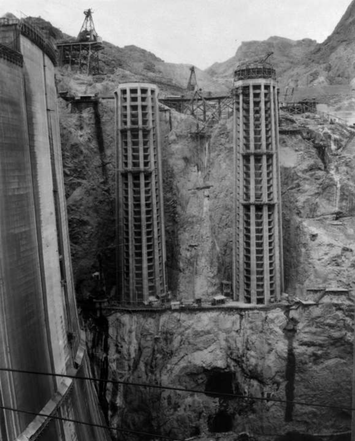
Upstream face of Dam and the Nevada Intake Towers (January 1935)
