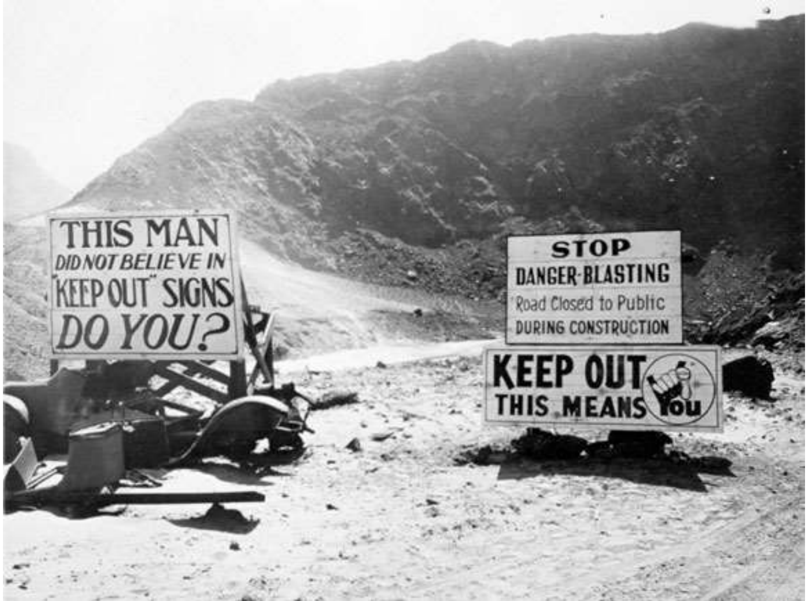
Safety signs put up by insurance company (August 1931)
