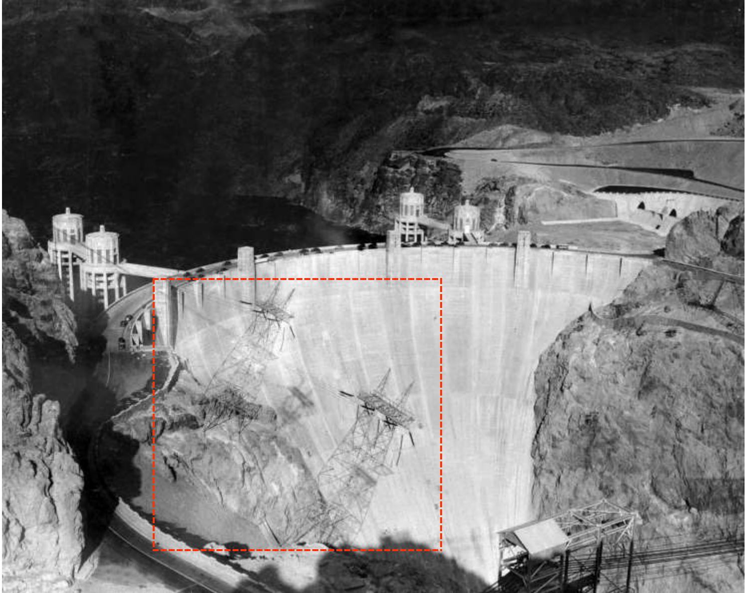
Boulder Canyon. Hoover Dam, Intake Towers and the rim towers (for Units N-1 to N-4). View from the Elks' Flag Pole Point (April 1938)
