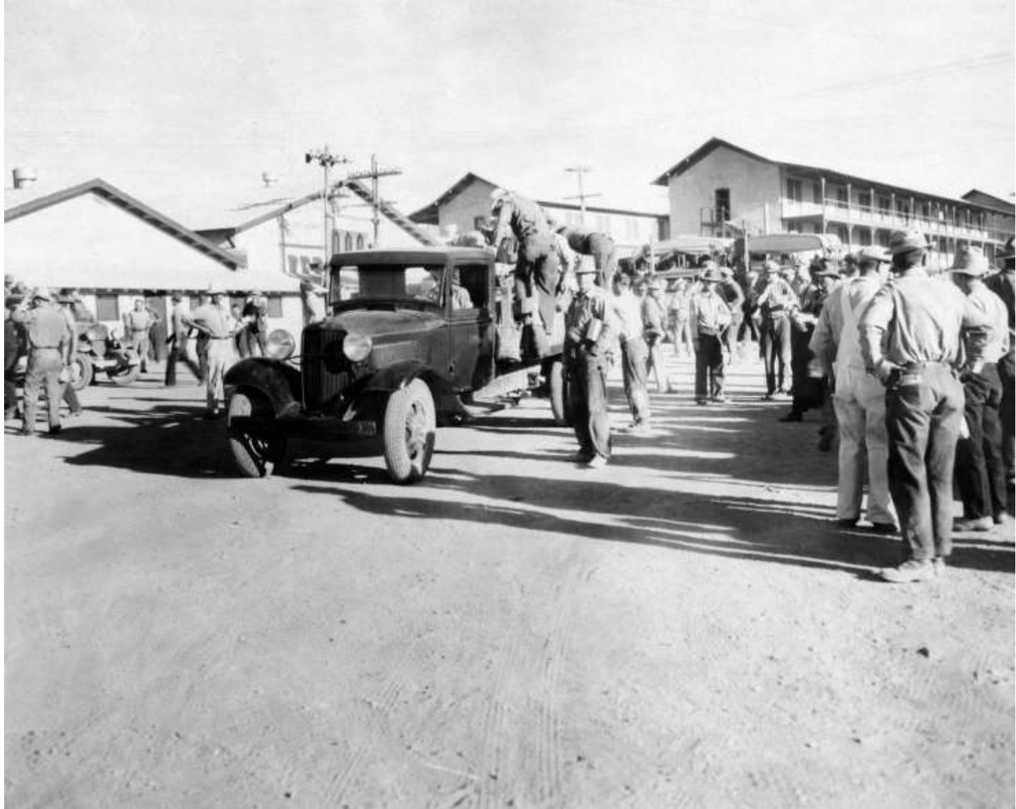
Workmen loading-out for the canyon on the day shift (in front of the Six Companies' Mess Hall, Dormitories in background)
