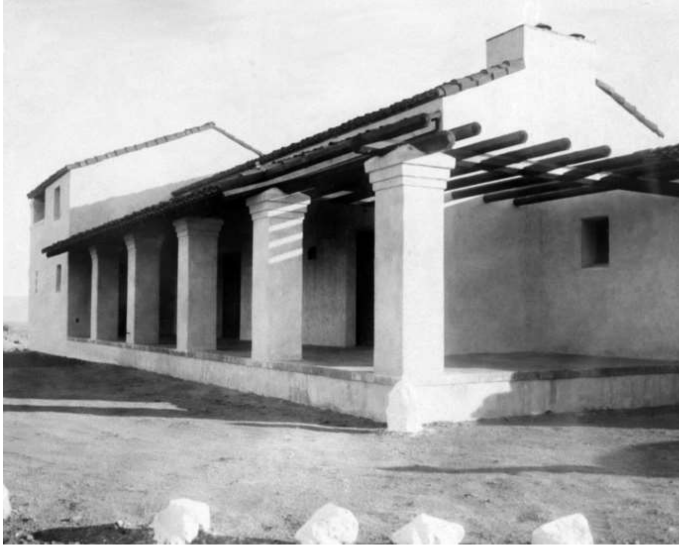
Front view of the Guest House showing the covered veranda which afforded a view of scenic grandeur across Hemenway Wash and the reservoir which was created when Hoover Dam was completed
