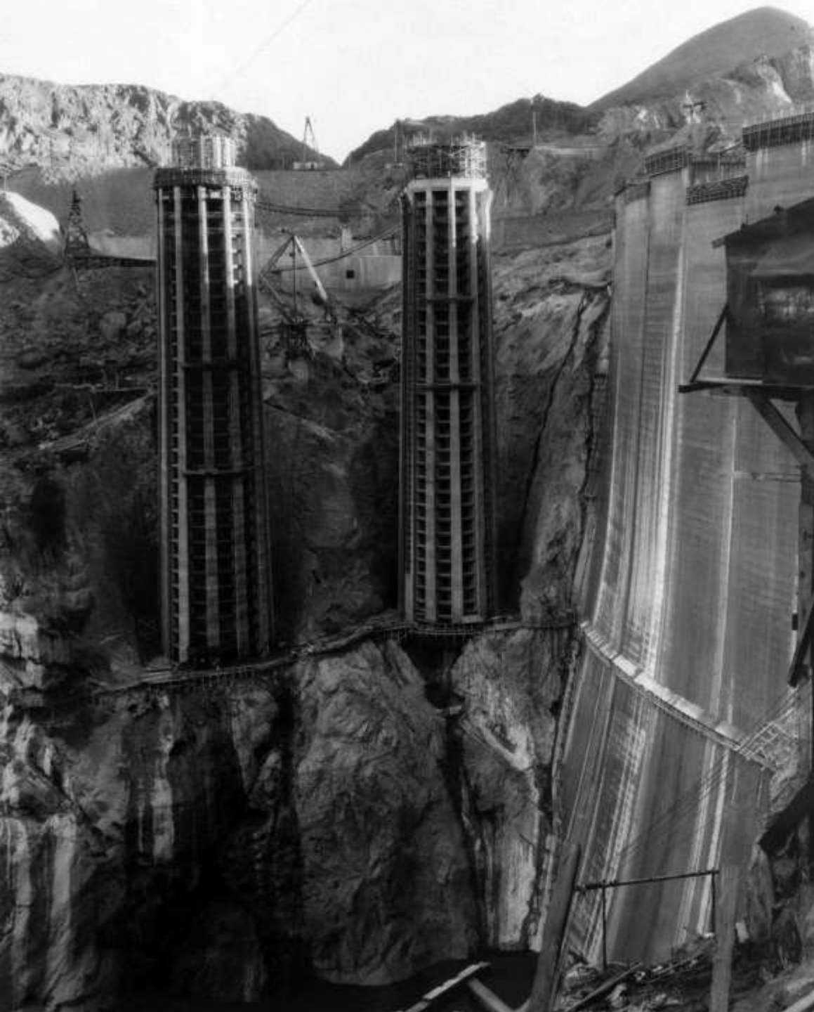
Upstream face of Dam and the Arizona Intake Towers (January 1935)
