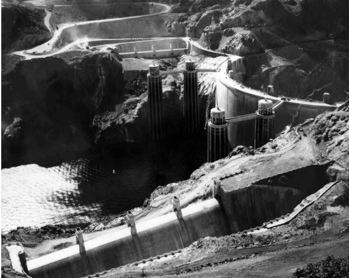
Looking downstream (from the Nevada side) showing Hoover Dam, spillways, Intake Towers, etc. Note the general clean-up and road work; also the Intake Tower lanterns in place (September 1935).
