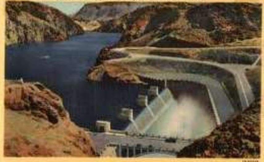
Lake Mead Flowing over Spillway Gates, Hoover (Boulder) Dam
