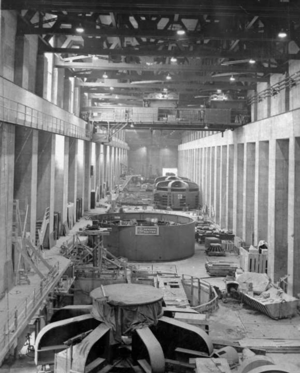
Left: interior view of the Nevada wing of the Powerhouse showing progress of generator installations (July 1936)
