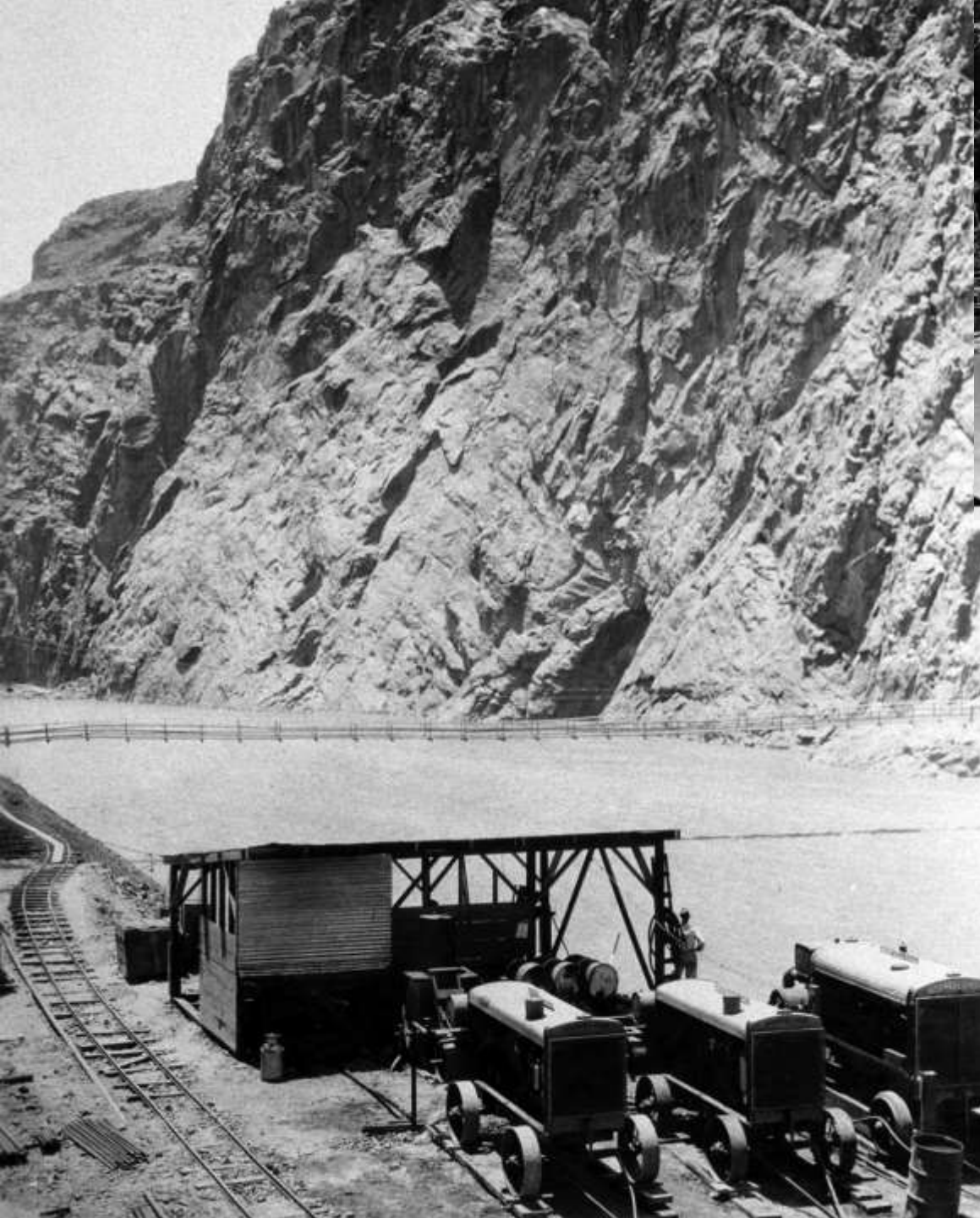
Left: Arizona Diversion Tunnel Adits compressor station (June 1931)
