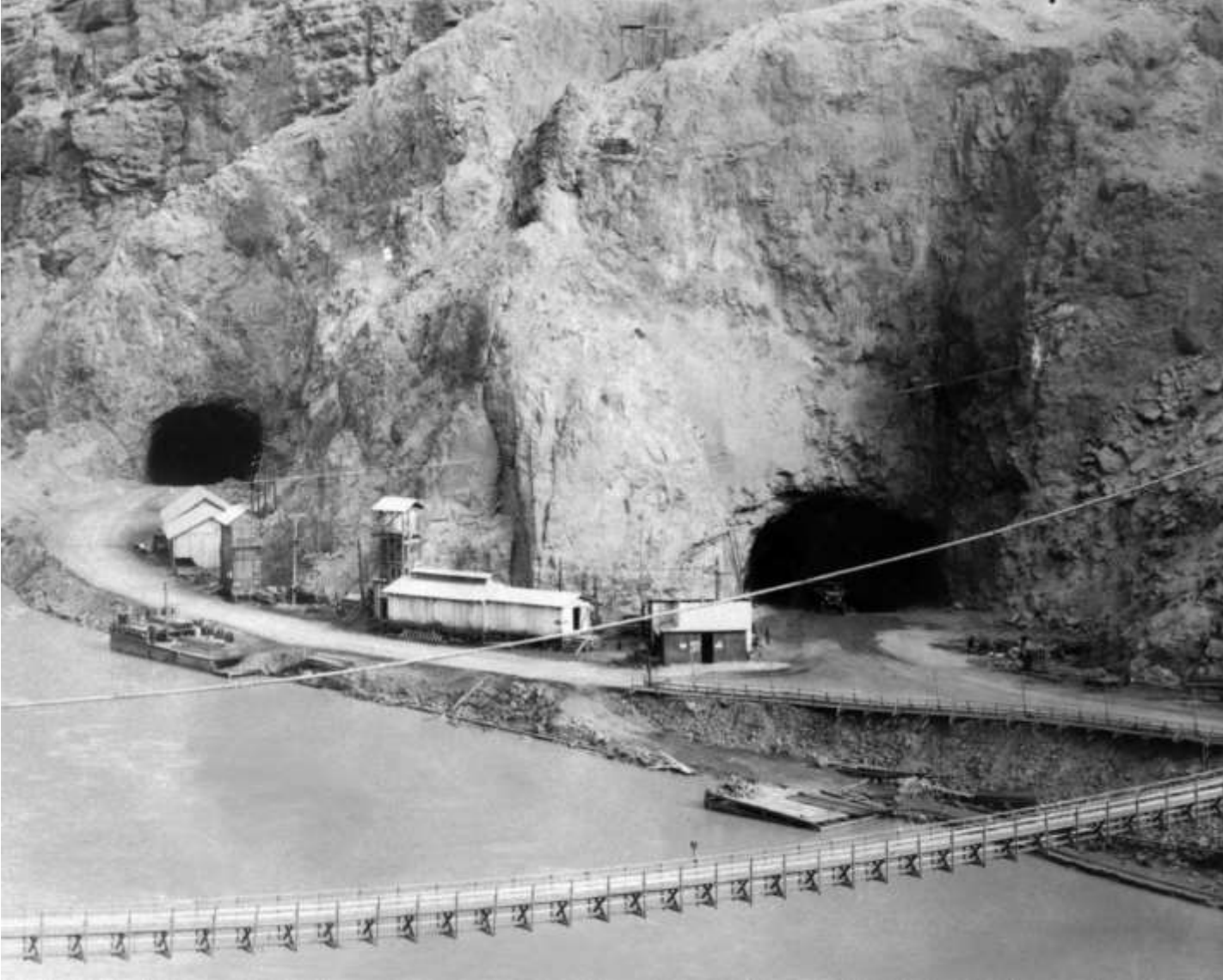
The downstream portals of Diversion Tunnels 3 and 4 on the Arizona side (the bridge in the foreground - in addition to being a foot-walk, carried a six inch compressed air-line; November 1932)
