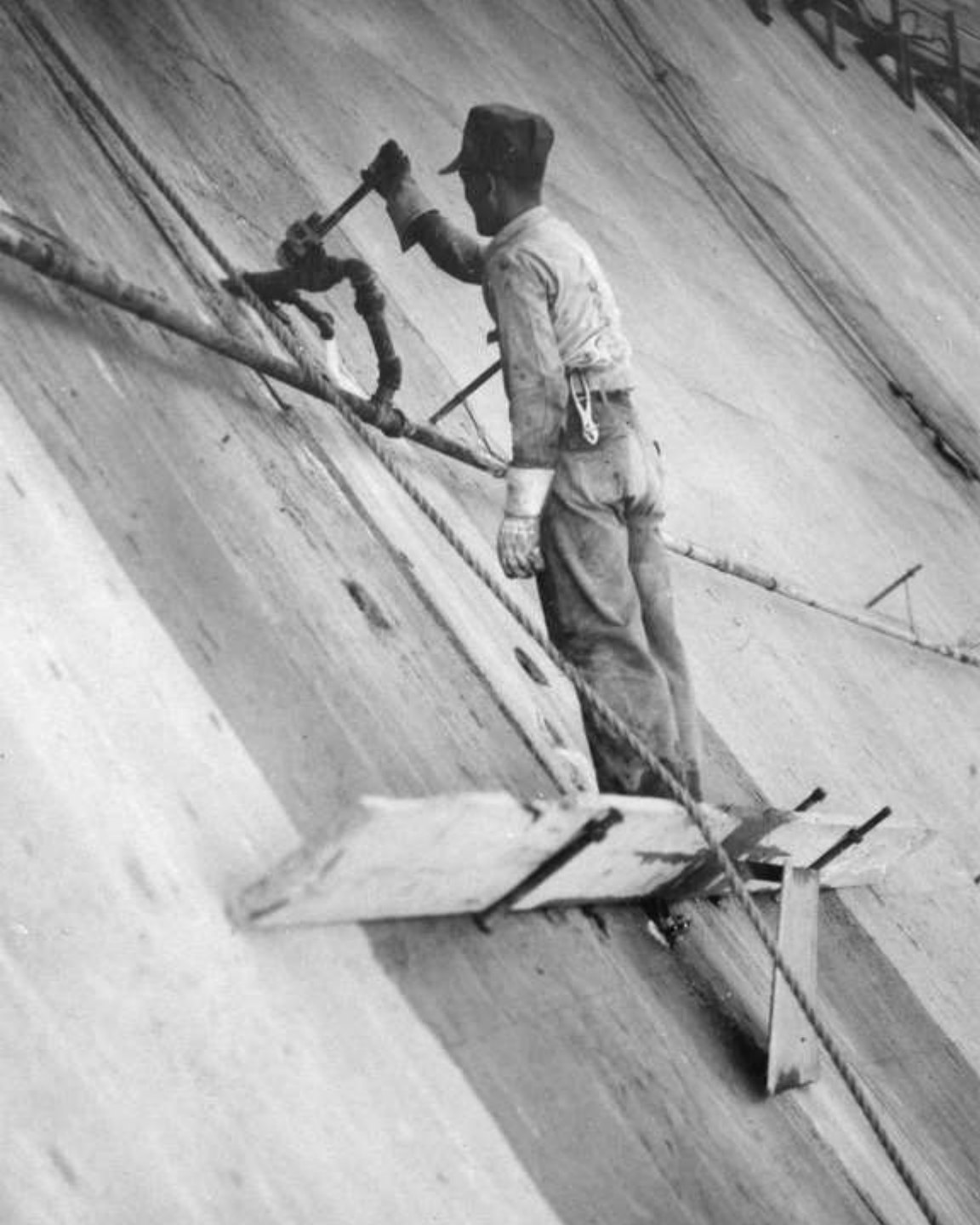
Left: valve connection at joint on lower (Elevation 1025) grout line (April 1935) Above: grout line showing catwalk and distribution line with valves (Elevation 1075; April 1935)
