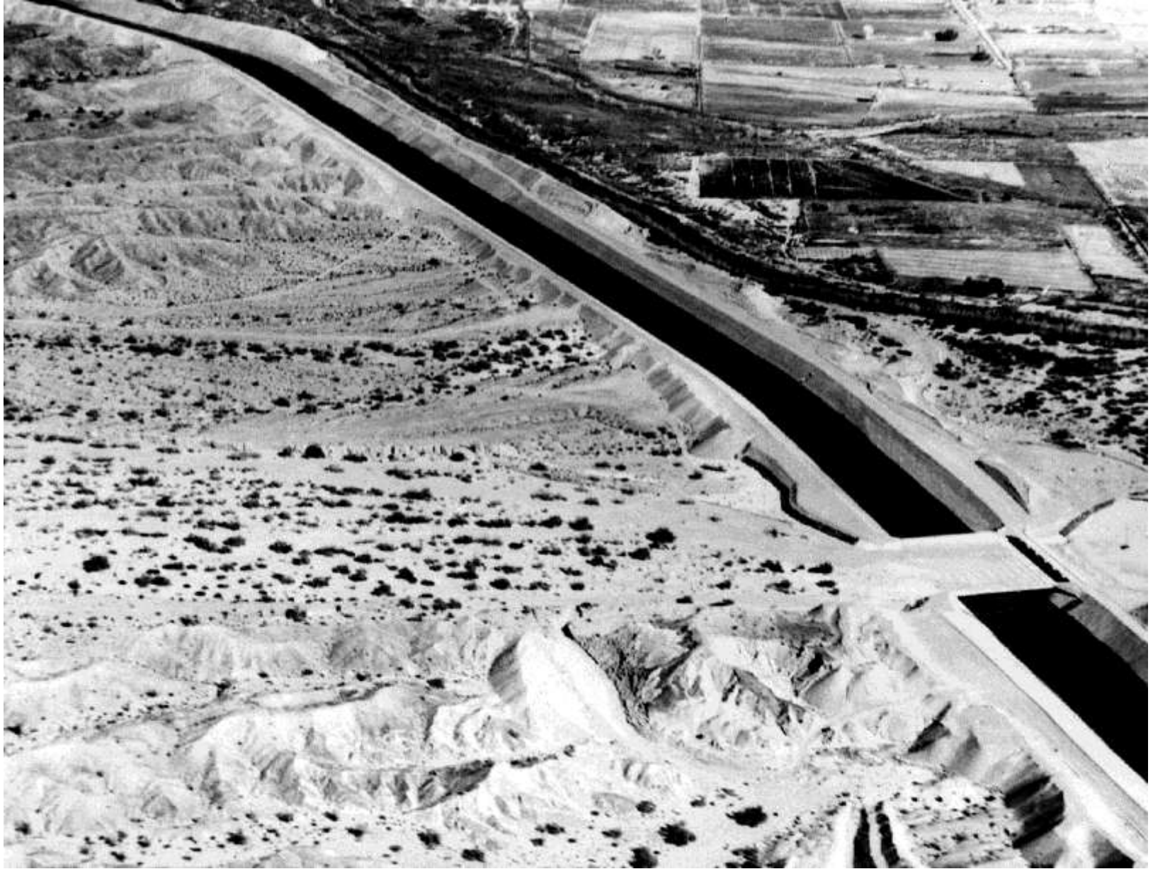
All-American Canal (Station 3330 to Station 3343; May 1940) 158
