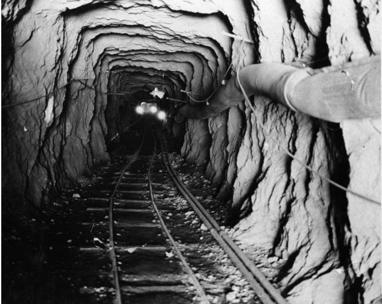
Arizona tunnel Adit (June 1931)
