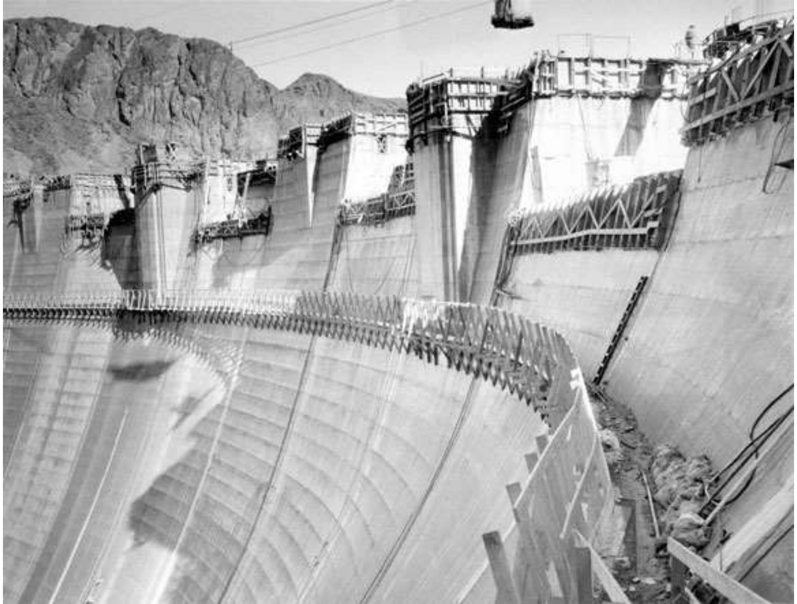
Downstream face of dam (top forms; January 1935)
