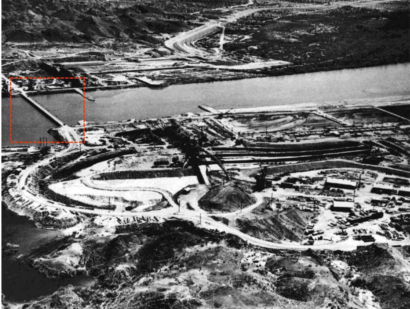
Imperial Dam , looking across the Colorado River toward the Arizona All-American Canal Headworks, with division walls of concrete sheet piling which separate the diversion channels to the Desilting works extending to the right (March 1937).
