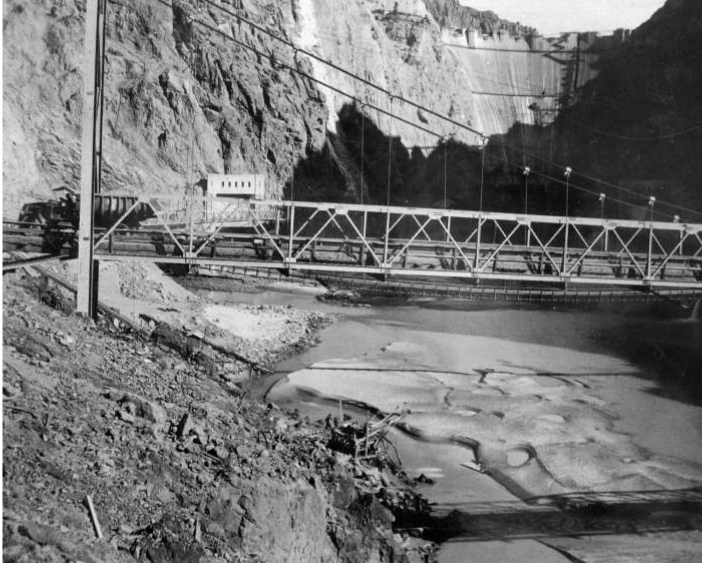
Riverbed immediately downstream from outlet of Diversion Tunnels during time when entire flow of river was being retained in reservoir (February 1935)
