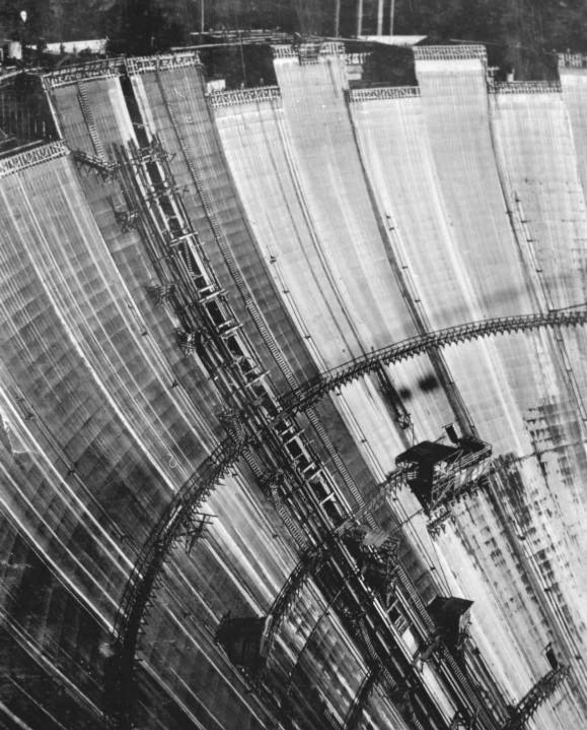
Mid-section of the downstream face of the dam showing eight-foot wide cooling system header slot and header pipes (top forms on dam at Elevation 1170; November 1934)
