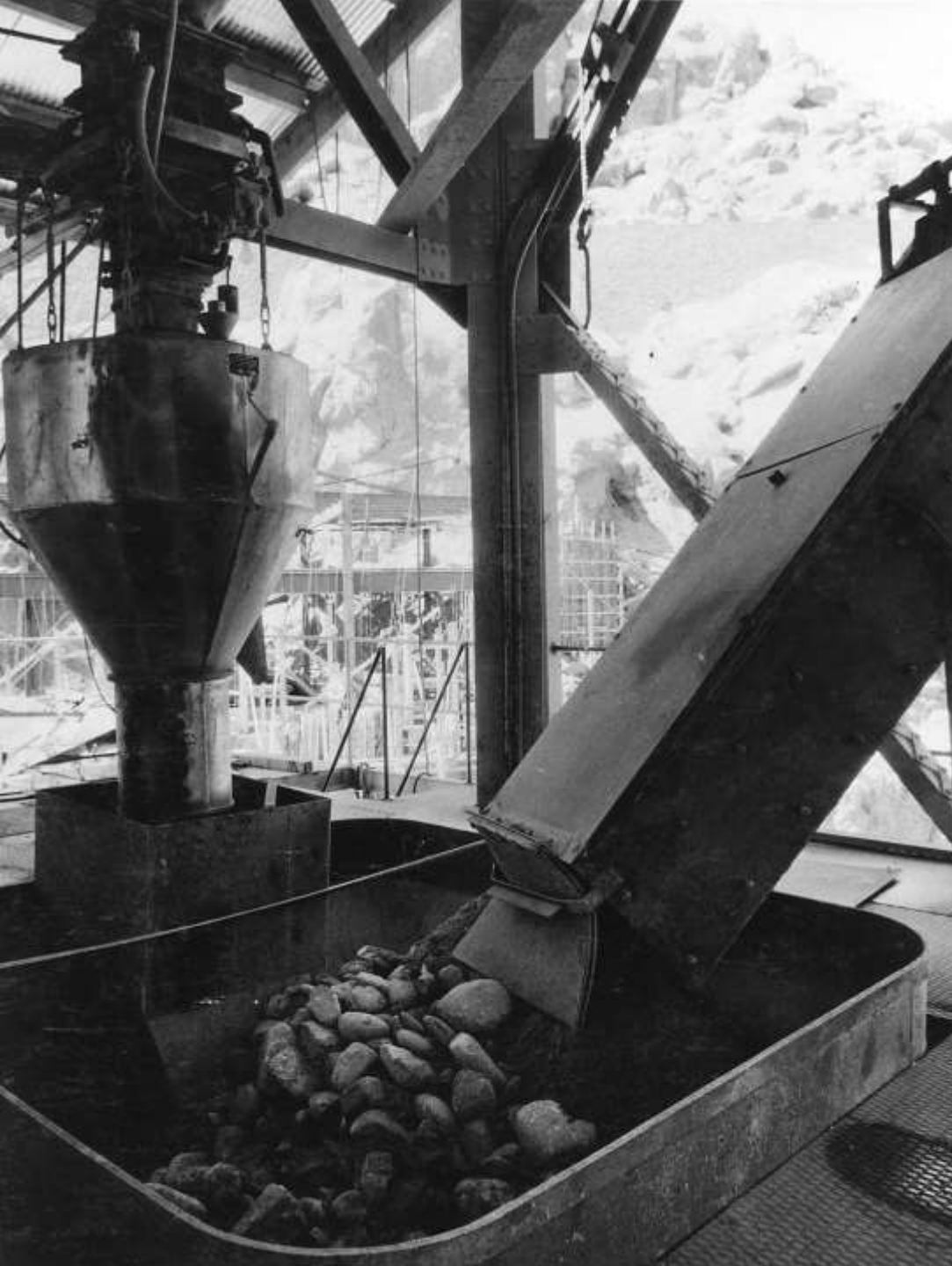
Aggregate delivery into mixer hopper at Six Companies' High-Level concrete mixing plant, (cement batcher and delivery seen at left; April 1933)
