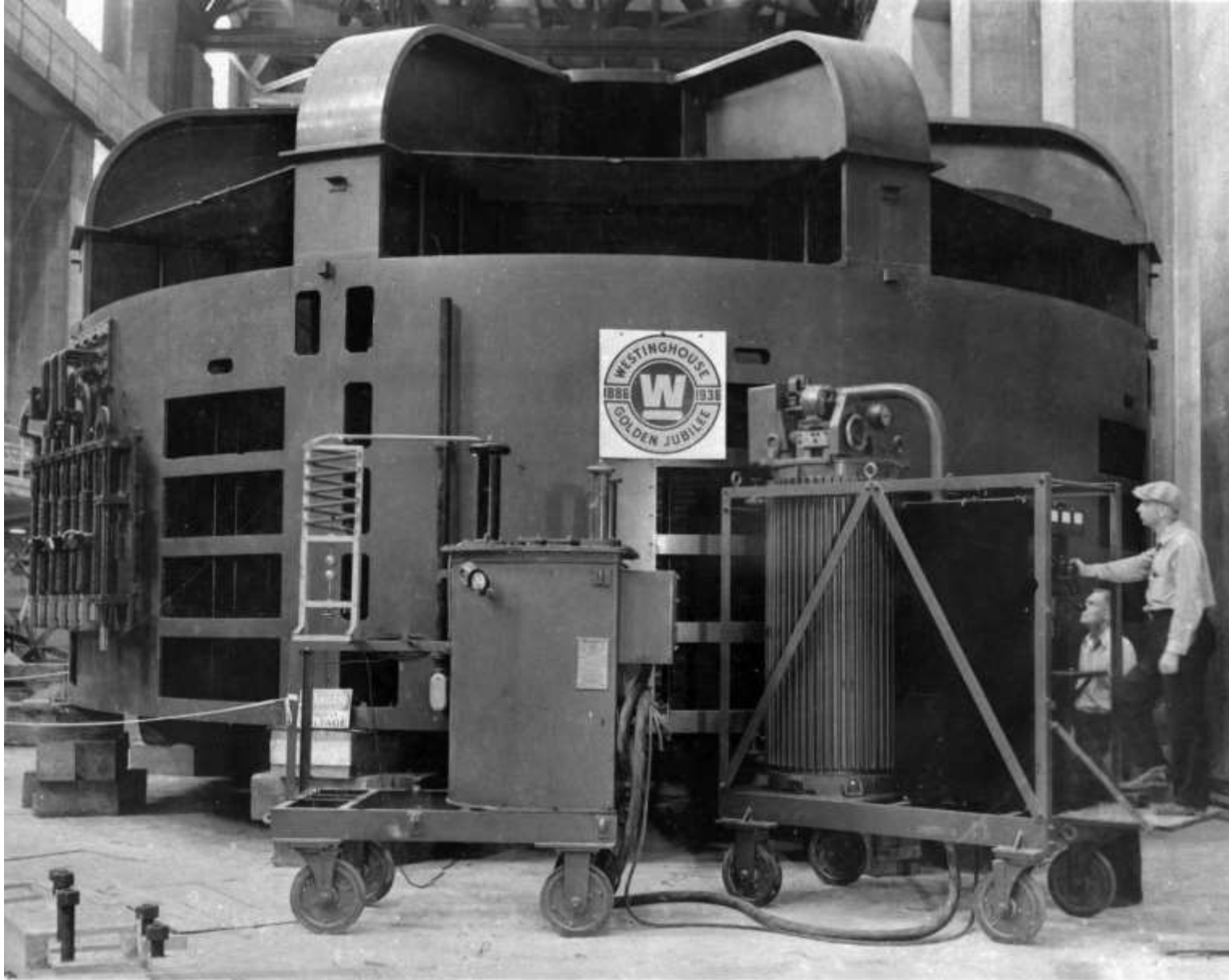
Westinghouse 82,500 kV-a stator shown with generator testing set (used to put artificial load on coils; June 1936)
