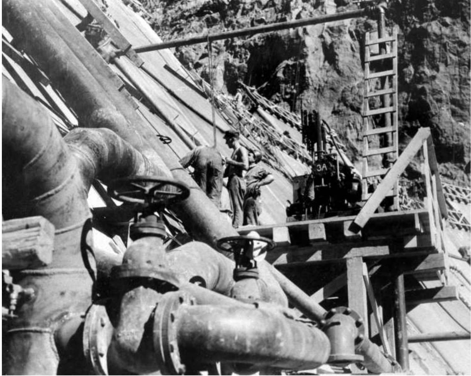
Booster pump and pipe connection into dam cooling system (at Elevation 795; April 1934)
