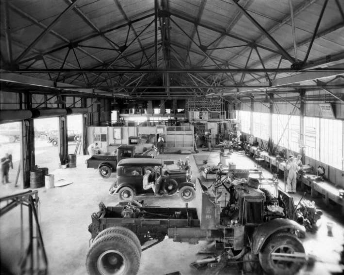
Interior view of Six Companies' garage and automobile repair shop in Boulder City. Complete facilities were installed for overhauling all classes of equipment (August 1932).
