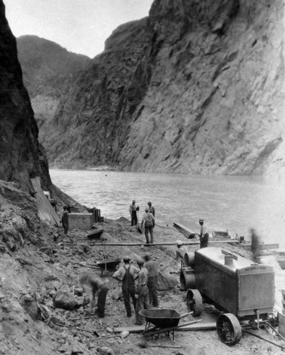
Leveling bar at Arizona abutment (for compressor plant) to drill Adits to Diversion Tunnel/s (April 1931)
