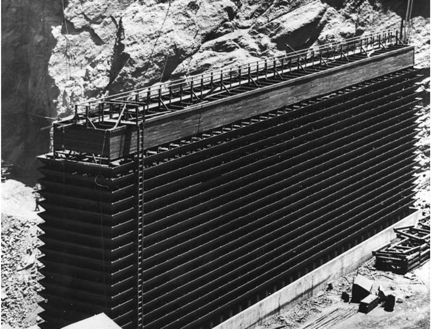
Evaporation Tower for concrete cooling system
