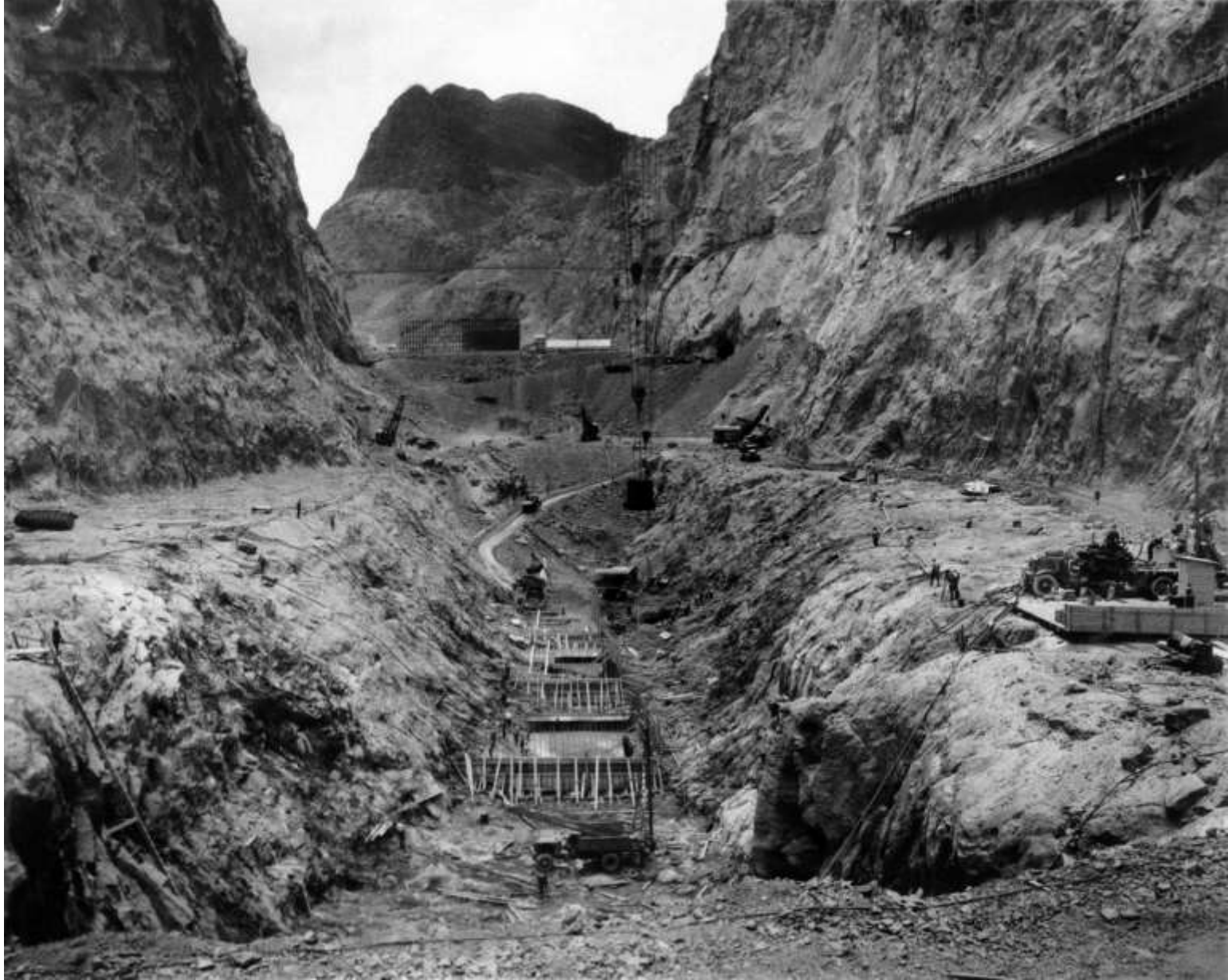
First forms for Hoover Dam (looking downstream; June 1933) 633
