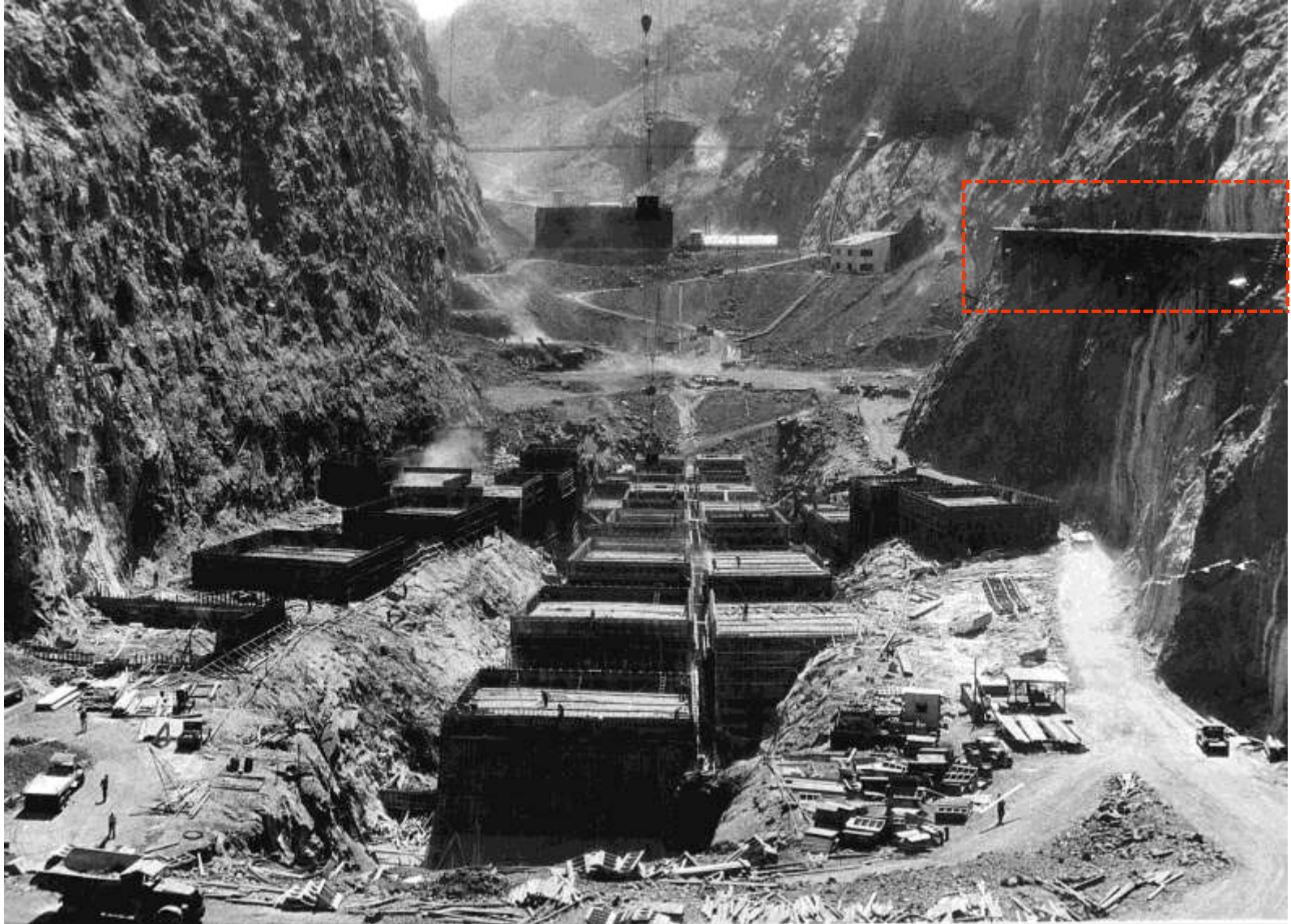
Looking downstream across dam construction (from upstream cofferdam). Trestle over which electric trains operated can be seen against the canyon wall (at right; July 1933).
