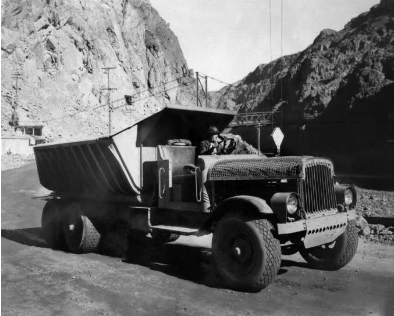
A Moreland truck of twelve cubic yards capacity, used in hauling muck from upper portals of the Diversion Tunnels. This truck has dual rear axle. (note the wire mesh protection over the hood and the protected headlights; January 1932).
