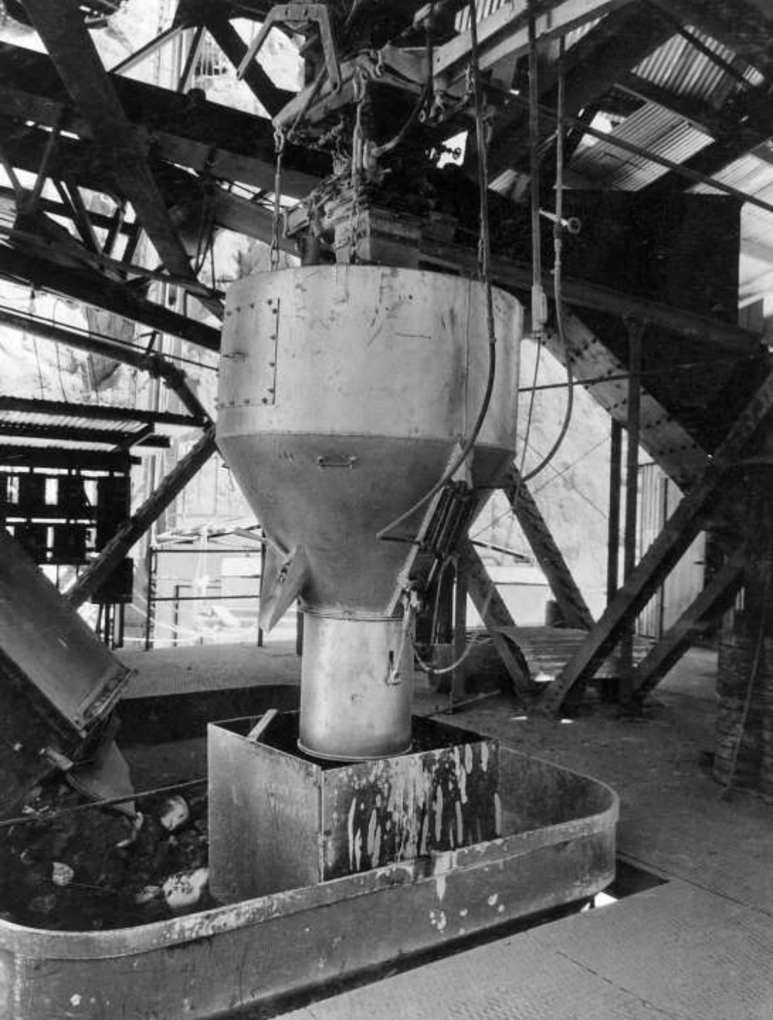
Cement batcher assembly over aggregate hopper at the Six Companies' High-Level concrete mixing plant (feed mechanism and lever arm connection to scales seen at top; April 1933)
