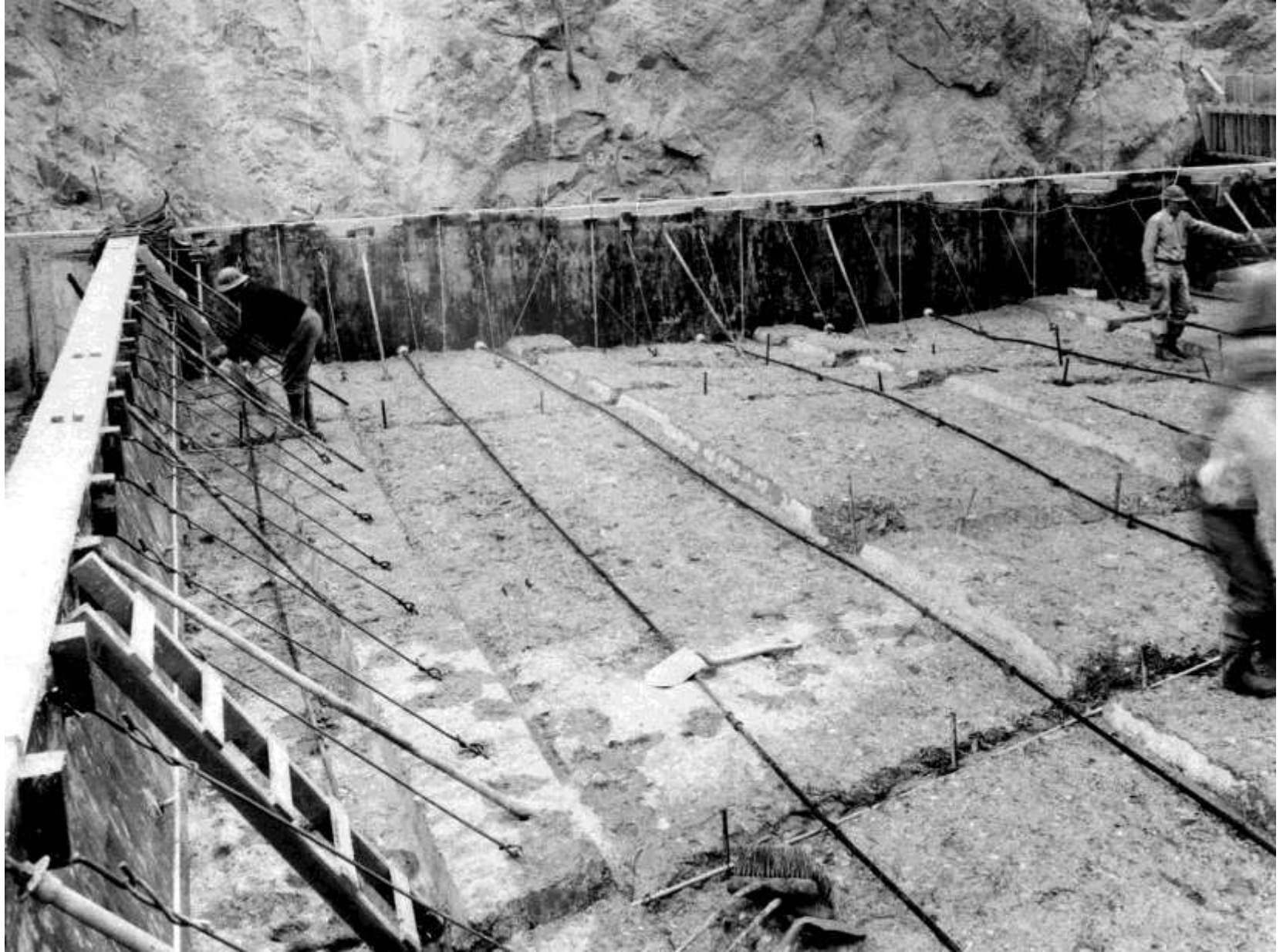
Close up of cooling pipe layout in Panel H3 (February 1934) 610
