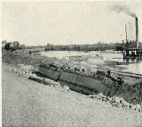
Controlled water disposal prevents floods
