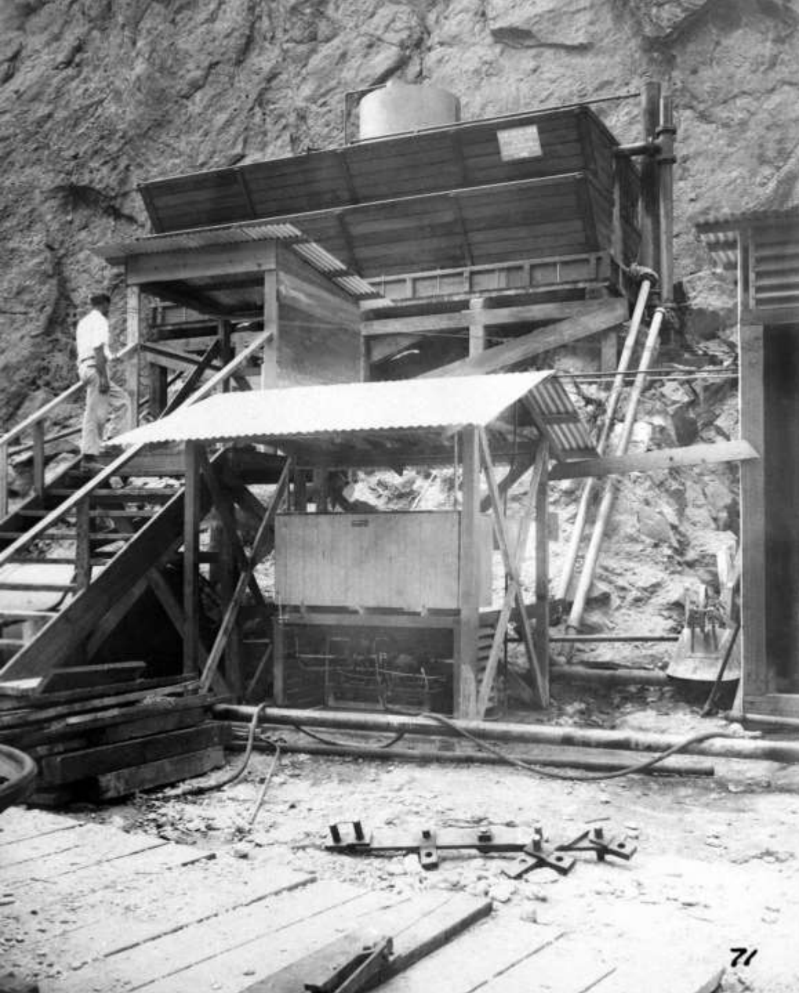
Frigidaire drinking water and water cooling plant (at compressor No. 2, Arizona side; August 1931)
