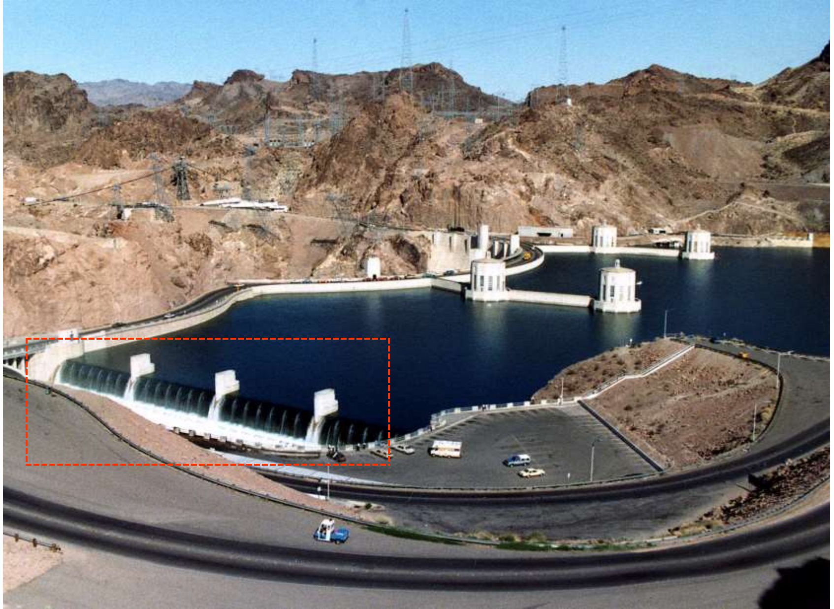
Westerly view of Arizona Spillway
