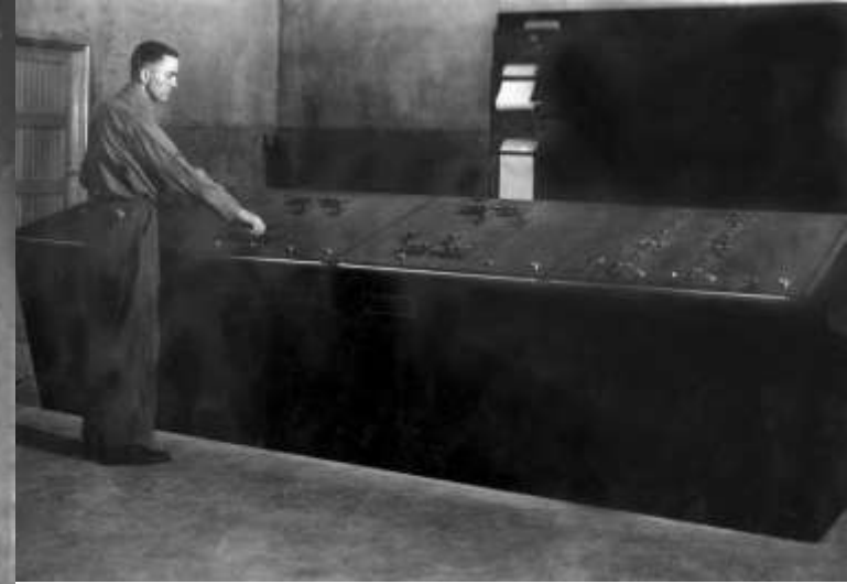
Left : recording instruments located on auxiliary boards in the Main Control Room (central portion of the Powerhouse; October 1936) Above : supervisory control board furnished by the City of Los Angeles. Located in the Main Control Room (central portion of the Powerhouse; Oct. 1936).
