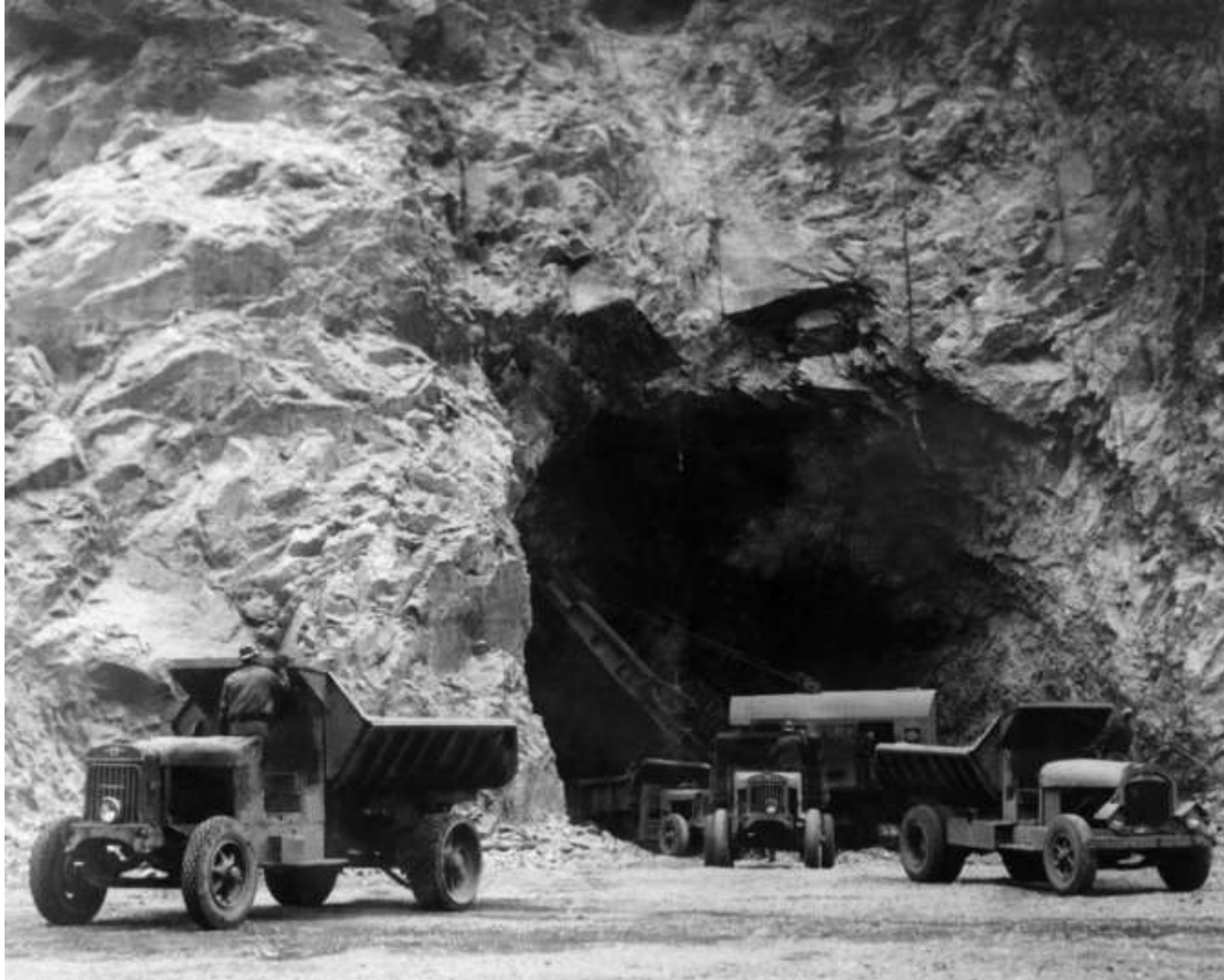
An International truck with capacity of seven cubic yards (shown on the left), with approved type of “bath-tub” body. Two International trucks in the background have older type of bodies. White truck with seven cubic yard body is shown on right (January 1932).
