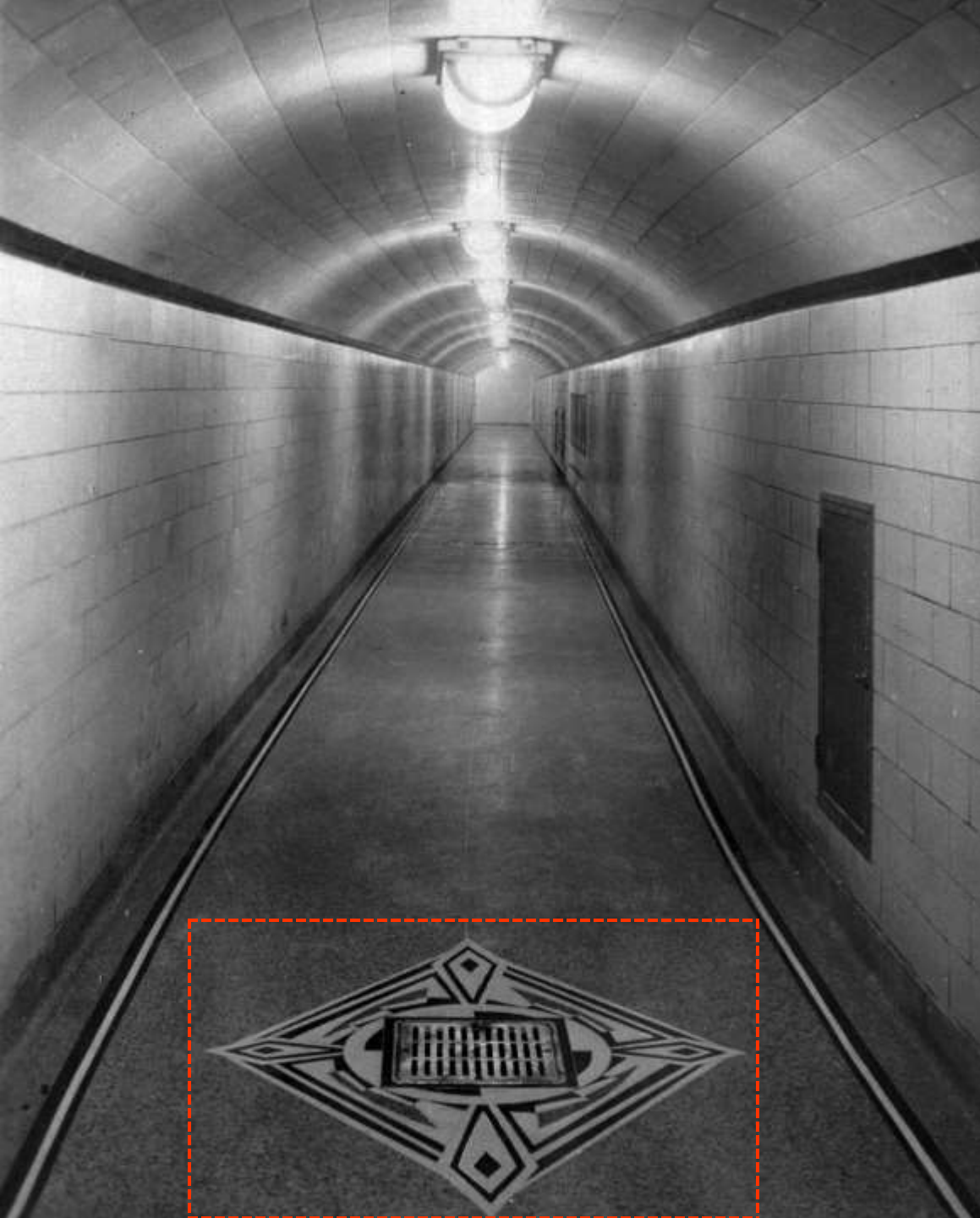
Gallery (at Elevation 705) inside the dam, Arizona side, (leading from the Elevator Lobby to the powerhouse). Note the Native-American decorative floor inlay (by Allen Tupper True; November 1936)
