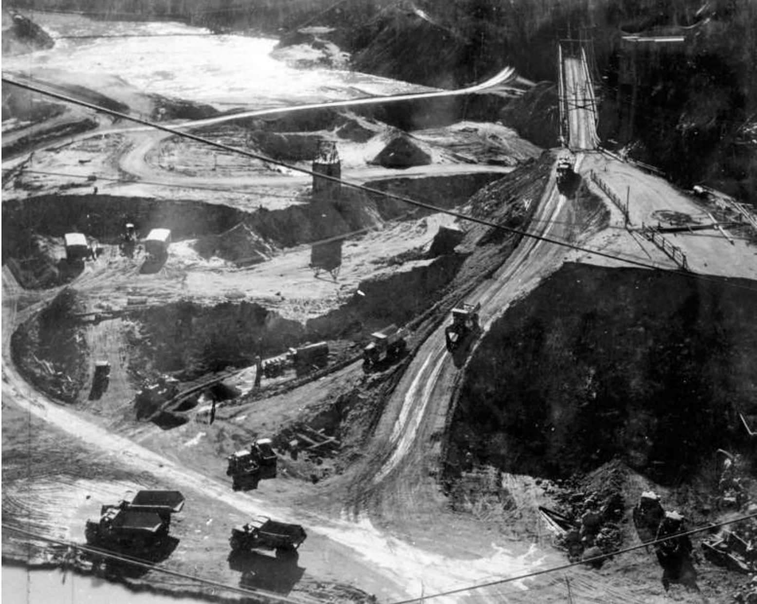
Power shovels and trucks removing Downstream Cofferdam (January 1935)
