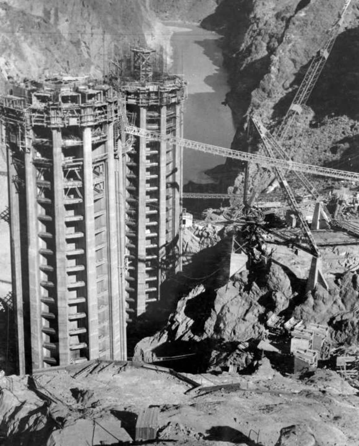
View looking upstream along Arizona canyon rim (showing the Arizona Intake Towers; November 1934)
