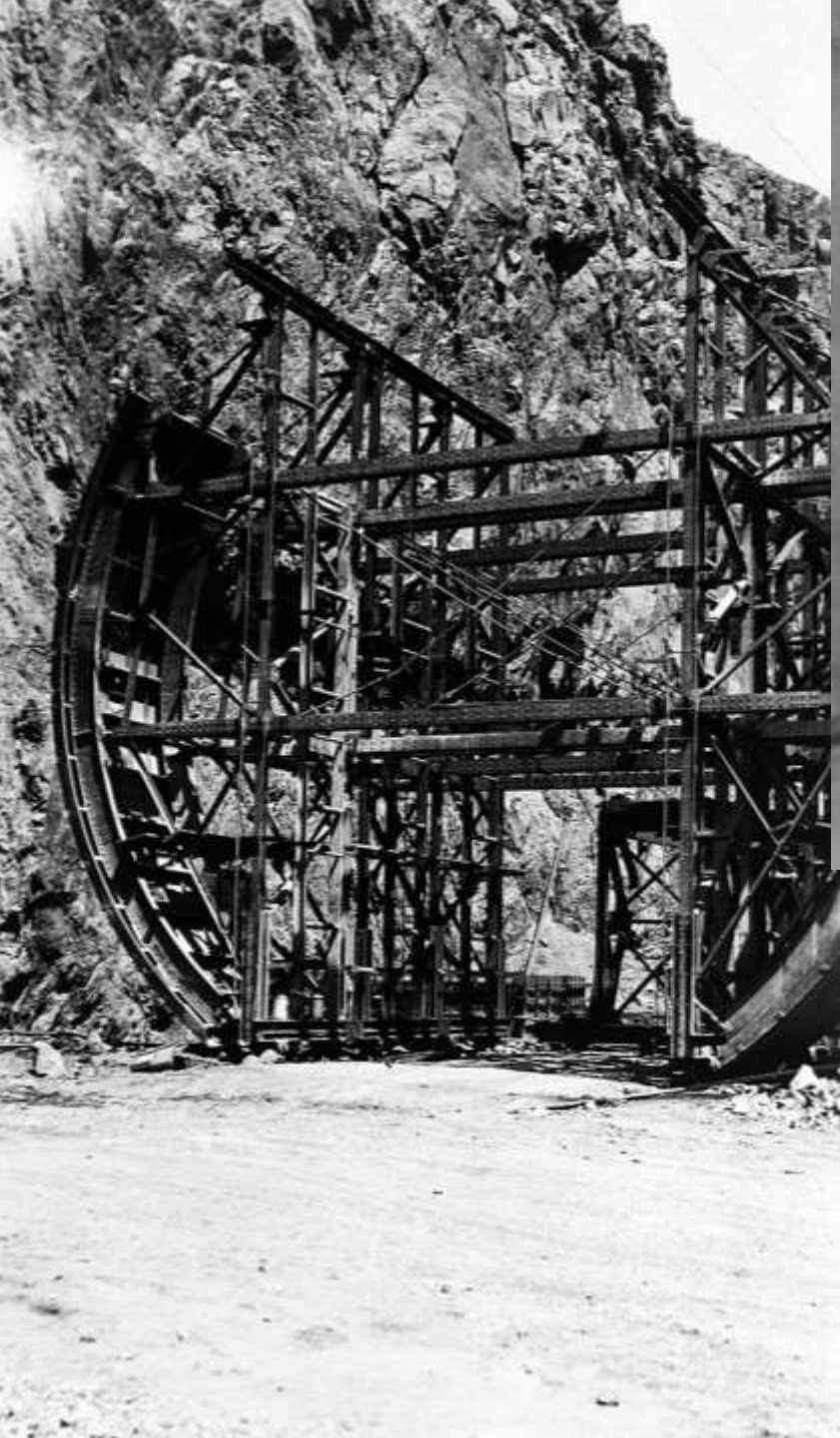
Left : Pressure Grouting Jumbo Frame Above : access Adit to Diversion Tunnel Number One (upstream tunnel plug demonstrating leakage prior to grouting; April 1935)
