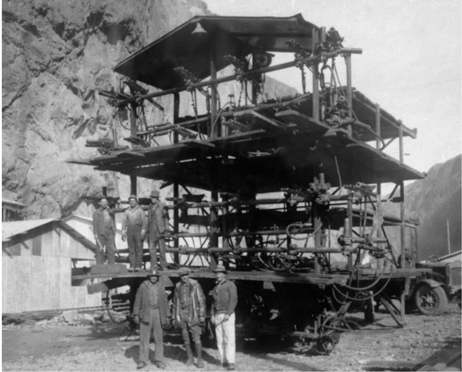
View of drilling Jumbo taken outside the Diversion Tunnels. It was welded steel construction, mounted on a truck chassis (December 1931).
