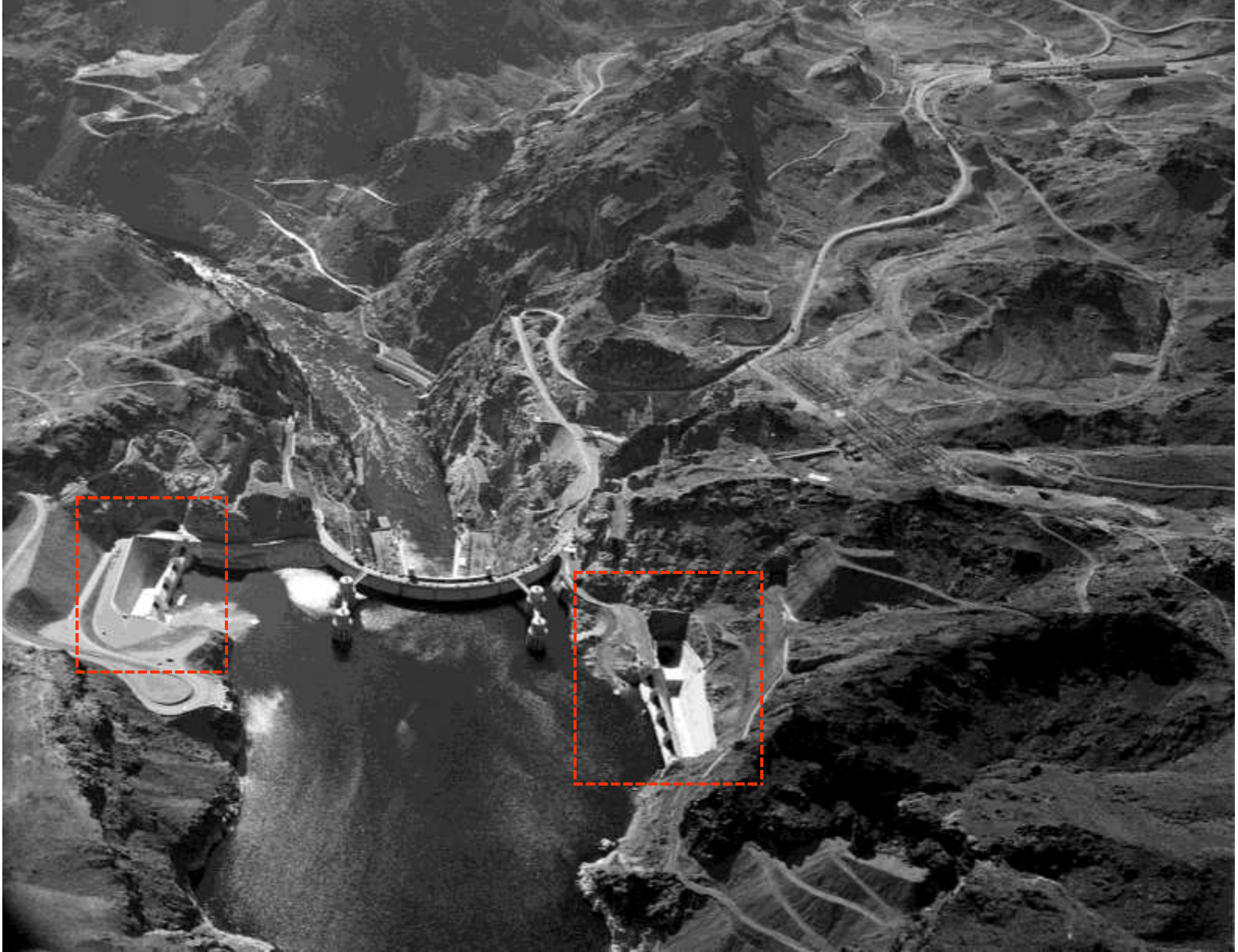
Aerial view of Hoover Dam showing Intake Towers, Spillways and roadways (October 1947)
