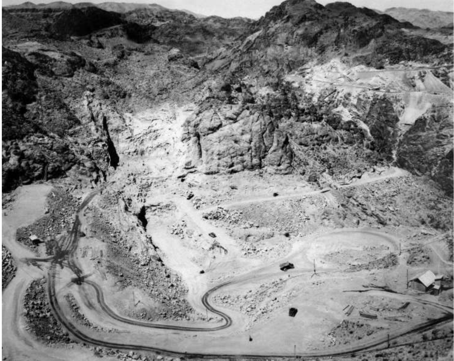
Six Companies constructed muck roads and spoil dumps (June 1932)
