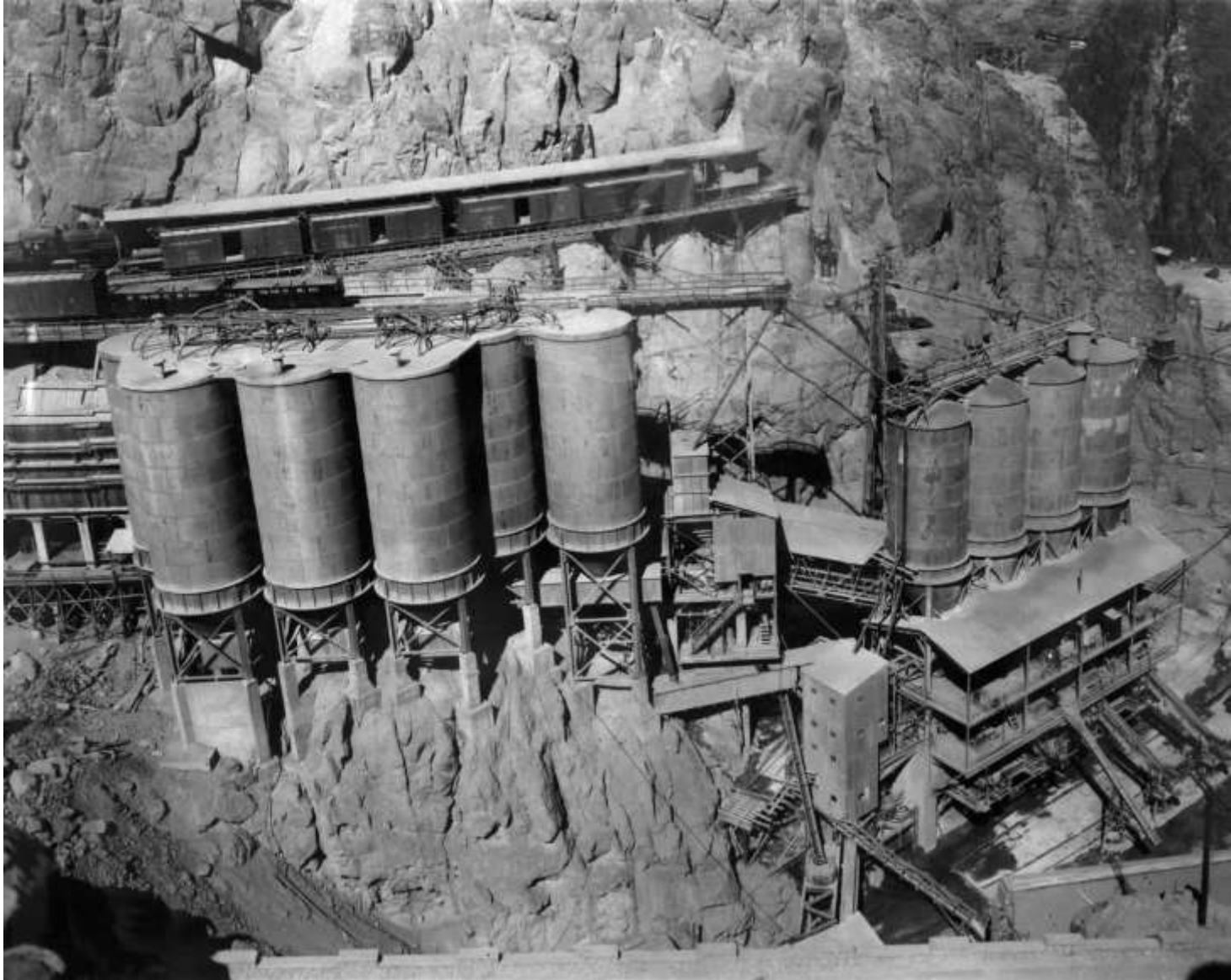
Hi-Mix and cement blending plants (with unloading track and aggregate bins above; April 1934)
