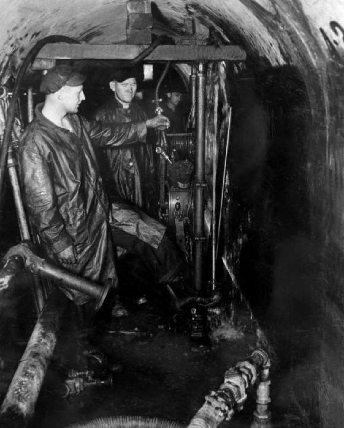
Diamond drill crew working on center hole A-4 (located at the approximate center of the inner gorge in the 553 gallery; June 1939)
