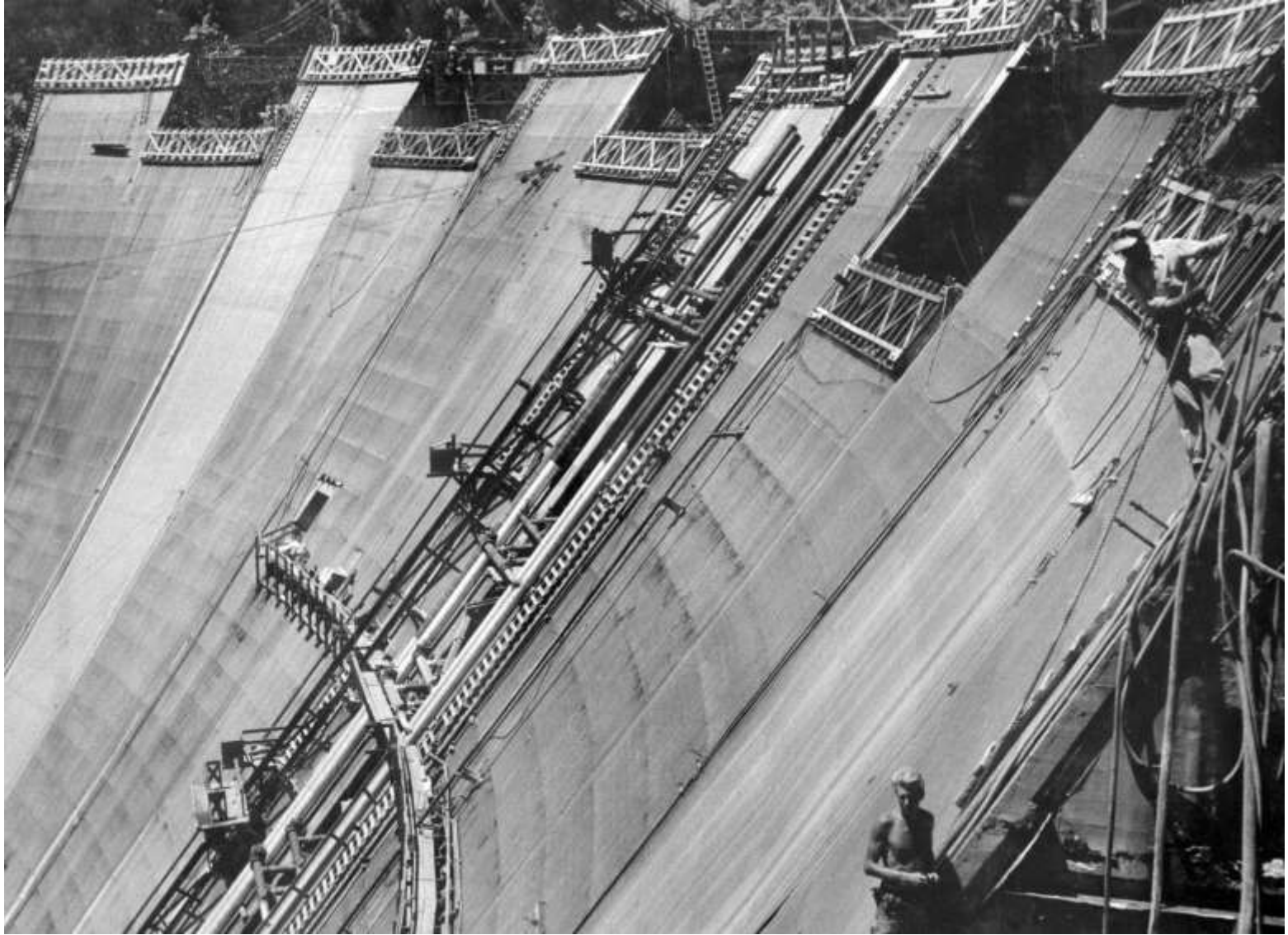
Looking across the downstream face of the dam at top of forms (toward Nevada side). Cooling system header pipes seen in middle (July 1934).
