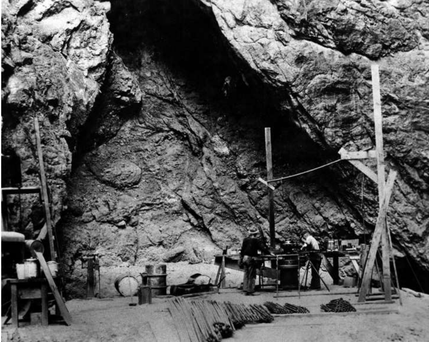
Halfway between the upper end of the diversion tunnels and the dam site, Six Companies operated a drill sharpening shop (on the Arizona side) in a large cave which afforded a cool spot for such work (May 1931)
