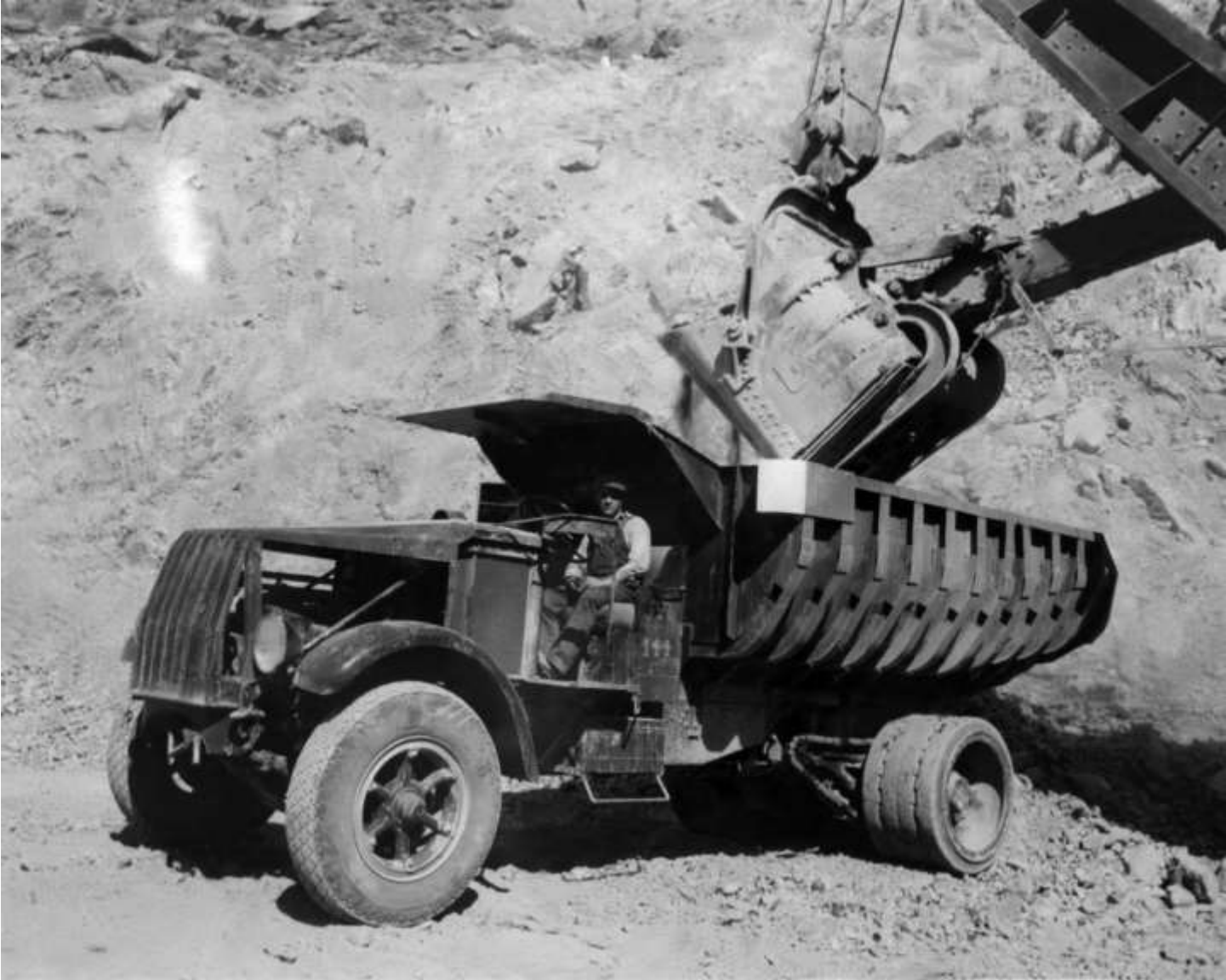
Mack truck with fourteen cubic yard body being loaded at the Nevada Spillway cut. Five similar trucks were being used on this operation (March 1932).
