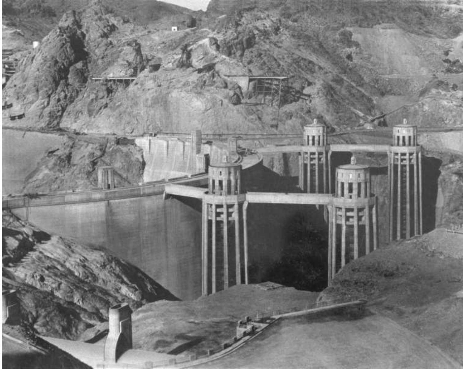
View looking across dam and Intake Towers (from saddle on Arizona Spillway; December 1935)
