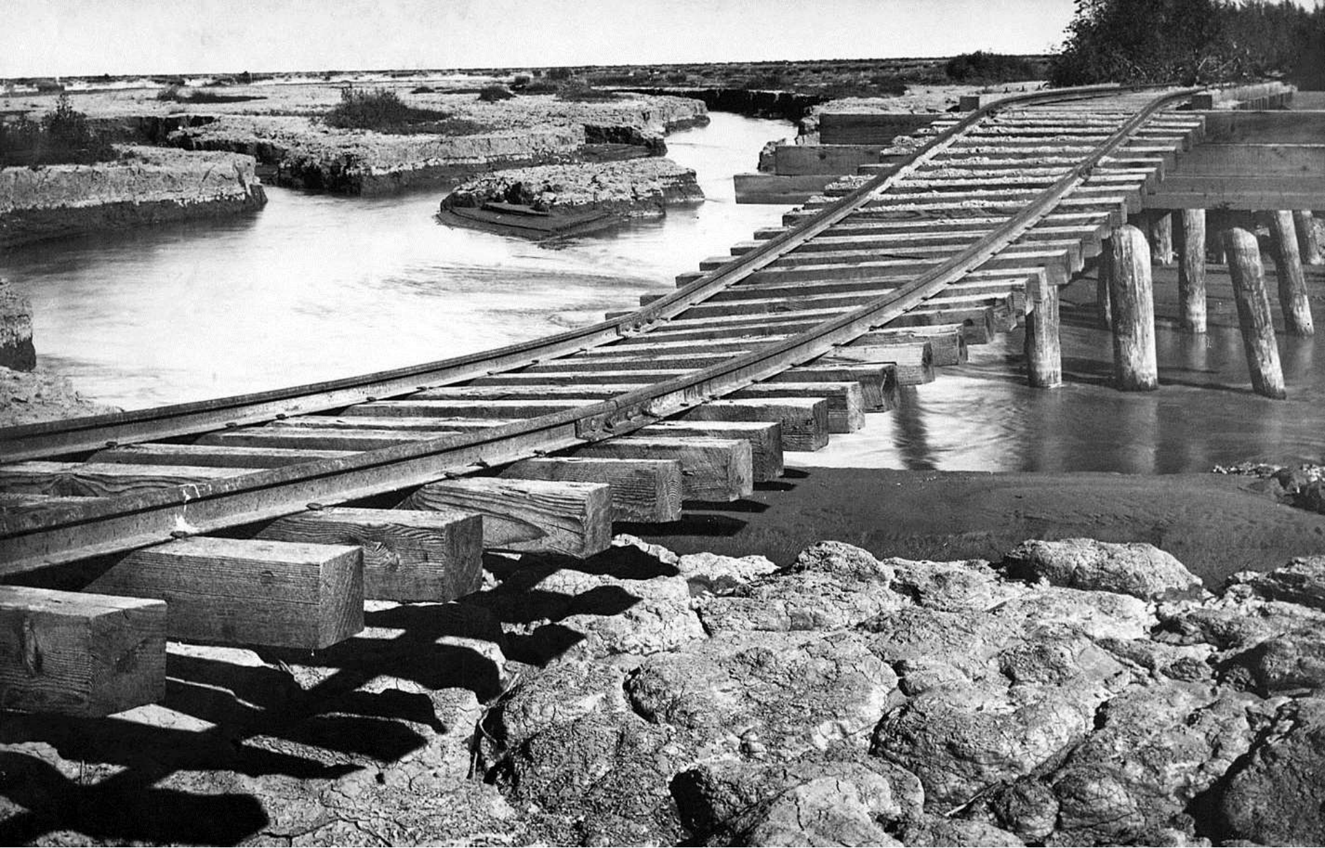
View shows where the Southern Pacific railroad tracks were cut into and washed out (September 1906)
