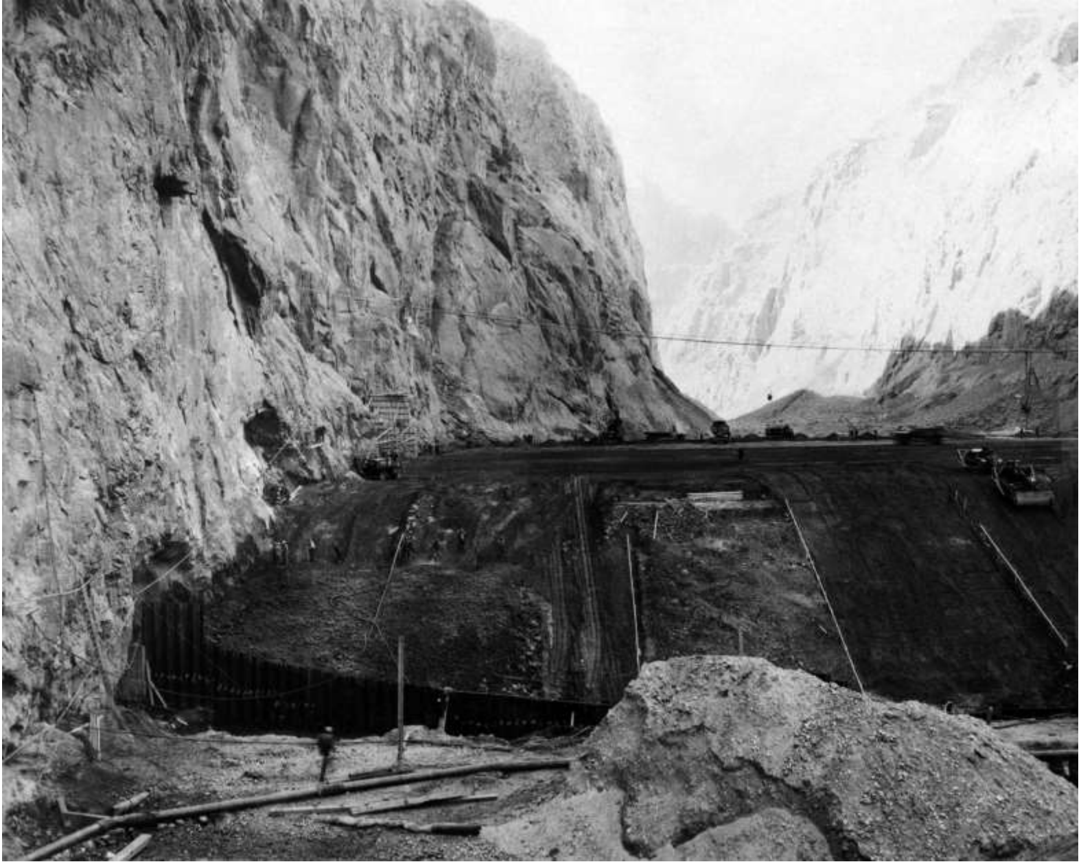
Upstream Cofferdam (looking downstream; Dec. 1932)
