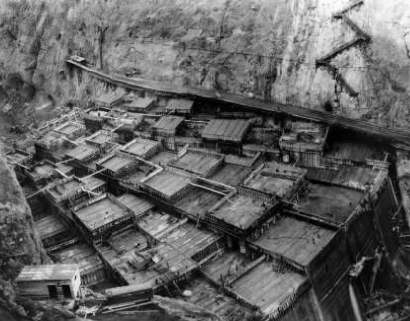
Top: upstream face of dam (as seen from upstream cofferdam). Top forms at Elevation 715 (December 1933). Left: Close-up of Hoover Dam. The top blocks are at Elevation 715 (November 1933).
