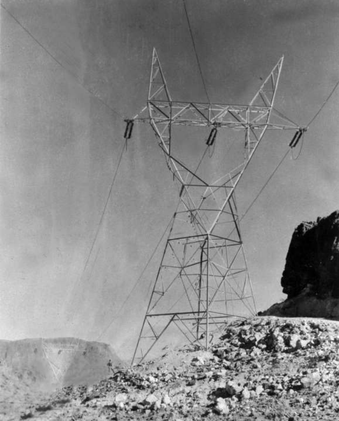
One of many transmission towers comprising the City of Los Angeles ' 287,500 volt transmission line
