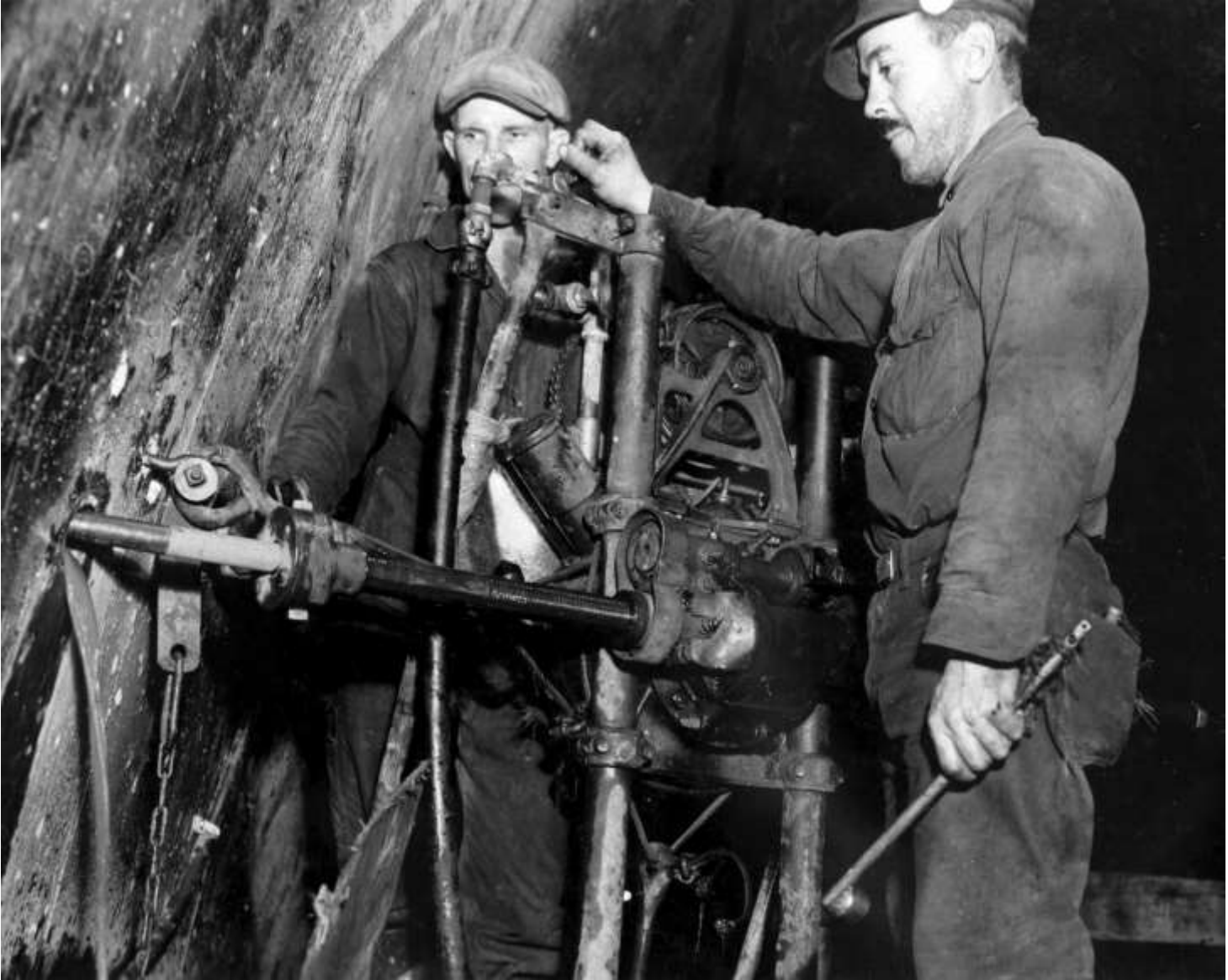
Drilling grout hole (December 1940). Drill rods were in ten-foot sections. These sections could be put together, making possible drilling depths of plus 1K-feet.
