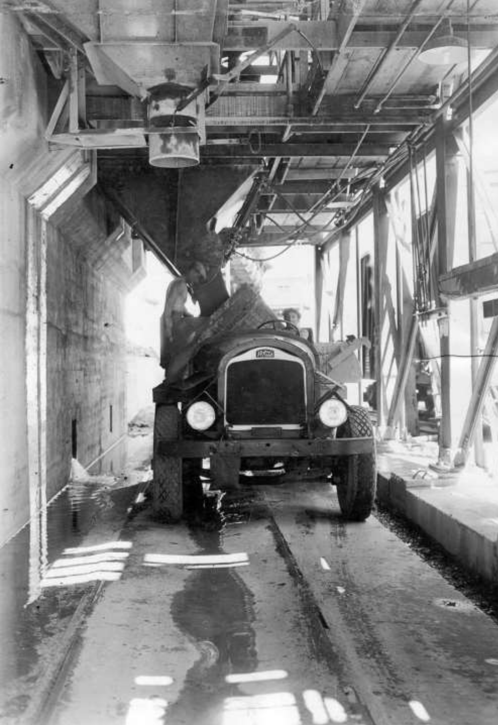
Left: loading concrete into two cubic yard bottom dump buckets at Six Companies' low level concrete mixing plant. Buckets were hauled (two to a truck) into Diversion Tunnels where they were handled by crane into position over invert forms (April 1932) Above: truck loaded with concrete entering the upper portal of Diversion Tunnel No. 2 (through opening left in Cofferdam; April 1932)
