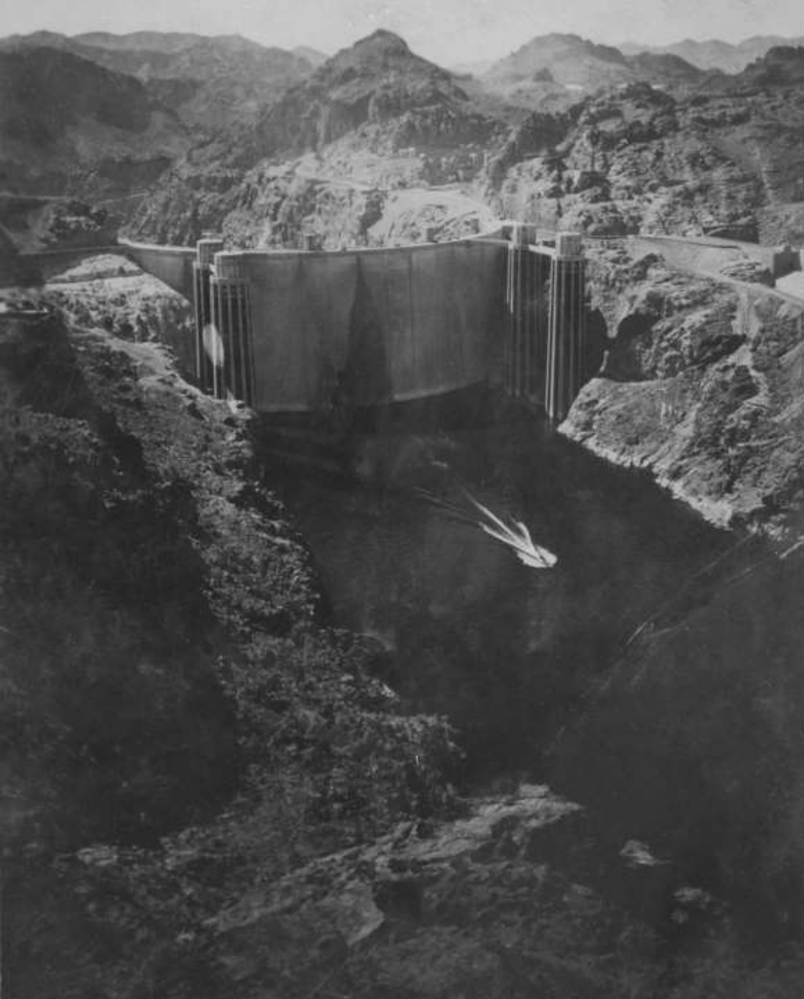
View looking downstream of the reservoir, Intake Towers, and Spillways (March 1936). The reservoir surface was near its lowest stage preceding the spring runoff of 1936
