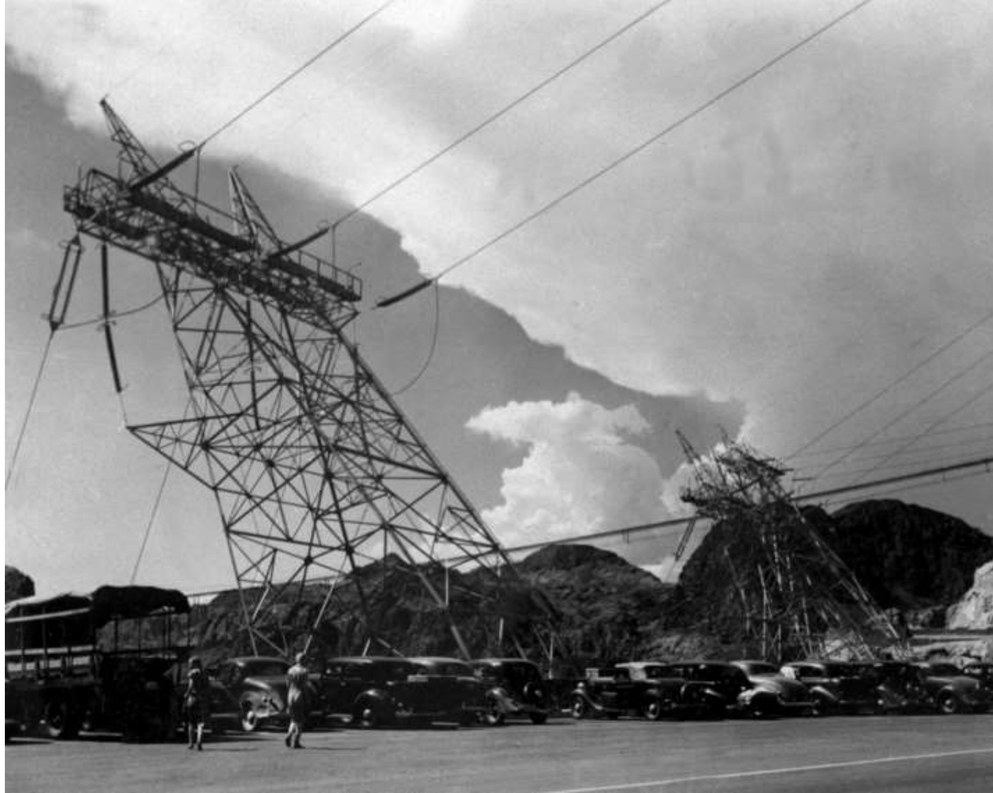
Leaning towers on the Nevada rim of Black Canyon that carry the power lines from the roof of the Nevada Powerhouse up and over the highway to the switchyards above (August 1939)
