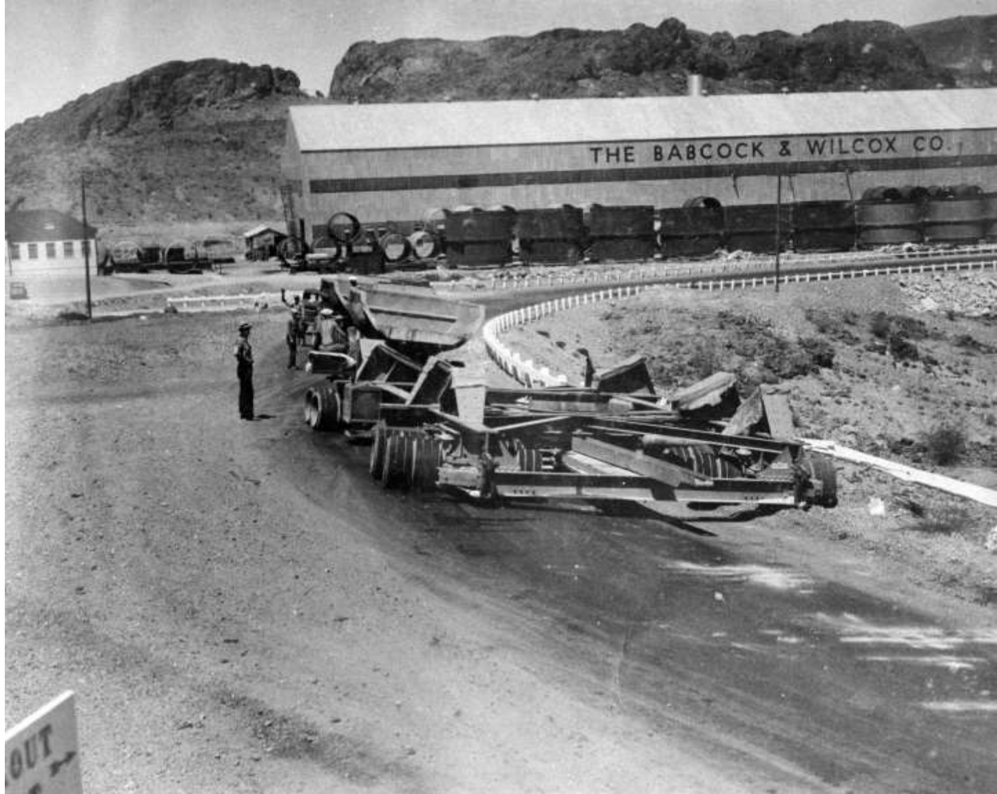
The 200-ton capacity La Crosse trailer used in transporting pipe sections from plant to dam slips on super-elevated roadbed between Boulder City and the Babcock and Wilcox Company plant (July 1934)
