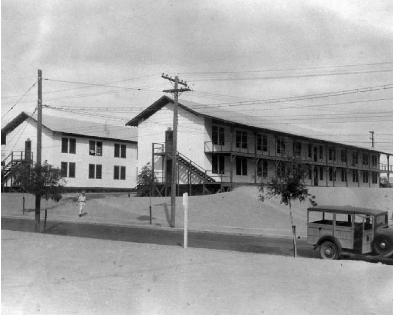
Typical dormitory housing employees of Six Companies. Each dormitory of this type (of which there were eight) housed 172 men in separate rooms, all of which were equipped with an air cooling system (October 1933).
