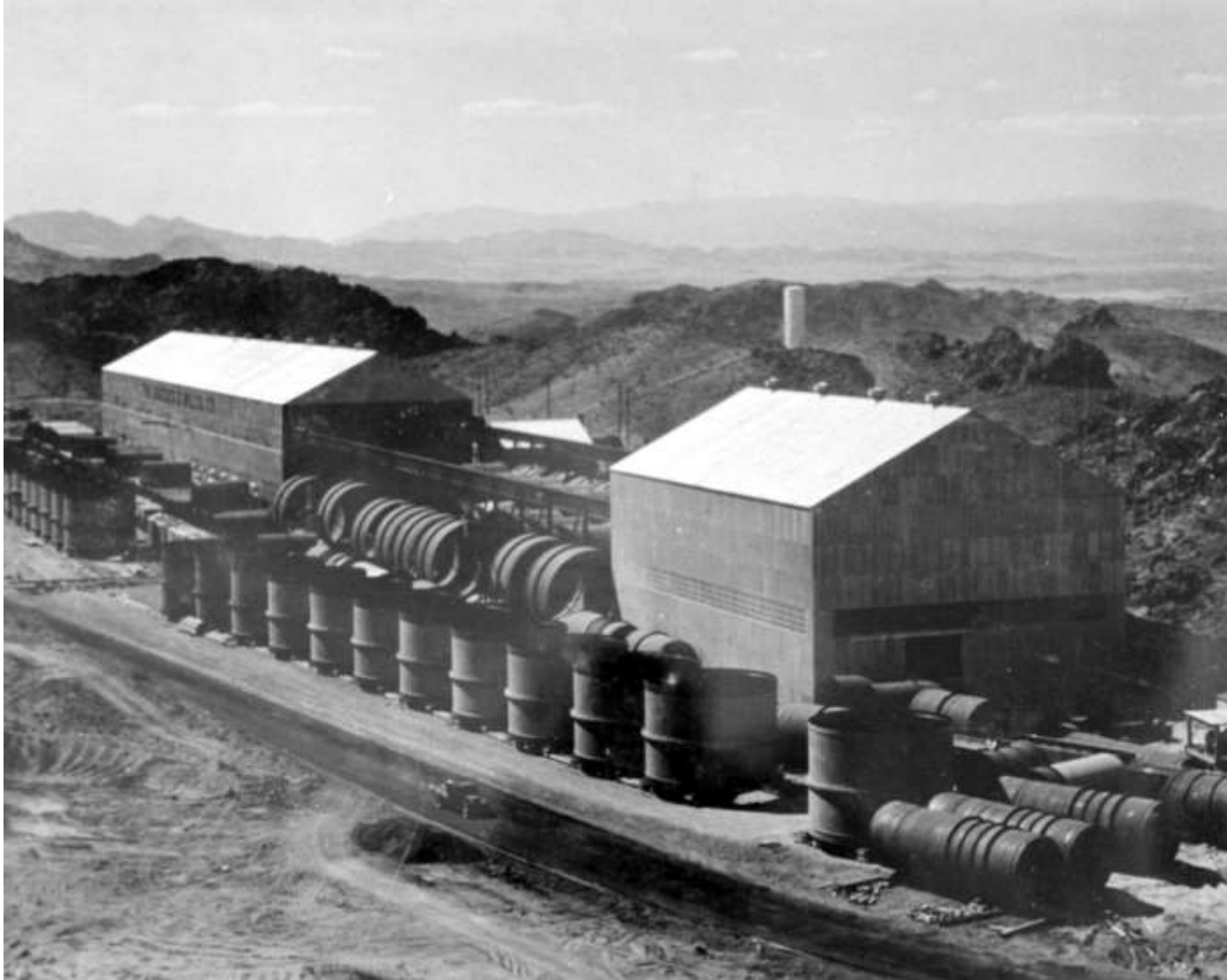
Plant of the Babcock and Wilcox Co. with view showing thirty-foot diameter penstock pipe awaiting transportation to the dam (July 1934)
