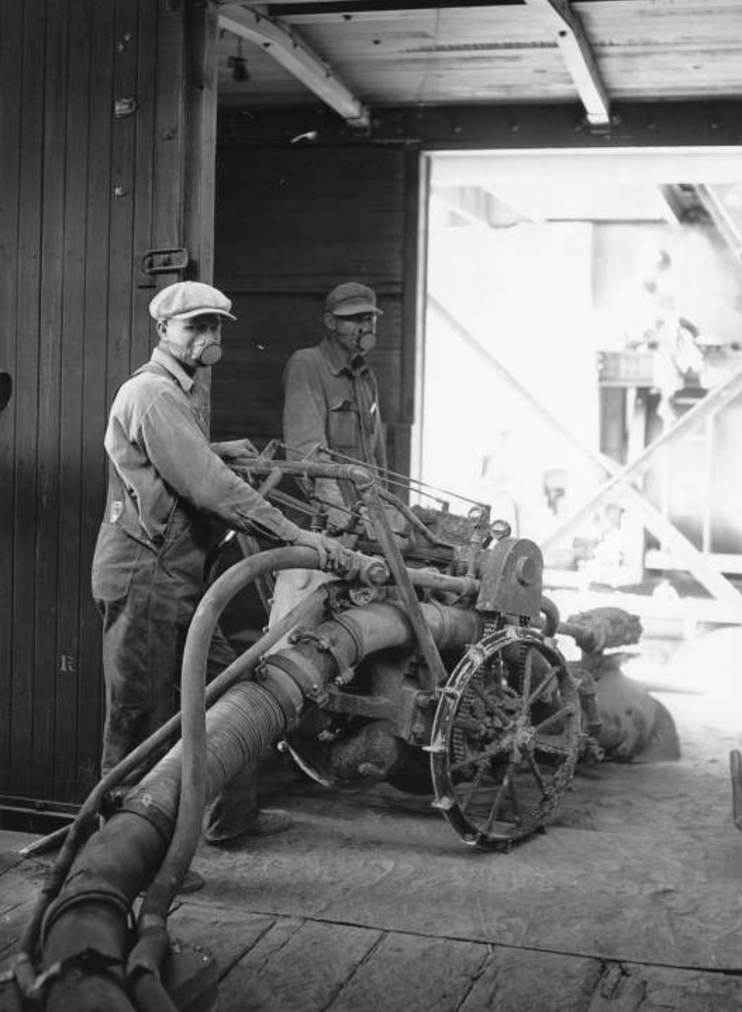
Left: unloading cement at Six Companies' Low-Level mixing plant (note that workmen are wearing respirators; May 1932) Above: agitator truck used to haul concrete from Low-Level concrete mixing plant to forms (March 1932)
