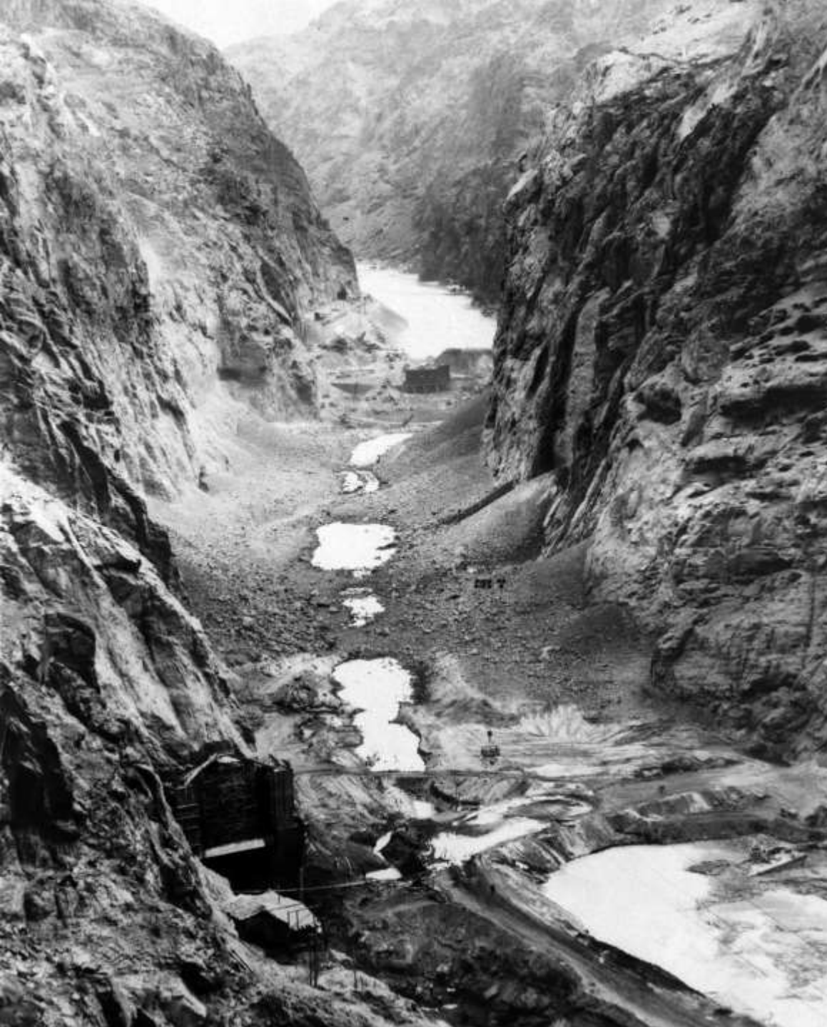
Looking upstream in Black Canyon (from lower portals) showing Lower Cofferdam site and general conditions after diversion of the Colorado River (November 1932)
