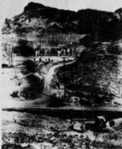
CONSTRUCTION STARTED FOR YARDS FOR METROPOLITAN AND SOUTHERN CALIFORNIA EDISON COMPANY
