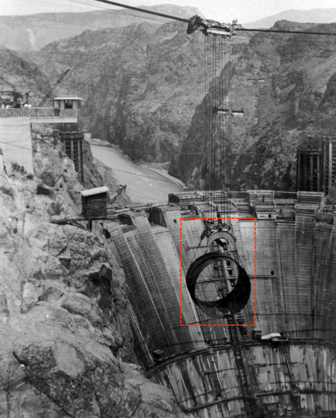
Section of thirty-foot diameter Penstock pipe being transported to tunnel via 150-ton cableway (1934)
