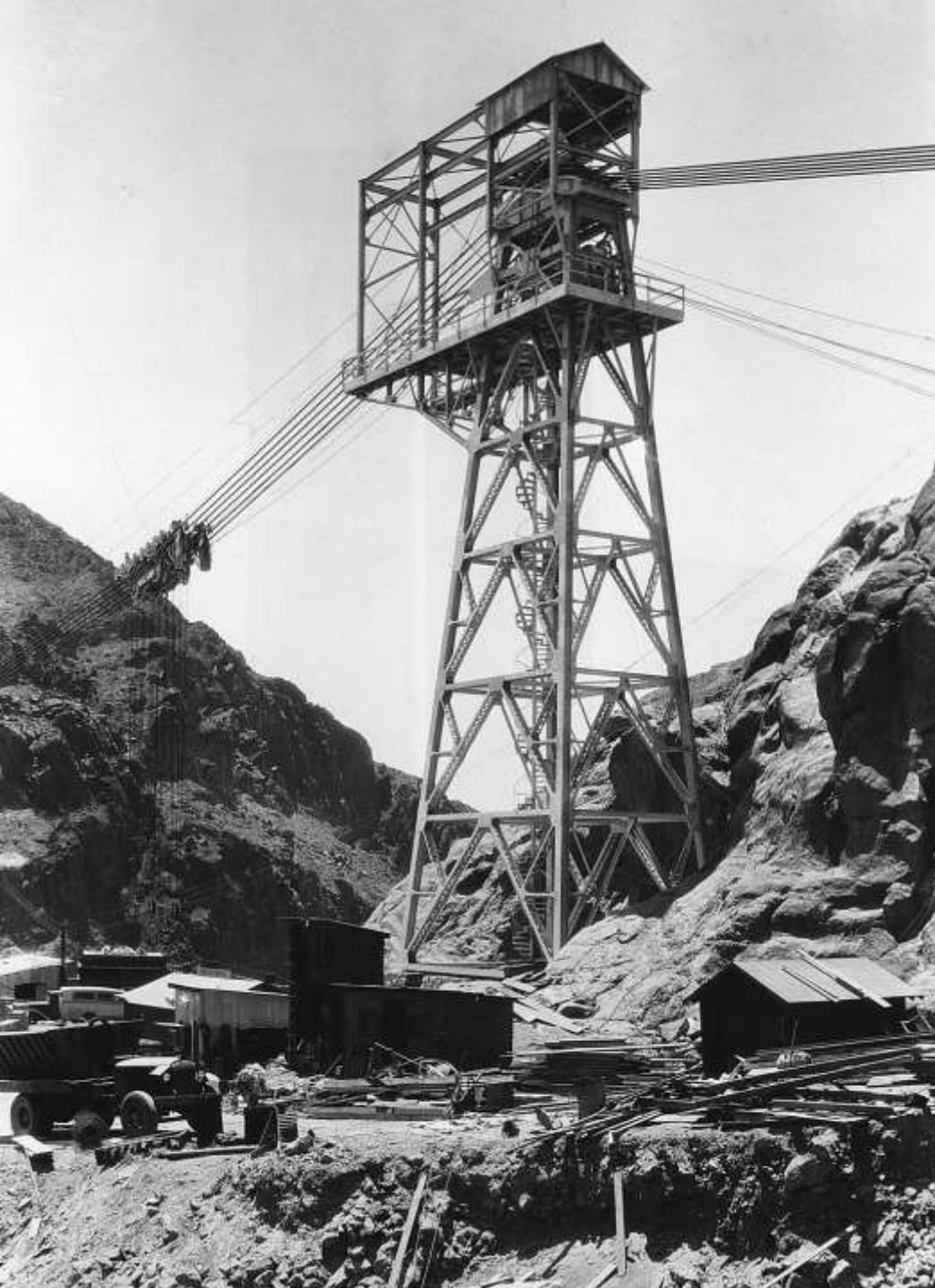
Head-tower of permanent 150-ton cableway (June 1933)
