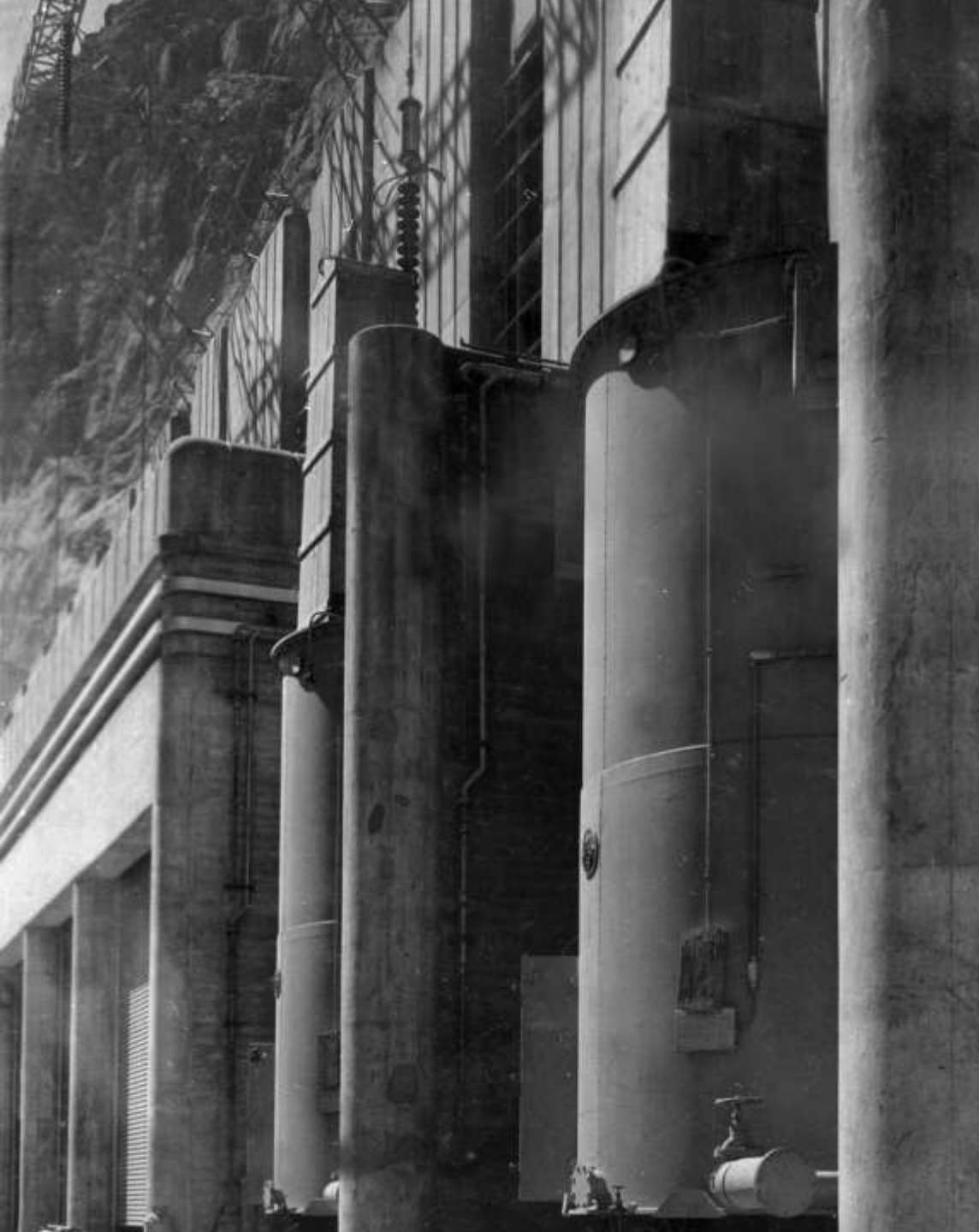
View/s looking downstream of the transformer platform (Nevada wing of the Powerhouse) showing 55K Kva transformers (Sept. 1936)
