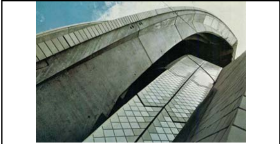
During construction, rib segments were stressed via nine steel cables (running from the bottom rib segment to the top rib segment). Once all segments of a rib were in place, up to twenty-one additional cables were stressed in three locations from the pedestal to the crown. Additional cables ran horizontally between ribs. On January 17 th 1967, the last of 2,194 rib segments went into its position at the top of the major hall. 565
