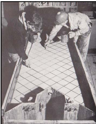
Sealing the clean grooves between tiles (face-side) with epoxy after overnight steam-curing has melted away the animal fat
