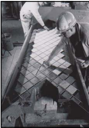
Laying the tiles in Tile Lid
