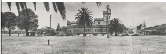
A VIEW FROM WASHINGTON STREET SHOWING APPROXIMATE AND EXISTING BUILDINGS
