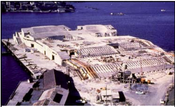
The Podium covers 4.5 acres measuring 600-feet long by 312-feet wide (at its southern end). The highest point of the Podium is 66-feet above mean sea level. 345
