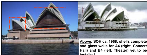
Figure 1: View from harbour showing glass walls A4 (right, Concert Hall) and B4 (left, Theater)
