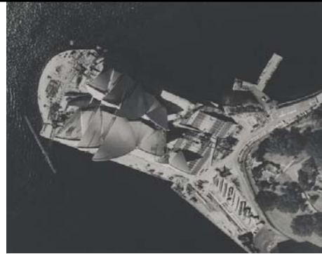
Aerial view of the SOH shells nearing completion (1967) 578
