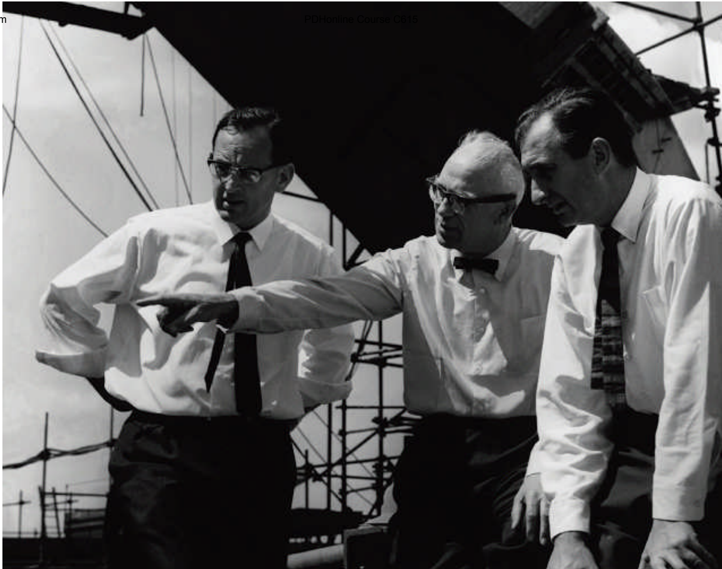
From left to right: Michael Lewis, Ove Arup and Jack Zunz. On-site during Stage Two construction.
