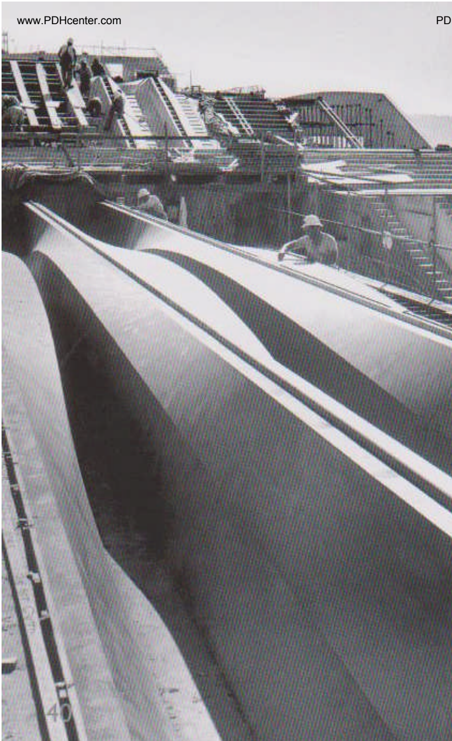
Left: resin-coated plywood forms for pre-cast concrete Concourse beams Above: forming the sculptural post-tensioned Concourse beams
