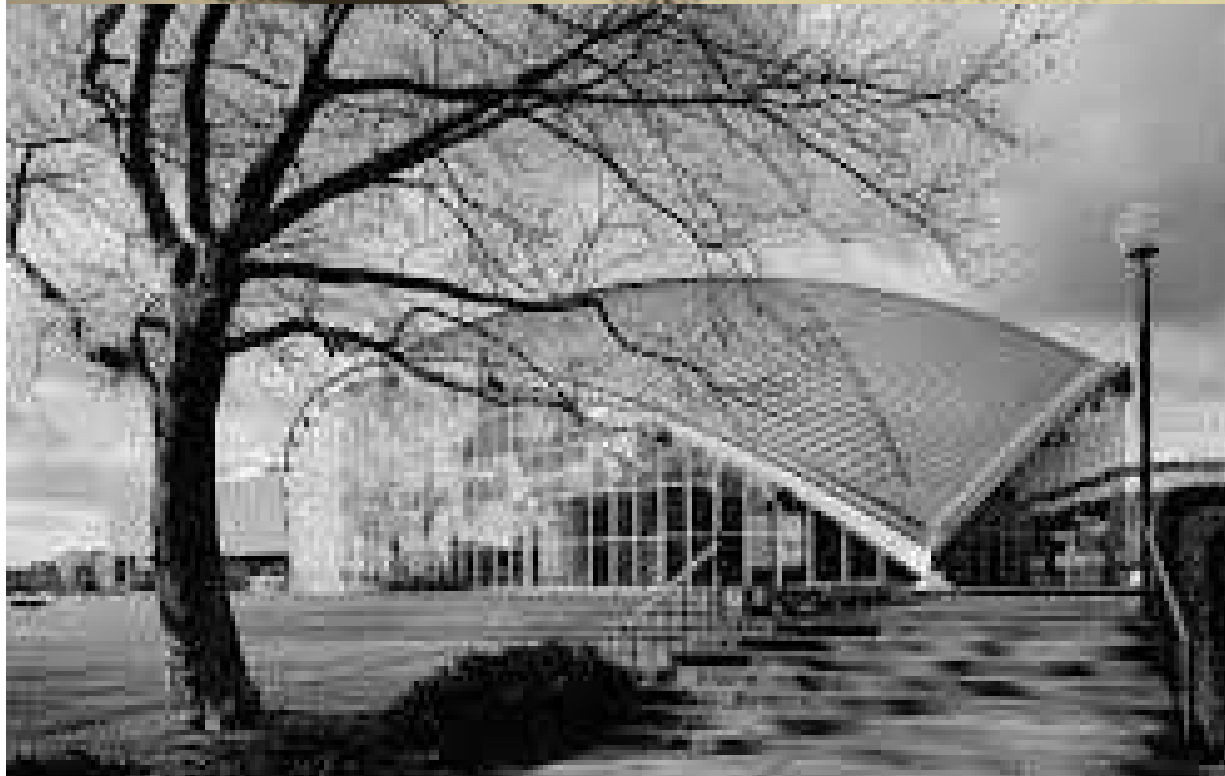
Left: Kresge Auditorium (MIT campus) by Eero Saarinen (1955) Above: cross-sectional view
