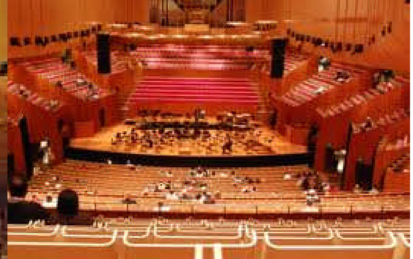
Concert Hall Interior views. The two performance halls (and other public spaces) are lined with panels made up of spaced Brush Box battens over a sound absorbing mat. 739
