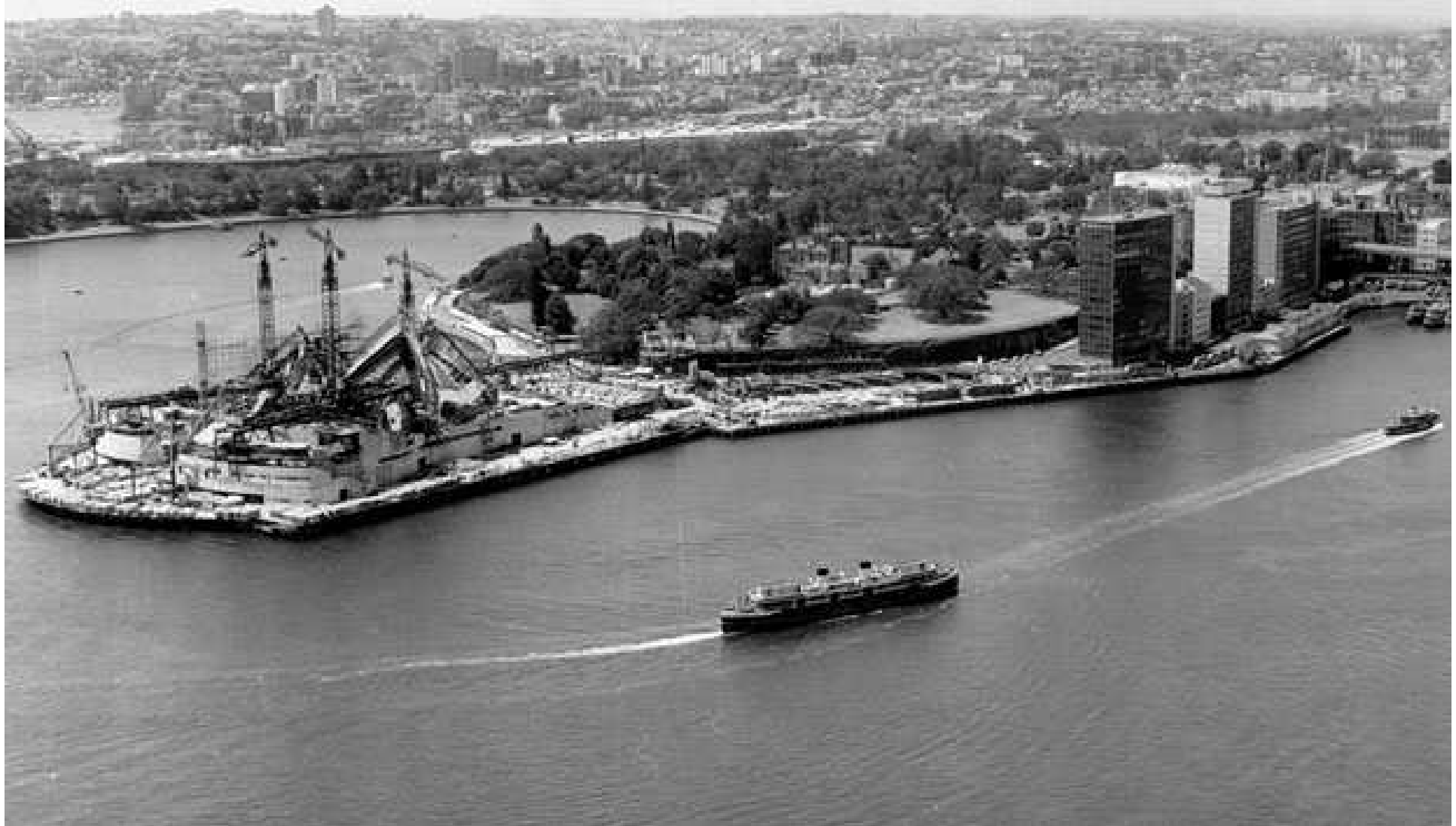
Aerial view of SOB under construction (December 1964)
