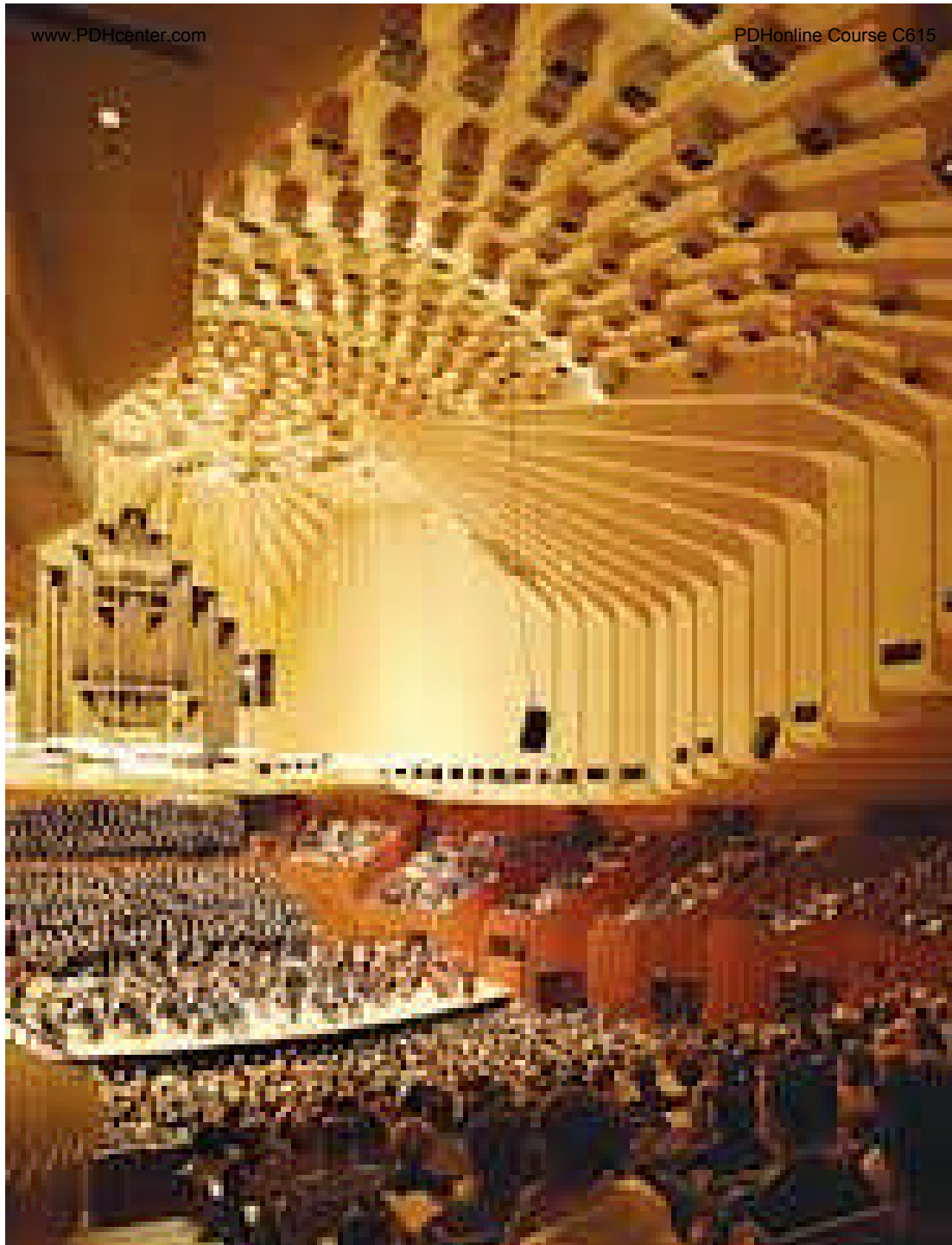
Concert Hall Interior views. The two performance halls (and other public spaces) are lined with panels made up of spaced Brush Box battens over a sound absorbing mat. 739
