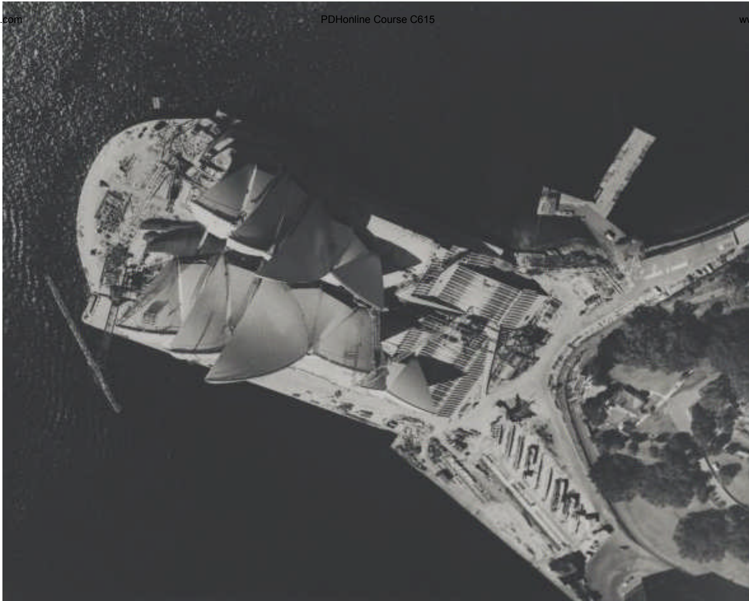
Aerial view of the SOH shells nearing completion (1967)
