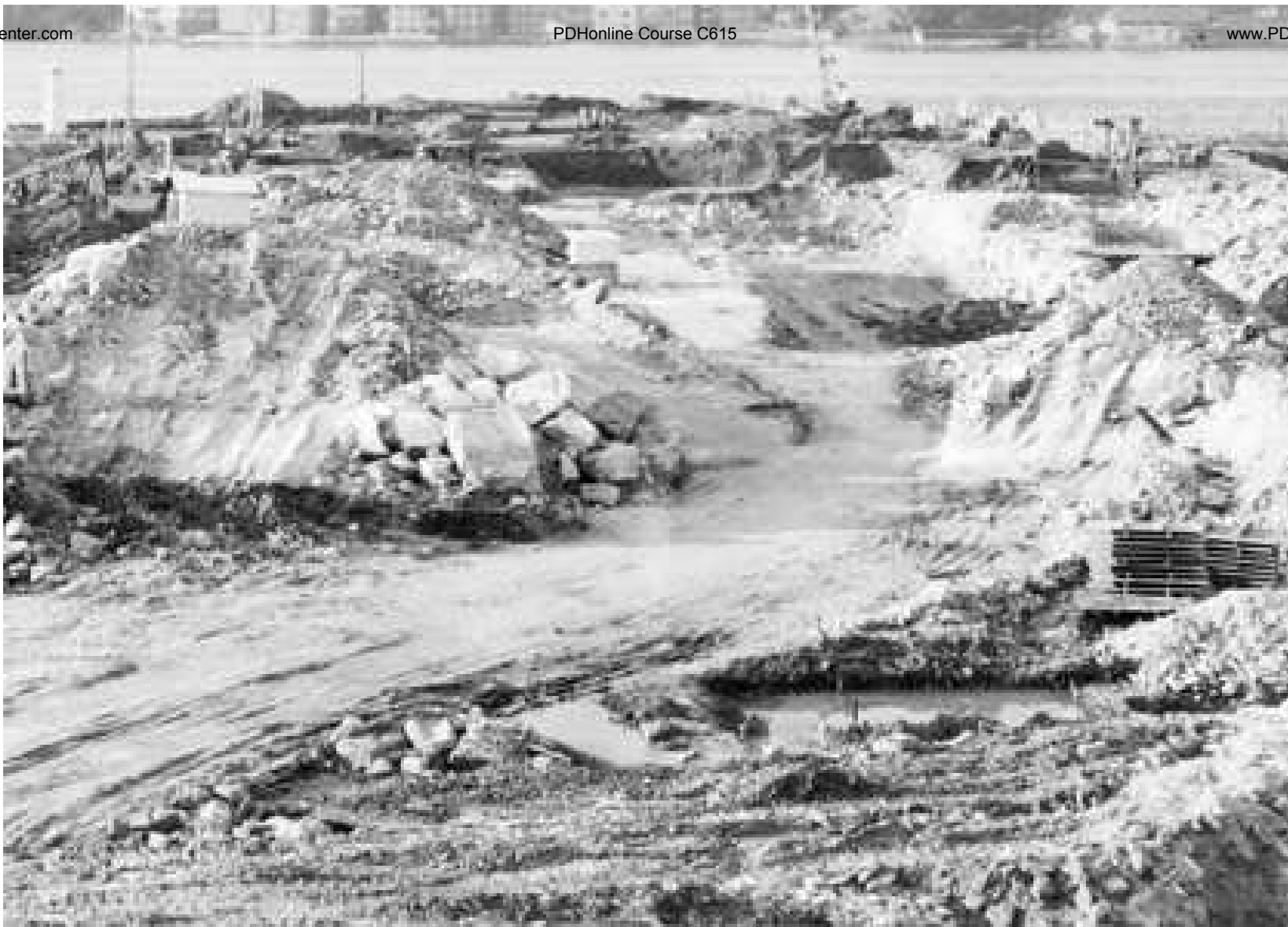
Excavation work commenced on Bennelong Point (Spring 1959)
