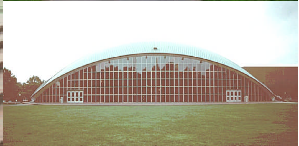
Kresge Auditorium, MIT Campus (1954). The dome-like roof (a concrete shell) is supported only on three points. Saarinen said it was “one-eighth of an orange.” The three “walls” are of glass.
