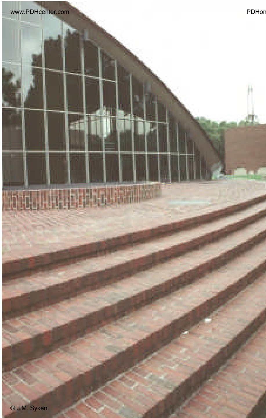
Kresge Auditorium, MIT Campus (1954). The dome-like roof (a concrete shell) is supported only on three points. Saarinen said it was “one-eighth of an orange.” The three “walls” are of glass.
