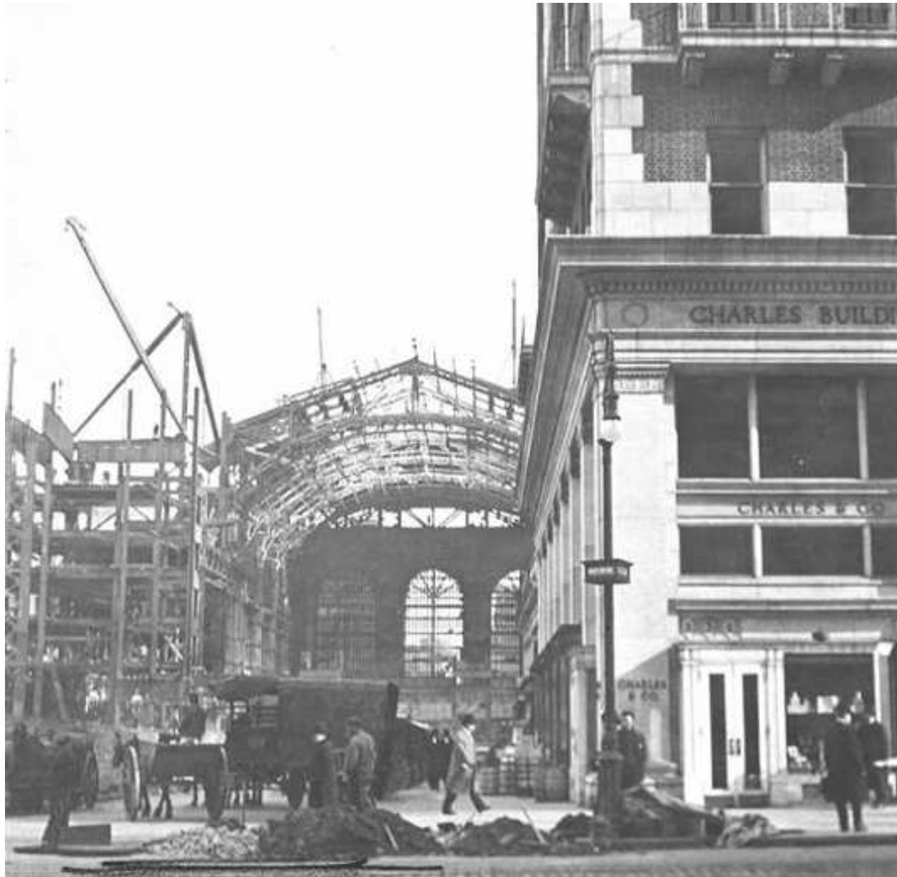
The steel framing support for the Main Concourses' vaulted ceiling in view (at center) in this photograph (ca. 1910)
