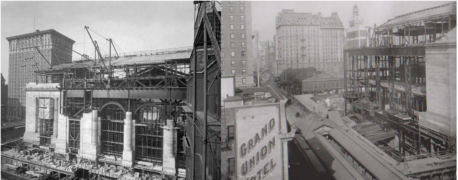
Top Left: steel framework complete and stone facade rising on the main ( 42nd Street ) elevation (January 1912)
