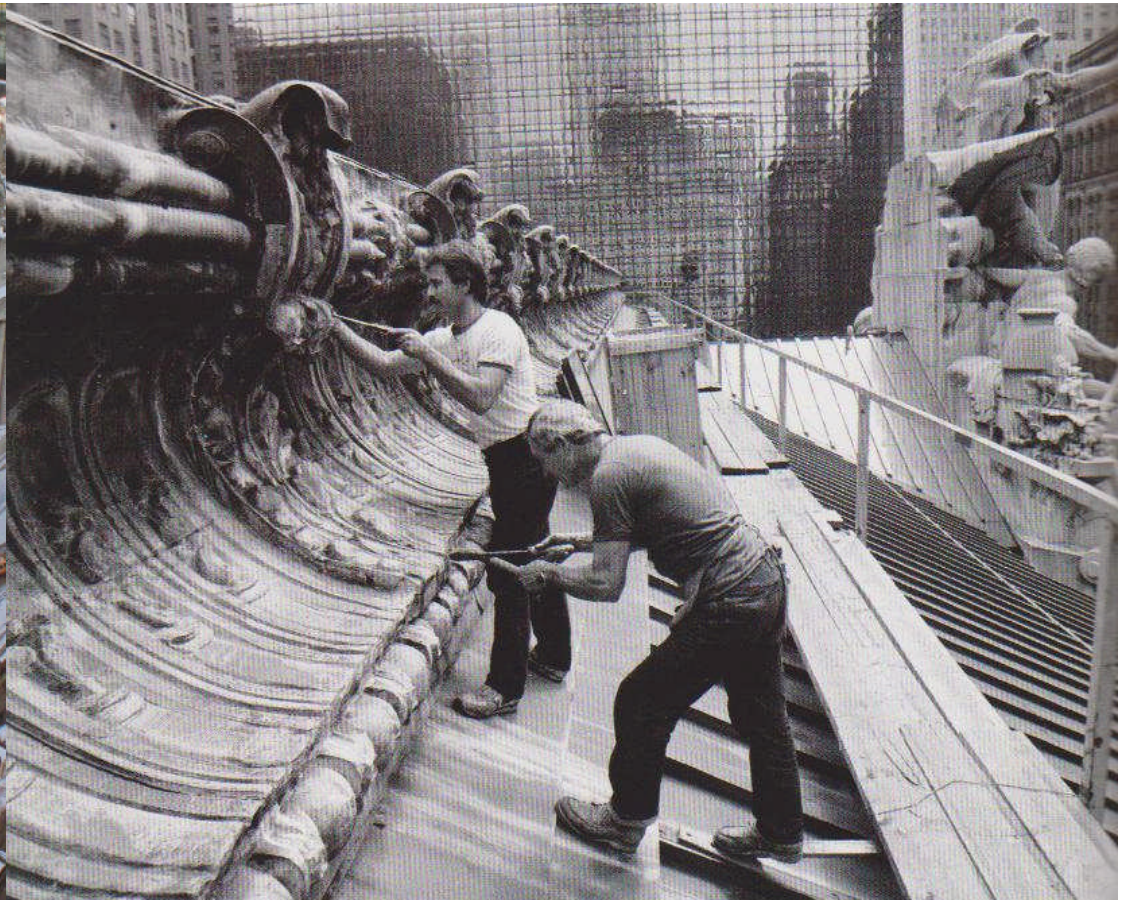
Above: $4.5 million roof repairs underway in 1987 (right). Before anything could be done to the interiors, GCT needed to be made weather-tight; it was no small/easy task. Due to expansion and contraction, metal fatigue had caused the copper plates (especially at the roof's fringes) to fray and fracture. A total of 55K square-foot of copper needed to be replaced. Eight-foot long copper panels were nailed to wooden strips spaced twenty-inches apart and the six-foot high frieze was repaired in-place. During WWII, eight twenty-four foot square skylights were "blacked-out". The black paint was peeled away or the glass pane/s replaced.
