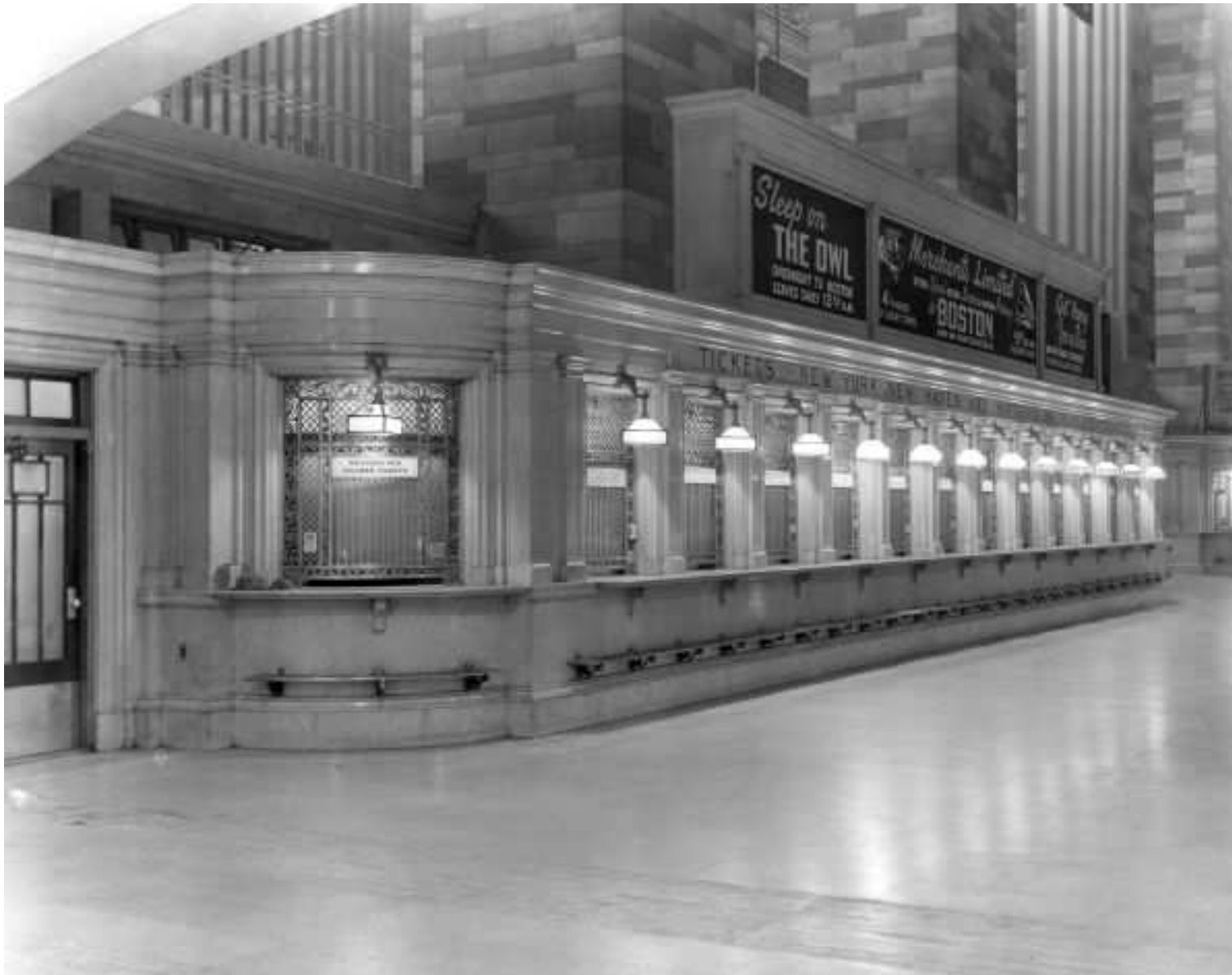
Above: Main Concourse ticket windows with original grills, rails and light fixtures (ca. 1913)
