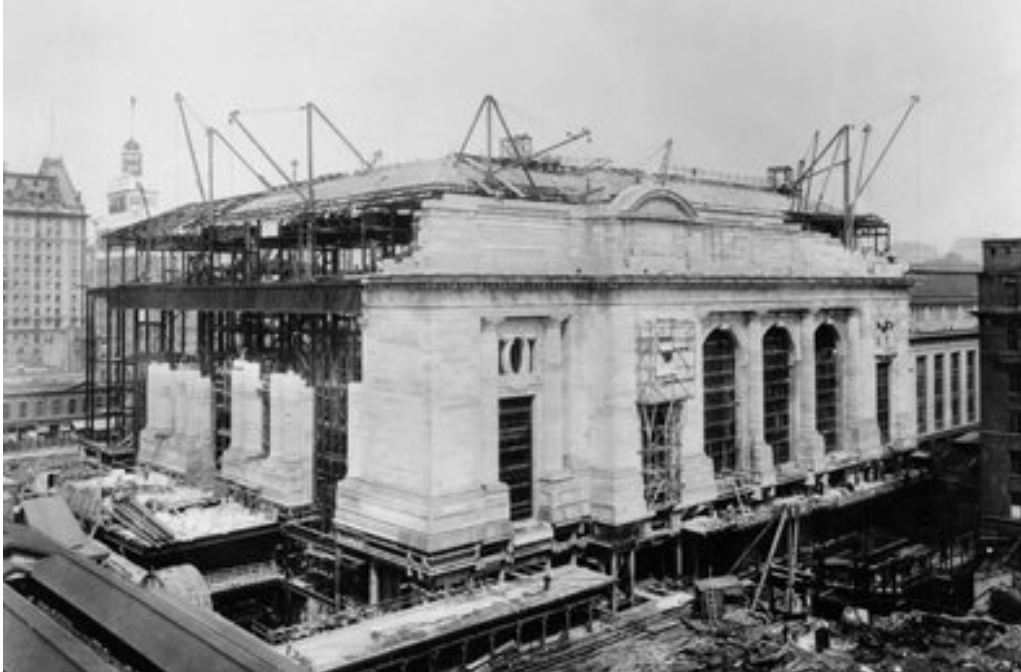
Top Left: steel framework complete and stone facade rising on the main ( 42nd Street ) elevation (January 1912)
