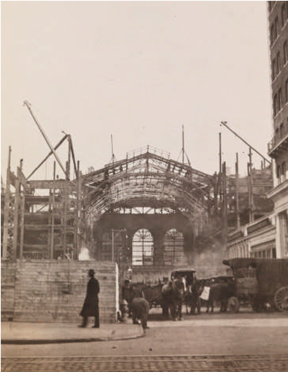
Above: view of the main (42 nd Street) facade looking north from Park Avenue . Note the derricks atop the multiple derricks atop the structure. Note the three “Portal” (arched) windows (April 1912) Left: construction of GCT (ca. 1911)
