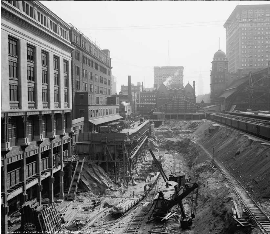
Top Left: excavation work (ca. 1908) Top right: Caption: “Looking south from 50th Street during the construction of Grand Central and the railroad yard in August 1909” Left: at left is the new Post Office and Railroad Office Building . Below are two levels of tracks that will be part of the completed terminal, which were already in service (1908)
