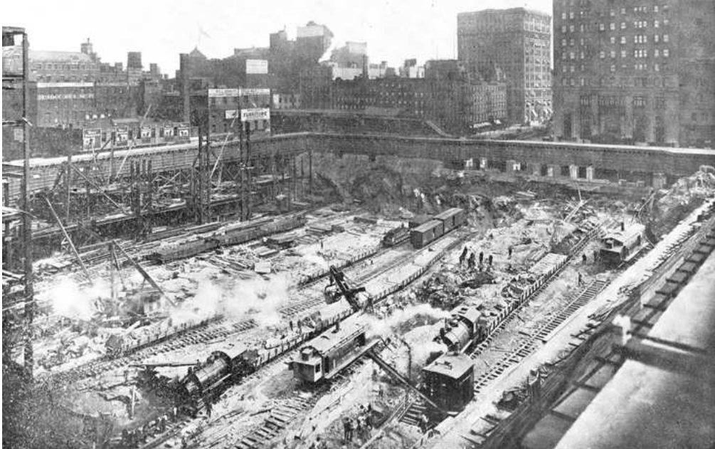
Above: Grand Central Terminal and Park Avenue under construction (ca. 1910)
