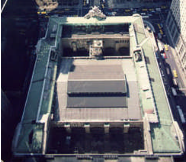
Above: $4.5 million roof repairs underway in 1987 (right). Before anything could be done to the interiors, GCT needed to be made weather-tight; it was no small/easy task. Due to expansion and contraction, metal fatigue had caused the copper plates (especially at the roof's fringes) to fray and fracture. A total of 55K square-foot of copper needed to be replaced. Eight-foot long copper panels were nailed to wooden strips spaced twenty-inches apart and the six-foot high frieze was repaired in-place. During WWII, eight twenty-four foot square skylights were "blacked-out". The black paint was peeled away or the glass pane/s replaced.
