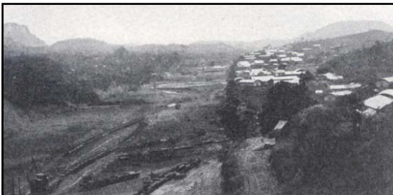
Above: northern end of excavation for proposed lock at Bas Obispo Left: hilltop at Bas Obispo torn up by dynamite. The French dump cars had a capacity from five to eight cubic yards.
