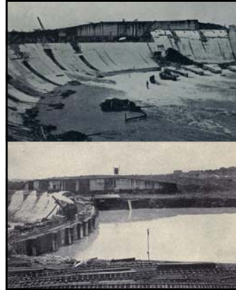
Top: caption: "Gatun Spillway looking South-West, showing downstream face of Ogee Dam, June 6, 1912"
