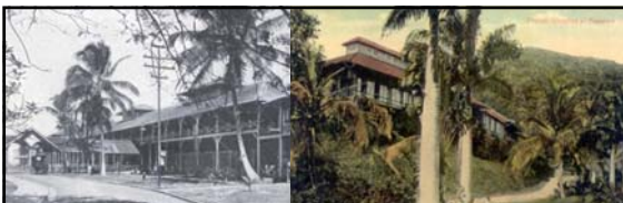
On the Isthmus, the Compagnie Universelle established medical services presided over by the Sisters of St. Vincent de Paul. The first 200-bed hospital was established in Colon in March 1882 (left). On the Pacific-side, construction for L'Hospital Central de Panama, the forerunner of Ancon Hospital, was begun on Ancon Hill (right). It was dedicated six months later, on September 17 th 1882. With the information on the mosquito connection in the transmission of Yellow Fever and Malaria not yet discovered, the French and the good sisters unwittingly committed a number of errors that were to cost dearly in human life and suffering. The hospital grounds were set out with many varieties of vegetables and flowers. To protect them from leaf-eating ants, waterways were constructed around flowerbeds. Inside the hospital itself, water pans were placed under bedposts to keep off insects. Both insect fighting methods provided excellent and convenient breeding sites for the Stegomyia Fasciata and Anopheles mosquitoes, carriers of Yellow Fever and Malaria. Many patients who came to the hospital for other reasons often fell ill with these diseases after their arrival. It got to the point where people avoided the hospital whenever possible.
