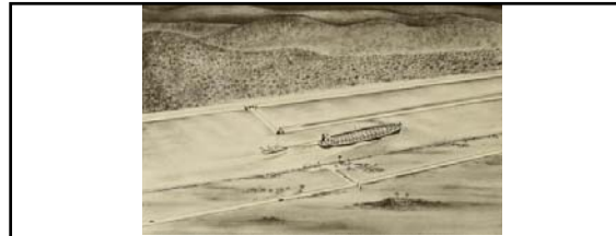
"...The uncertainty of safety of navigation under all tidal conditions led to consideration of a new concept: the installation of a tidal control structure at each end of a long restricted reach to limit the velocities of flow in a sea-level canal. It is contemplated that one structure and gate would be located close to the Pacific entrance and another 24 to 25 miles north thereof. The check gates would be moved alternately into position across or out of the channel at intervals of 6.2 hours or some multiple thereof when the Pacific is at the same level as the Atlantic. Under these conditions, the maximum velocity of flow would be approximately 2 knots at the Pacific entrance and less elsewhere. It is also contemplated that structures for gates would be built close to the Atlantic entrance where, if a gate were installed and employed alternately with the Pacific gate, the maximum velocity could be held to approximately 3 knots..." RE: excerpt from the Atlantic-Pacific Interoceanic Canal Study Commission report, 1970 794
