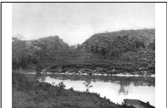
Above: caption: “View of the excavation at Bohio ”
