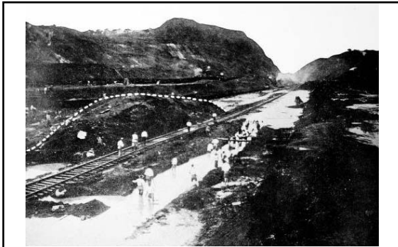
Above: caption: "An Eruption of the Canal Bed.' The pressure of the adjoining hills has forced up the soil at its weakest point, namely the bed of the Canal, to a height of 18 feet, as shown by the dotted line." 601
