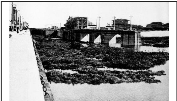
Above: caption: "Floating Islands in Gatun Lock Entrance. These islands, formed of aquatic plants with entwined roots and a little soil, must be towed away by tugs and sent over the spillway lest they block navigation."
