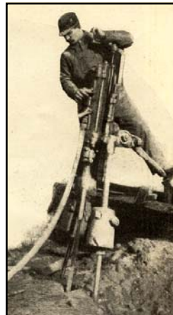
Left: caption: "A pneumatic drill at work - about a million cubic yards of rock will be excavated in building the tunnel. The rock of Manhattan Island is gneiss, pretty hard, but quite workable."
