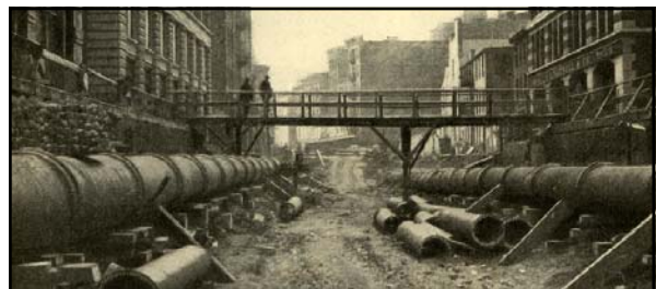
"...Having determined the route, the board's engineers, under the direction of their chief, William Barclay Parsons made a series of borings over the entire route to determine the precise nature of the ground in which the work was to be carried on. These borings went twenty-five feet below the surface, and they were only twenty feet apart - nearly six thousand of them altogether. Minute examinations of the city maps and records gave the exact location of every water pipe, gas main, sewer, pneumatic tube and wire conduit, every street car track, elevated railroad foundation, and building foundation that would be encountered on the route. The plan of the four track road, with stations a quarter of a mile apart, every sixth station being of double size to accommodate express traffic, was carefully worked out. It was determined that the four tracks should not be placed in pairs, one above the other, but that they should lie side by side in a broad, low tunnel. No motive power causing combustion in the tunnel should be used..."
