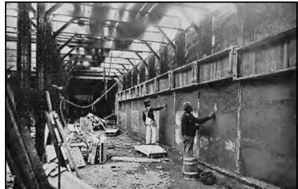
Above: caption: "Finishing Concrete Side-Arches of Subway"
