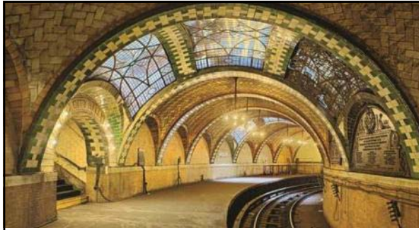
An example of the care used to obtain artistic effects can be seen clearly at City Hall station (above). The line at this point was through an arched tunnel. In order to secure consistency in treatment, the roof of the station was continued by a larger arch of special design.
