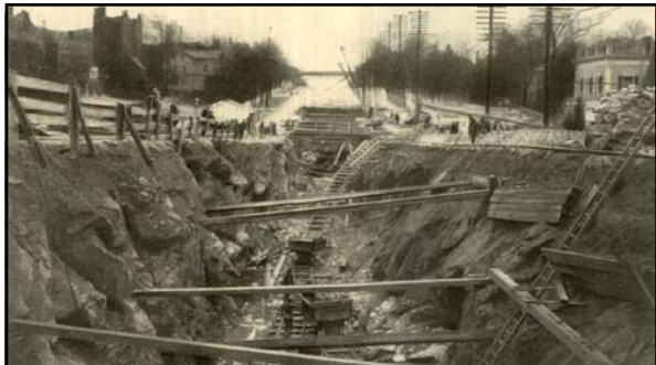
Above: caption: "View of the work on Broadway, looking south from One Hundred and Fifty Seventh Street, toward Trinity Church Cemetery. Both north and south of this point are hills through which a tunnel is being driven, the northern tunnel being nearly two miles long."
