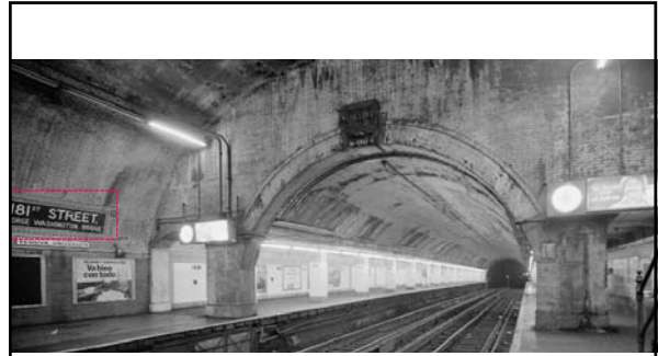
At the 168th Street , 181st Street (above) and at Mott Avenue station/s, where the Subway is deep beneath the surface, unadorned arches were built over the stations and tracks with spans of fifty-feet.
