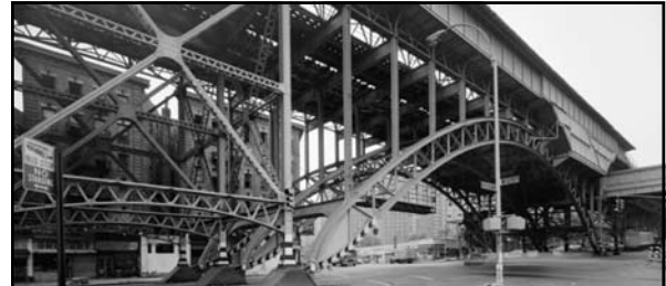
"...On April 16 the Carnegie Steel Co. took the contract to manufacture 74,326 tons of structural steel and about 4,000 tons of steel rails for this work...this contract requires the Carnegie Works to manufacture 22,439 tons of steel beams, 20,466 tons of riveted steelwork, 7,921 tons of steel columns, 23,500 tons of steel viaduct, and 4,064 tons of steel rails, or a total of 78,390 tons of finished steelwork. It has already been stated that this is the largest contract for steel ever undertaken by a single steel-maker for a single engineering work. It is as much steel as would be required to lay 556 miles of railway track with 80-lb. rails..." Engineering News and American Railway Journal, May 24 th 1900
