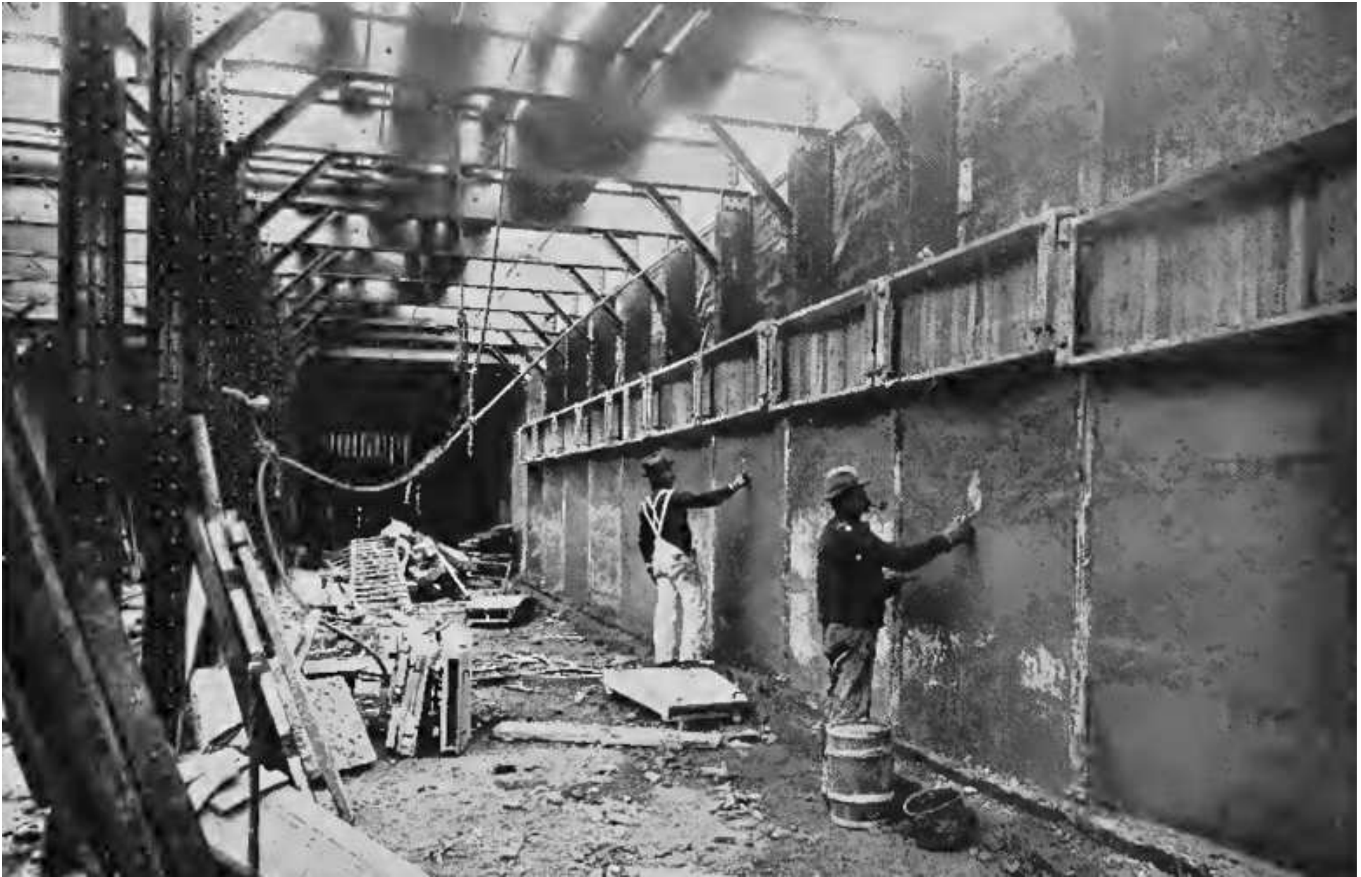
Above: caption: “Finishing Concrete Side-Arches of Subway”
