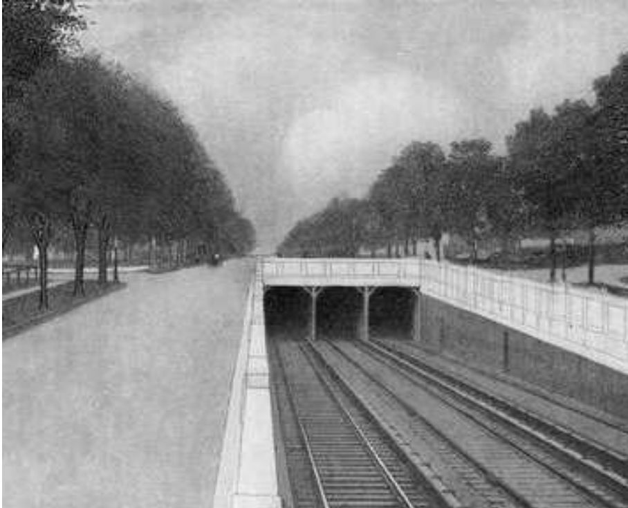
Top Left : southern masonry approach (view southwest from 123rd Street ) Top Right : tunnel approach (123rd Street) from viaduct (beyond) Left : Manhattan Valley Viaduct tunnel approach
