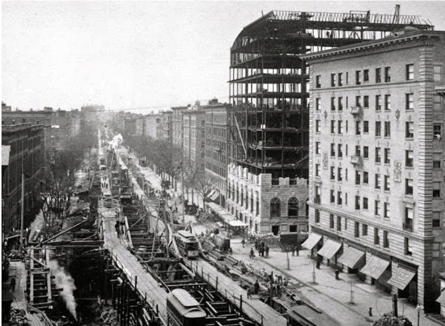
Top Left: caption: “Looking up Broadway from Trinity Church – showing working platform and gas mains temporarily supported overhead”
