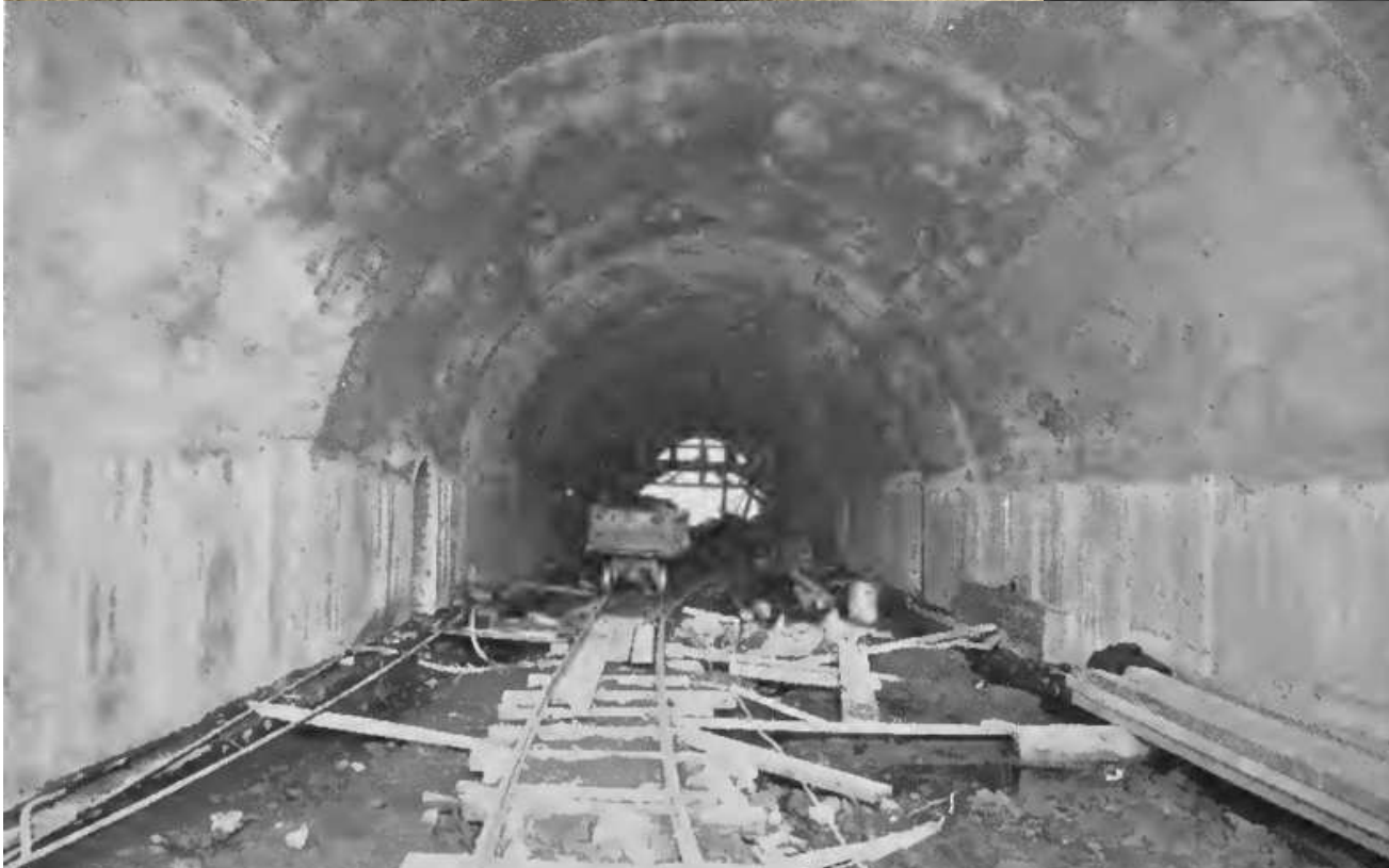
Top Left: caption: “Deep tunnel at Broadway and 156th Street”
