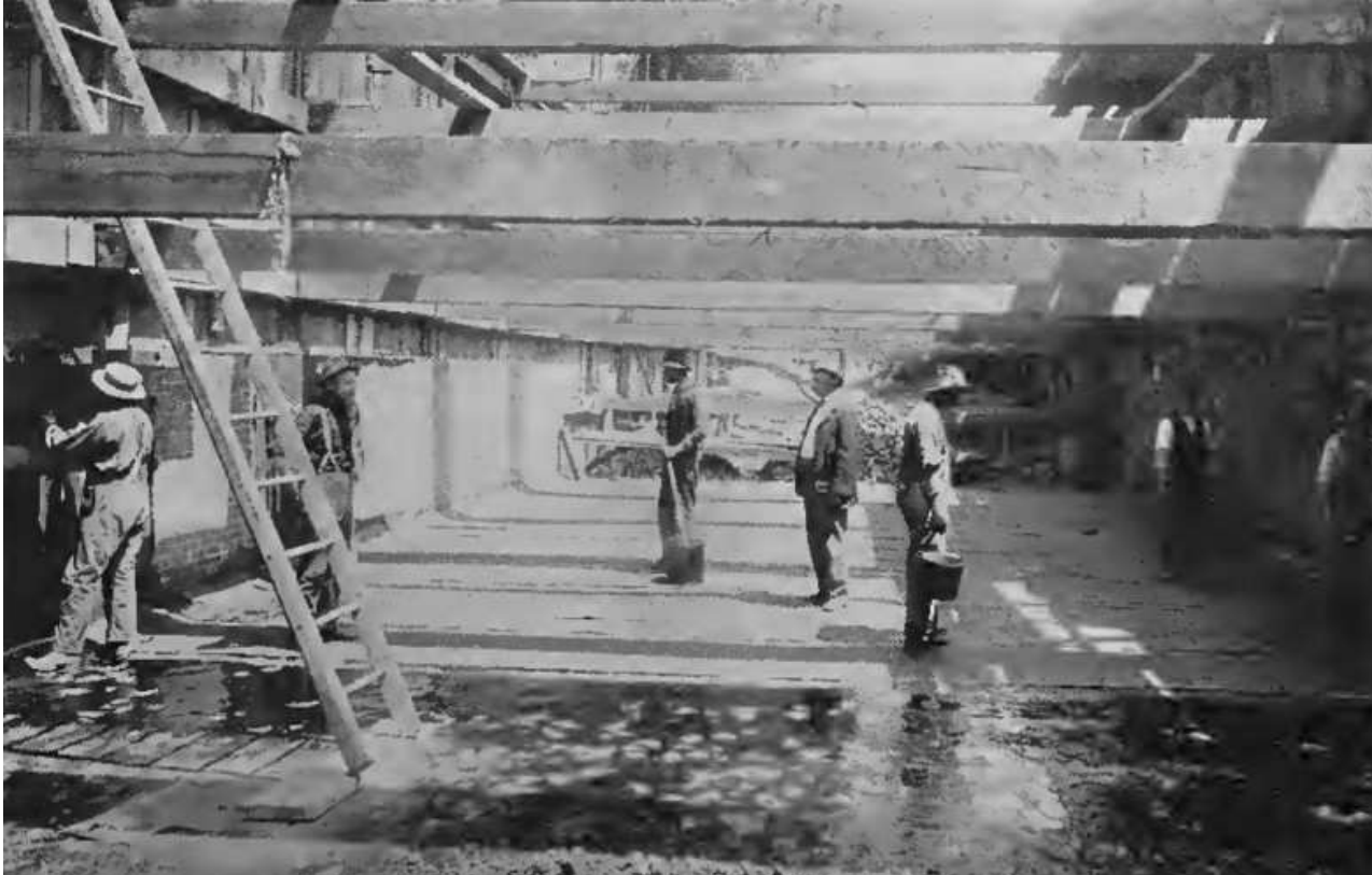
Top Left: caption: “Laying sheet waterproofing in bottom”
