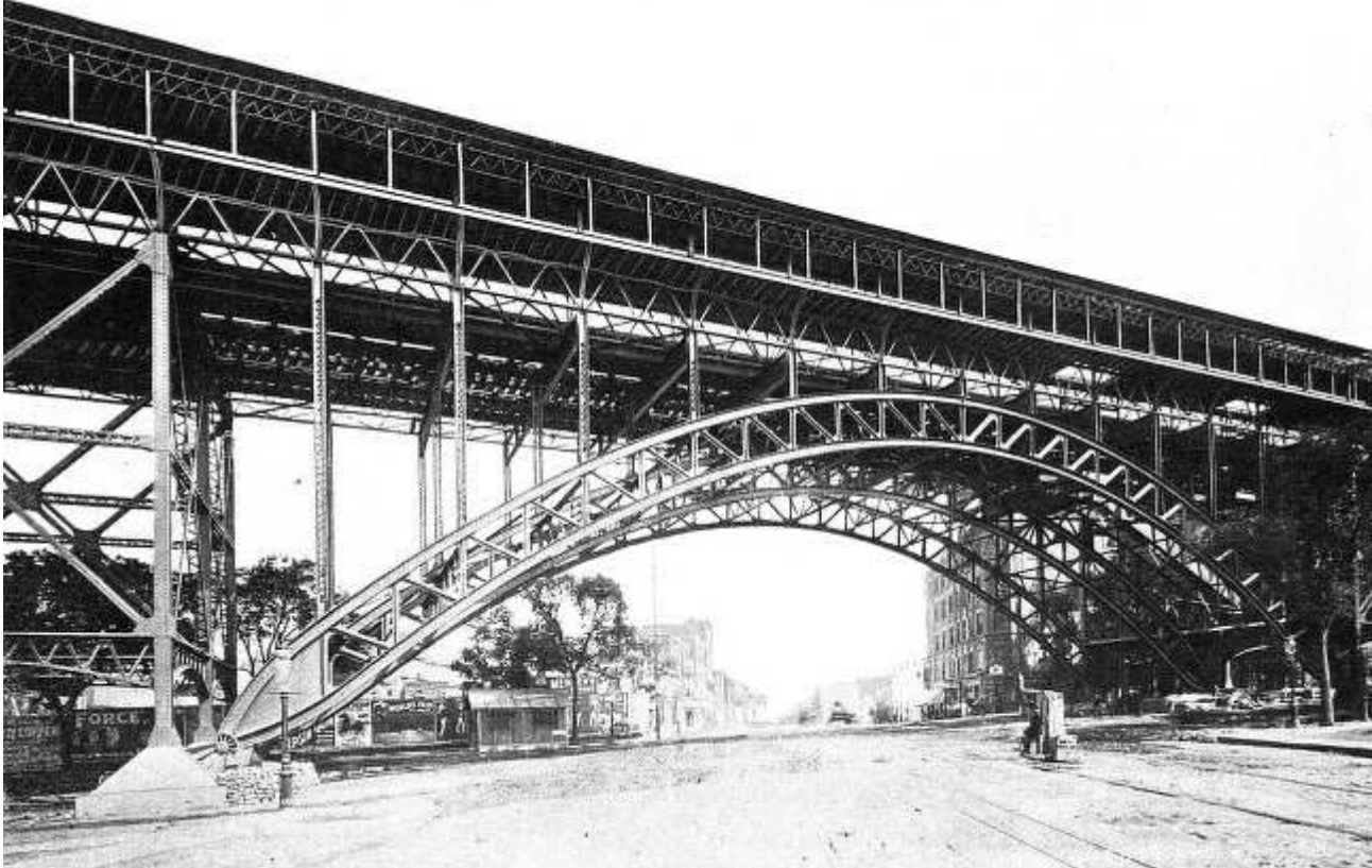
Top L&R: Westchester Avenue Viaduct Left: Manhattan Valley (Harlem) Viaduct
