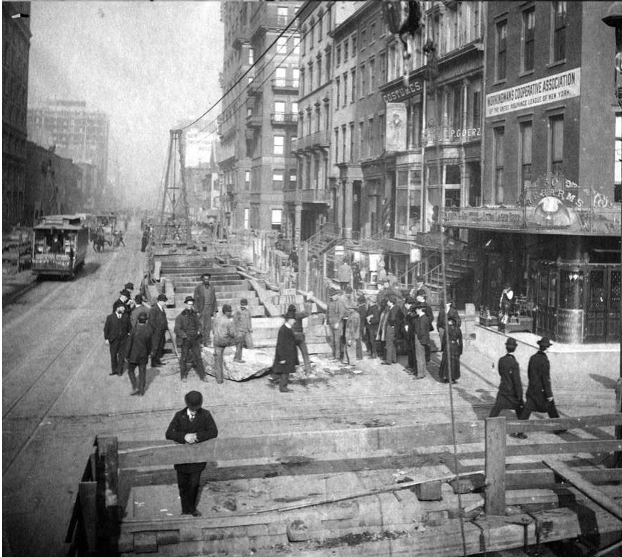
Top Left: caption: “Upper Broadway During Construction of Subway”
