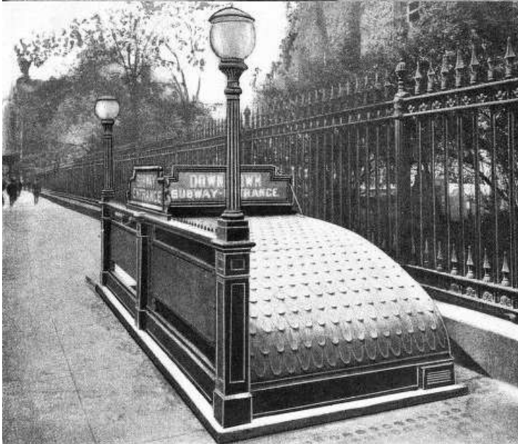
Top Left: exterior of IRT sub-station Top Right: interior of 23 rd Street IRT station Left: Fulton Street IRT entrance
