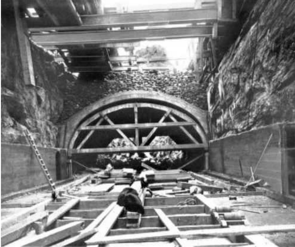
Top Left: caption: “Side drift looking from tunnel toward shaft”
