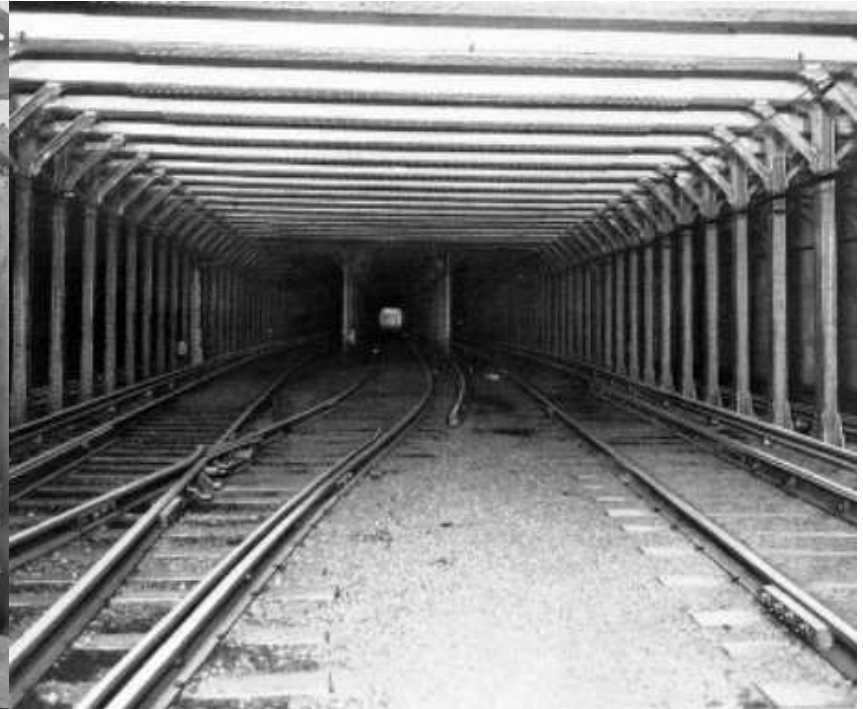
Top Left: caption: “Four-Track Steel Work in place between Reade and Duane Streets”
