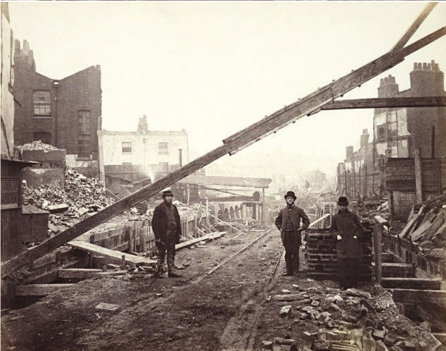
Top Left: caption: “Construction of the Metropolitan Railway, about 1861”
