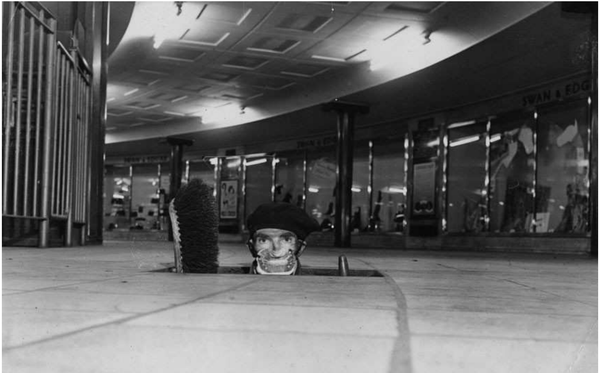
Above: Harry Weatheley, responsible for keeping the ventilator shafts clean, surfaces from a vent at Piccadilly Circus Underground station (ca. 1959) 260
