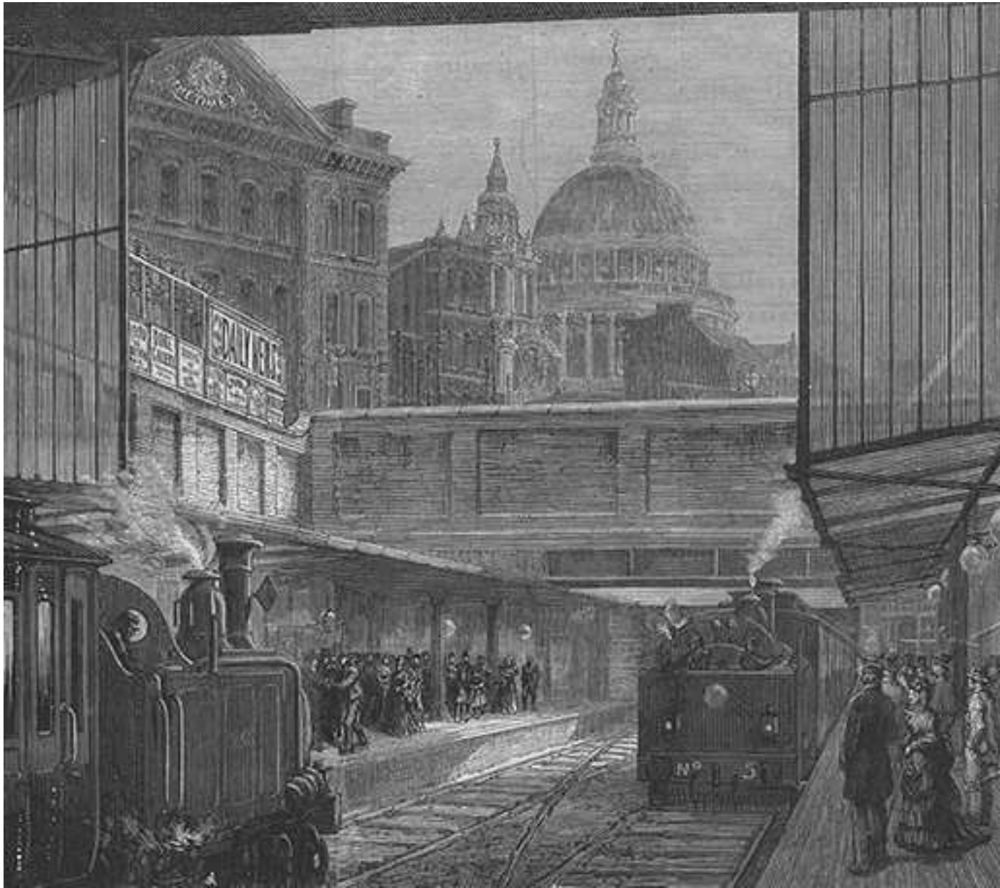
Above: Blackfriars Bridge Underground station (with St. Paul's Cathedral in the background)
