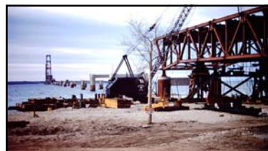
Top: caption: "Placing the first section of the bridge superstructure on the piers on the south side of the Mackinac Bridge"
