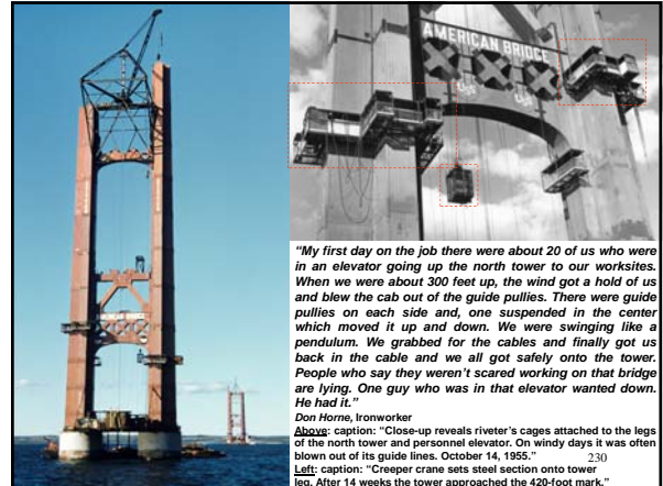
Left: caption: "Crepper crane sets steel section onto tower top. After 14 weeks the tower approached the 400-foot mark." 231
