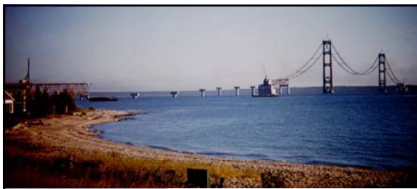
Above: caption: "Truss span construction starting out from Mackinaw City (south side)."
