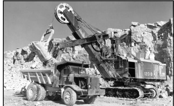
Above: caption: "The aggregates or crushed stone for the Mackinac Bridge foundations had to be specific sizes, hardness and cleanliness (actually washed two or three times to remove fine dust particles). It was quarried, crushed, screened and washed at Drummond Island, about 50 water miles away." 176
