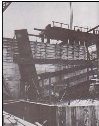
Left: caption: "The American Bridge Division of the U.S. Steel Corporation erecting the first steel in their $44,532,900 contract for the Mackinac Bridge superstructure. This first steel, consisting of anchor bars, is all buried in concrete."
