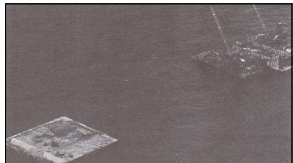
Above: caption: "An aerial view of the south anchorage, Pier 17, as it appeared in October, 1954; 85,000 tons of concrete and steel from the rock bottom of the Straits 90 feet below the surface to 10 feet above. To the right, foundation of Pier 18, caisson construction." 180
