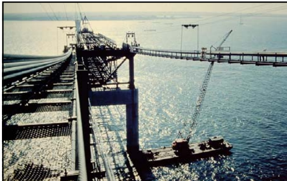
Above: caption: "Temporary catwalk with cable under construction." 291
