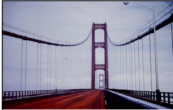
Above: caption: "The Mackinac Bridge roadway is complete"
