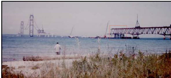
Left: caption: "Falsework had to be erected between distant piers to support the truss span until all the steel was 'hooked up,' connecting one permanent pier to the next."
