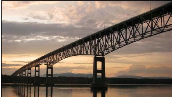
The Kingston-Rhinecliff Bridge (a.k.a. George Clinton Memorial Bridge) is a continuous under-deck truss bridge that carries NY 199 across the Hudson River in New York State (north of the city of Kingston and the hamlet of Rhinecliff). Though not complete, it was opened to traffic on February 2 nd 1957 as a two-lane (one in each direction) bridge. The formal opening was held on May 11 th 1957.
