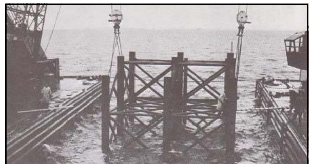
Above: caption: "With the caisson guide (one side of the corral) resting on the bottom, workmen unhitch the block and tackle connected to the derricks which lowered the huge clumsy framework precisely into position."
