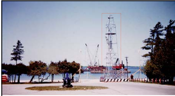
Above: construction of the Mackinac Bridge officially began on May 7 th 1954 at what was the parking lot for Michilimackinac State Park. The metal structure (highlighted) was one of seven land-based survey towers at fixed locations which were used along with six water-based towers. By sighting along lines from one location to another and by directing surveyors in boats to position themselves where these lines crossed, the location/s of piers was thus determined precisely.
