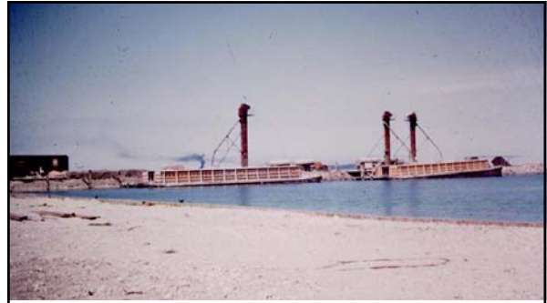
Above: caption: "Barges used for floating superstructure truss panels into position." 164
