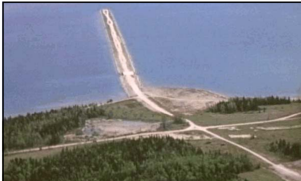
Above: a causeway 4,200-feet long was built from 1939 to 1941 in anticipation of a bridge across the Straits that was delayed due to the outbreak of WWII. Steinman used the existing causeway in his plans for the new bridge realizing a savings of $3 million in construction costs.
