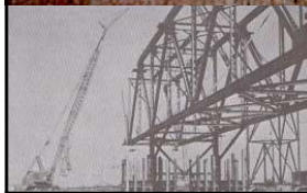
Left: caption: "Falsework had to be erected between distant piers to support the truss span until all the steel was 'hooked up,' connecting one permanent pier to the next."
