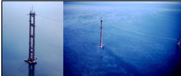
Left: caption: "Catwalk spanning over the 762-foot tall tower; 210-feet below the water line and 552-feet above." Right: caption: " Catwalk spanning between tower, left, and cable-bent, right."
