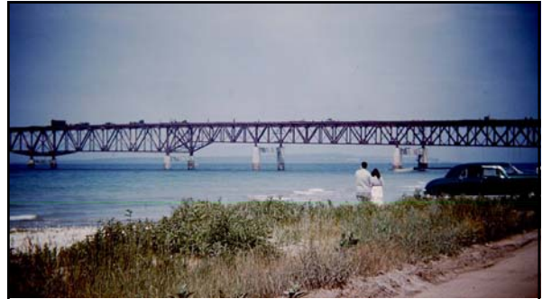
Above: caption: "Hundreds of visitors watched and photographed the Mackinac Bridge construction each day."
