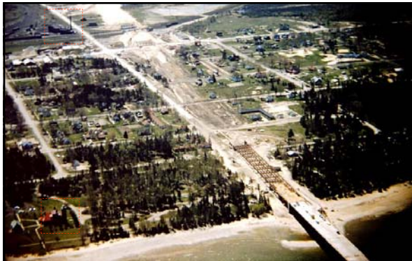
Above: caption: "Construction of the south approach to the Mackinac Bridge. Old Mackinac Point Lighthouse can be seen at the lower left and the Michigan Central Railroad roundhouse with the tall smokestack at the upper left."
