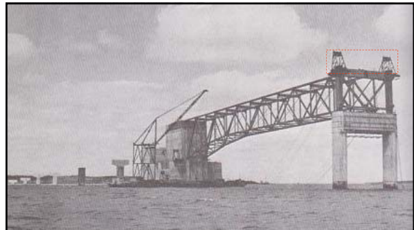
Above: caption: "In order to spin the cable there had to be a catwalk (a.k.a. "Footbridge") on which the cable spinners could work. In order to build a catwalk there had to be wire ropes to support it, five for each catwalk, raised from one anchor block over the tower tops to the other anchor block following the same curve and contour that the cables would eventually take. Here the wire ropes were started from the anchorage to the cable-bent (Piers 21 and 22)."
