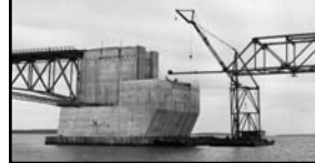
Above: caption: "At the outset of 1957 construction season the previous year's unfinished work was completed when the truss spans were carried all the way to the anchor blocks, thus completing a steel structure across the Straits."
