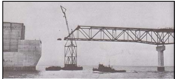
Above: caption: "At the outset of 1957 construction season the previous year's unfinished work was completed when the truss spans were carried all the way to the anchor blocks, thus completing a steel structure across the Straits."
