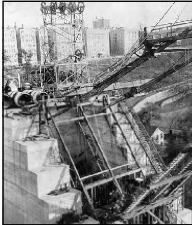
Left: caption: "Wire reels, unreeling machines, tension counterweight tower and stiffleg derrick on New York south anchorage block. Footbridge cables and their anchorage eyebars in foreground, Strand anchorage eyebars under footbridge cables. Inclined spinning frame and adjustable spinning platform over anchor pit."
