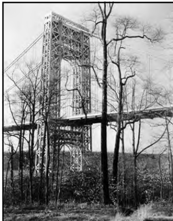
“Based on comparison and on the theories we find in textbooks and other treatises on suspension bridges, we should expect the stiffening system of the George Washington Bridge to weigh from 13,000 to 14,000 pounds per foot and be eleven stories high. Actually, it weighs only 1,100 pounds per foot in the initial stage with only one deck for highway traffic and will weigh 2,350 in the final stage with two decks.”
