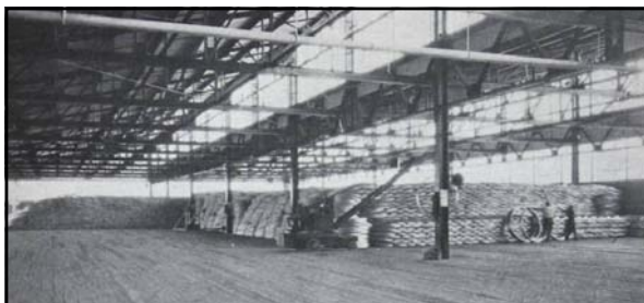
"...The coils of galvanized cable wire for the Hudson River Bridge are delivered by electric crane trucks to a great storage warehouse, where thousands of tons are piled awaiting reeling and shipment. Each coil bears a metal tag giving the heat and other numbers by which its test record can be identified, and its records traced back through the rods, billets, blooms and ingots, to the raw products charged into the acid open hearth furnace..." John A. Roebing's Sons Co.
