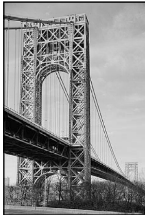
"...As first inaugurated, the bridge thus took the form of a simple suspension structure, designed on a tremendous scale. The building of the lower deck, with its four railway tracks, involved the addition of two stiffening members set 106 feet apart and having a depth of 29 feet..." Wonders of World Engineering, November 1937 Left: caption: "New York Tower, looking West"
