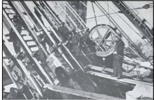
Above: caption: "Removing wire loop from wheel momentarily stopped for reversal at anchorage. Note permanent strand shoe and strand connected to strand arm in spinning position at lower left corner."
