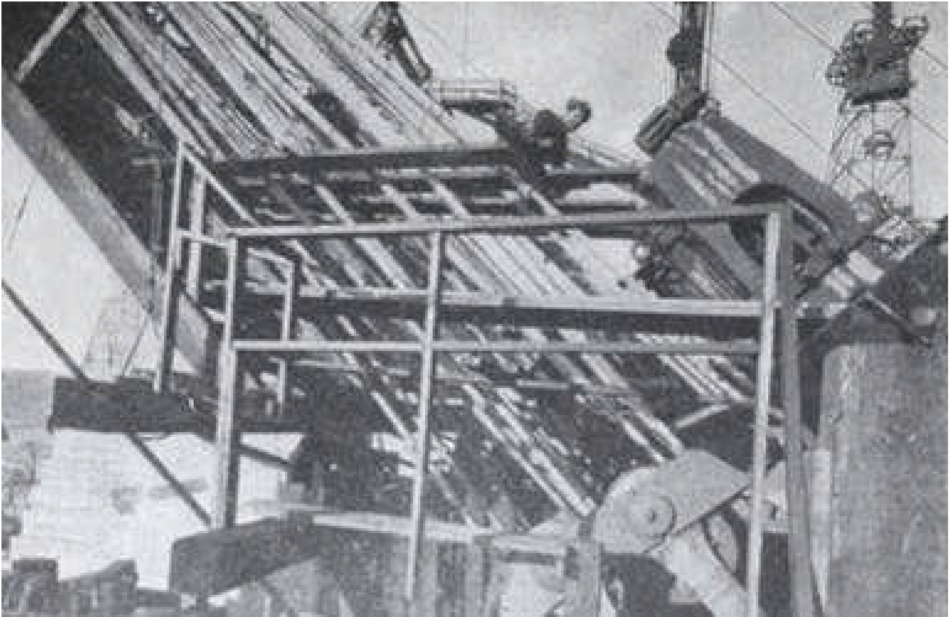
Above: caption: “Lower tiers of strands connected to eyebars in New York anchorage, and working platforms prepared for spinning higher and higher 337 tiers of strands”
