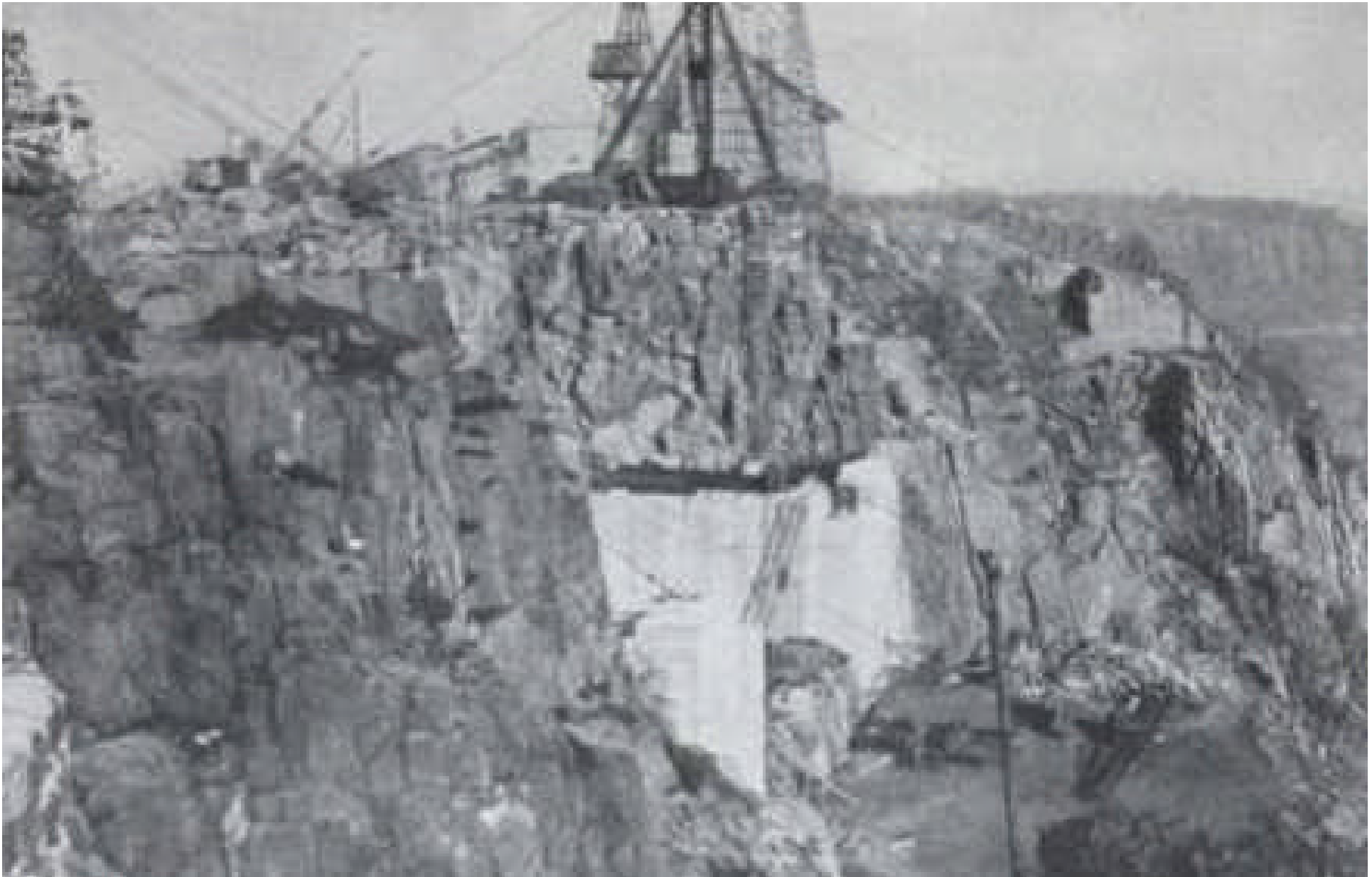
Above: caption: “Upper end of hoisting cableway on New Jersey shore, derrick mounted alongside of approach cut, commanding anchor block in cut”
