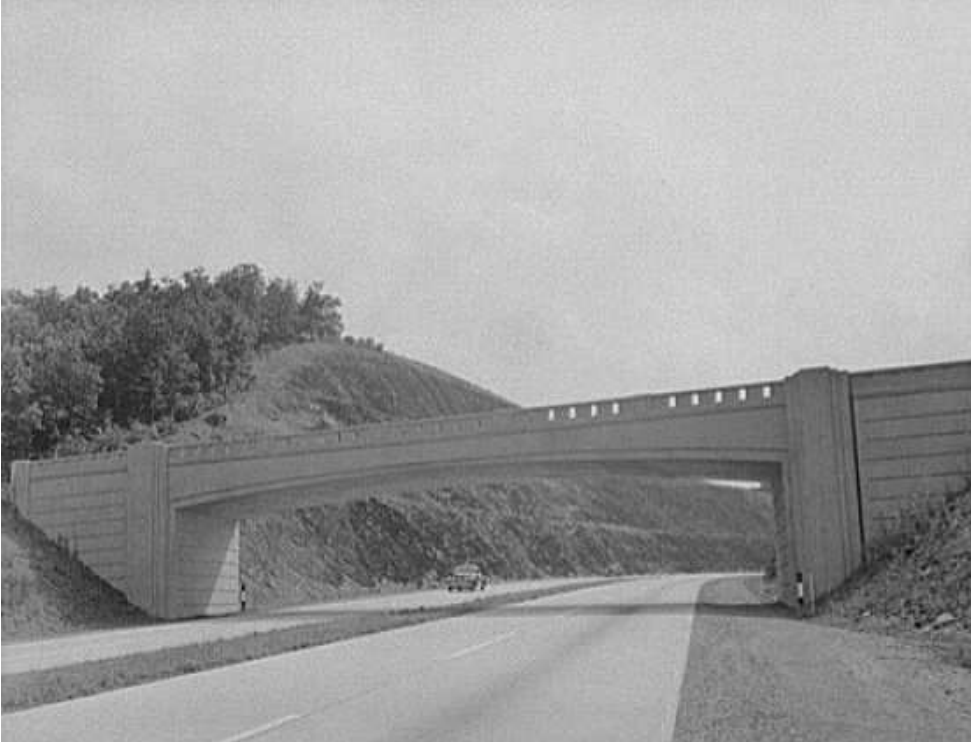
Above & Left: typical PA Turnpike overpasses
