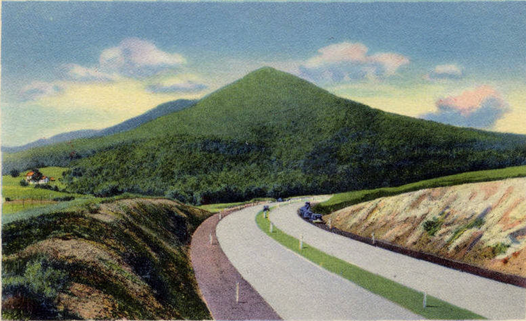
Pyramid Point on Pennsylvania Turnpike, East of Fort Littleton, Pa.
