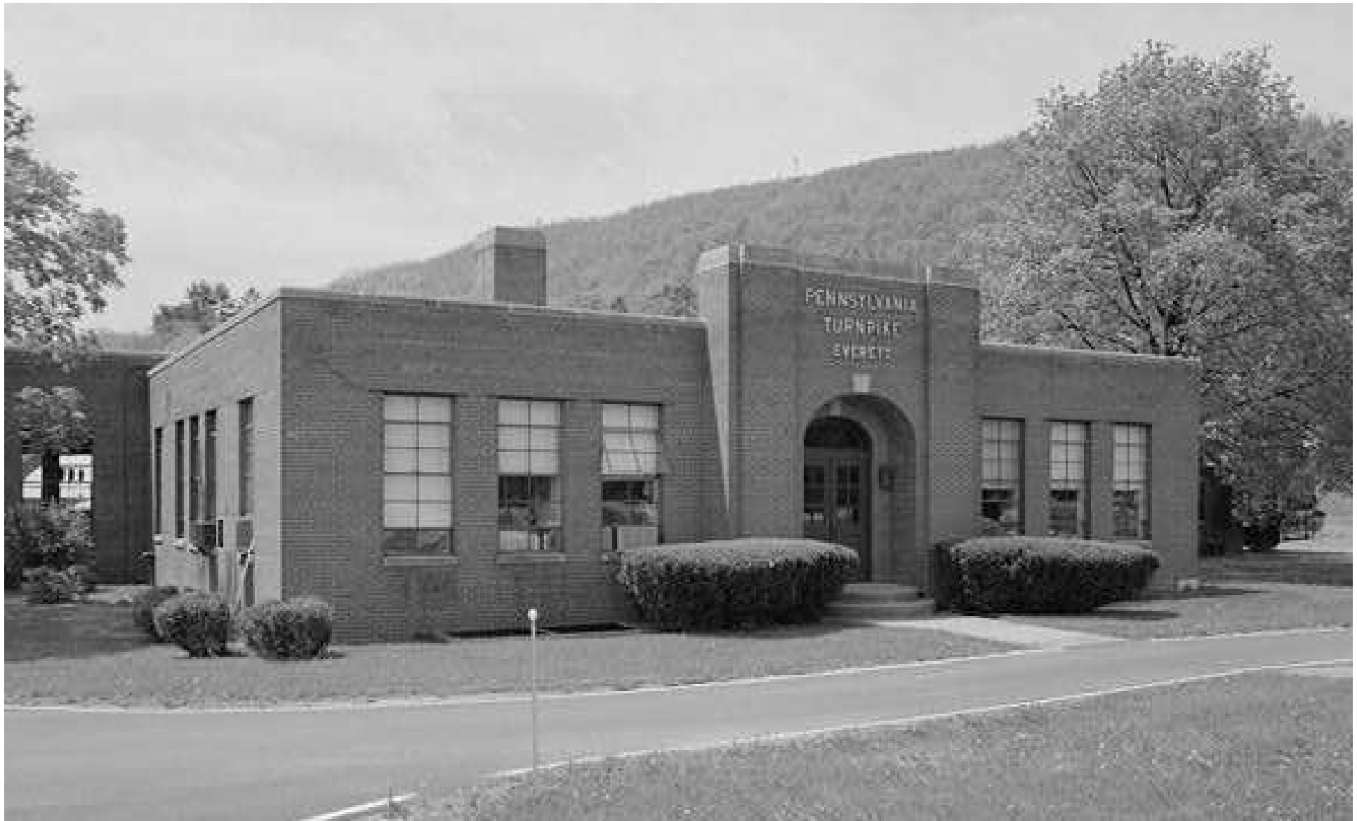
Above: caption: “Pennsylvania Turnpike, Everett Headquarters, North side of State Route 1004 near intersection with Township Route 503, Everett, Bedford County, PA – General View of Headquarters Building, Looking West” 122
