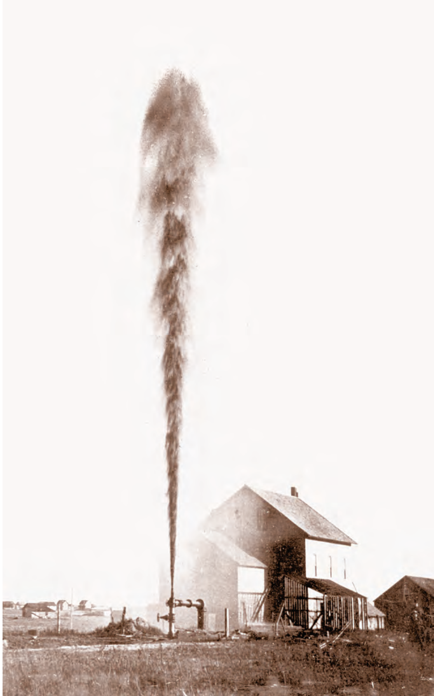
Artesian well at Woonsocket, well throws a 3-inch-wide stream to height of 97 feet, Sanborn County, South Dakota, Circa 1900 (Darton, N.H., 1905, Plate 60-B).
