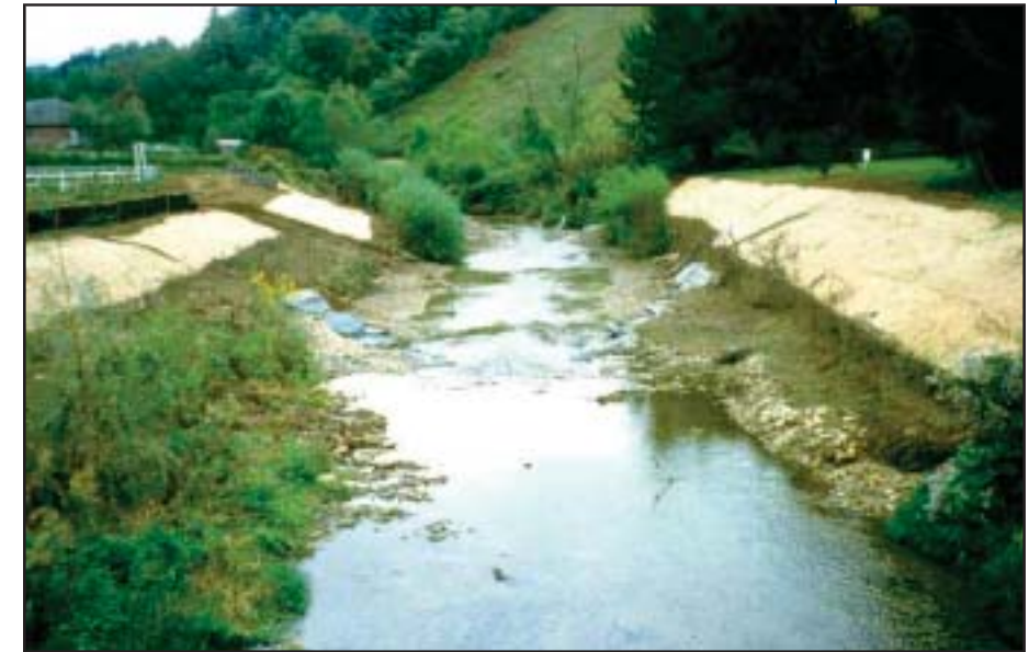
Figure 11.6 Cove Creek after restoration
