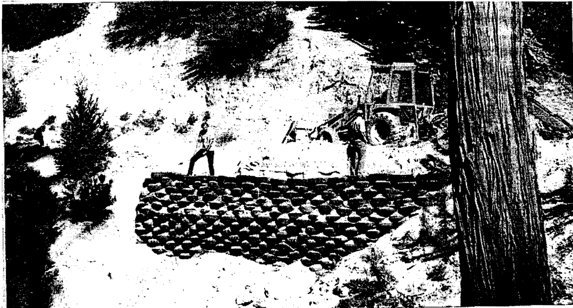
Figure 2.4. A Tire-faced Wall in California (7)
