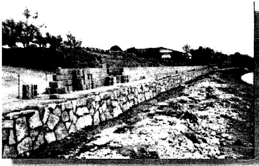
Figure 2.22: Block Retaining Wall on Top of Bales (12)
