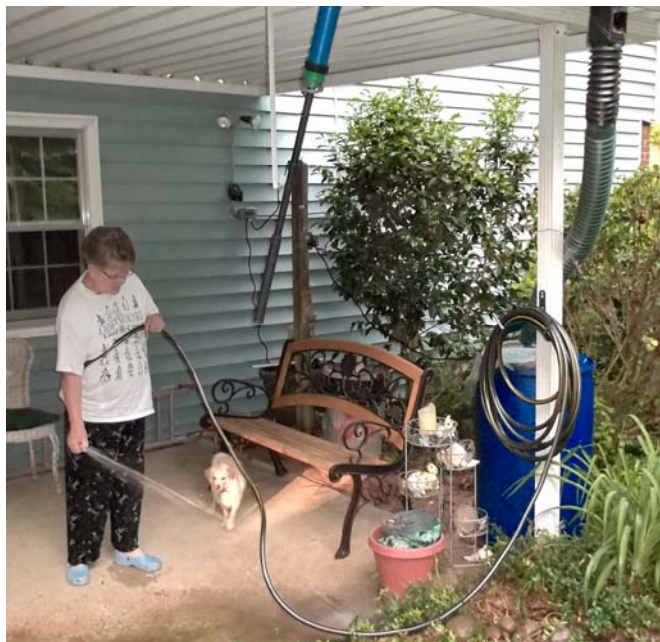
Shows the power of the pump spraying water Sump pump provides good pressure, requires 5/8" hose
