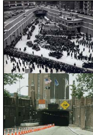
Top: caption: "Opening ceremonies Lincoln Tunnel, New York entrance, December 21, 1937" Bottom: caption: "Photo shows the Art Deco-style Manhattan portal of the Lincoln Tunnel and the east ventilation tower"
