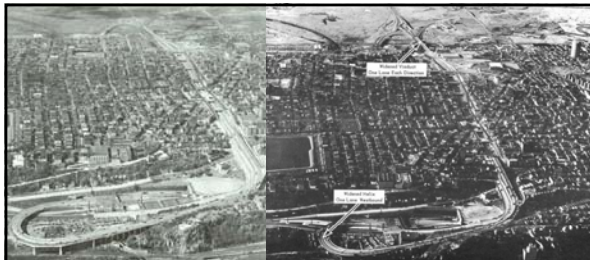
Left: caption: "New Jersey Approaches prior to start of construction of the Third Tube Project" Right: caption: "New Jersey Approaches after completion of the Third Tube Project"
