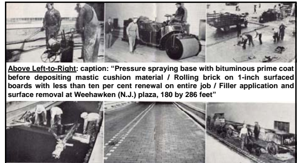
Above Left-to-Right: caption: "Striking off asphaltic-sand mastic bed course with screed traveling on rollers and discs with compensating carriage / Close-up view of completed brick pavement showing clean wire-cut skid-resistant traffic surface / Kerosene fueled heating kettles in which 'blended' asphalt filler was heated to 450-degrees F"
