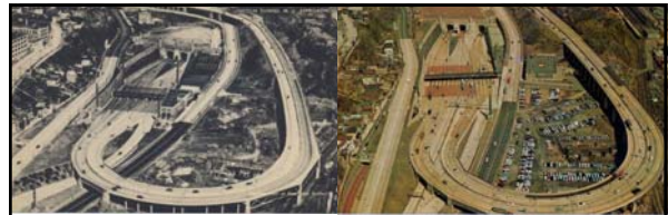
In 1952, the PA and the New Jersey Turnpike Authority (NJTA) extended the Lincoln Tunnel western approach for 0.9 mile west to EXIT 16 of the recently opened New Jersey Turnpike in Secaucus . The extension provided for grade-separated interchanges for US 1/9 and NJ 3 , as well as for a toll plaza. The Lincoln Tunnel Approach became part of the Interstate highway system in 1956. In 1971, the Mid-Manhattan Ex-pressway that was to connect the two I-495 sections in New Jersey and New York (the Lincoln Tunnel Approach and the Long Island Expressway ) was canceled. It was not until 1989 that the Lincoln Tunnel Approach was re-designated NJ 495 .
