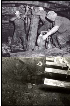
"...Thanks to this device and to a host of other, if less spectacular, refinements in mechanical technique – including an improved type of erector arm to lift the heavy segments into place, and high-speed muck conveyors that disposed of the river-bed ooze through which the tunnel was pushed – its construction is expected to set a speed record for undertakings of its type. Its scheduled opening date of January 1, 1938, may be materially advanced..." Popular Science, March 1936 Top: caption: "Sandhogs place locking ring segment in place to complete a ring prior to making another push of the shield. Note the erector arm in the center of the photo." Bottom: caption: "Removing muck from tunnel with shovel operated by compressed-air" 145
