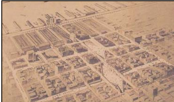
Above: caption: "Ultimate Arrangement of New York Approach. How the plazas and approaches for both tubes of Lincoln Tunnel, as well as plazas of the proposed Crosstown City Tunnel, will appear when completed. The new approaches (named Dyer Avenue and Galvin Avenue in memory of former Chairmen of the Port of New York Authority) extend from West 34th Street to West 42nd Street, midway between existing avenues. They are planned for use of tunnel traffic exclusively." (as of December 1937) 127
