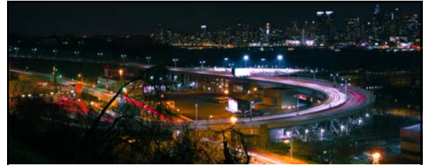
Above: caption: "That great curving ramp, called a helix by the engineers who built it, leads down into three of the world's most expensive holes in the ground: The triple-tube Lincoln Tunnel from New Jersey to New York City. Eighteen traffic lanes pass under the toll booths on the plaza at lower left, and they merge into six as they enter the tunnel. Beyond the Hudson River, the lights of the metropolis glamorize the night. The tallest building (upper left) is the Empire State. Each day, nearly 40,000 automobiles go underground here at Weehawken, N.J. and emerge after a five minute trip on the west side of Manhattan between 38th and 39th Streets. And an equal number escape the jammed streets of the crowded island and sweep back up the helix. The impatient drivers take little note of the design which their headlights emphasize, but they are part of an accidental pattern of beauty. And even these weary travelers must find subconscious satisfaction in traversing this mighty spiral, upward and outward from deep beneath the river." Saturday Evening Post, September 1958
